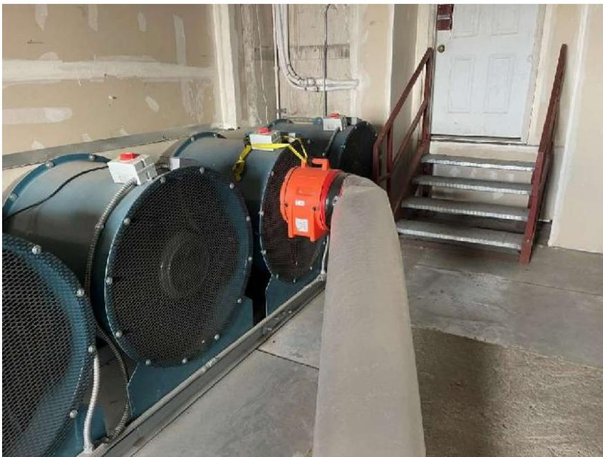
Our system, if implemented, would involve covering the end of the duct fan with visqueen (see the highlighted area in previous photo) and cutting an appropriately sized hole to match the intake of the ramfan to better control the air coming up the duct from the basement. dtThe current ramfan mounting pulls air from the duct and sends it through the
