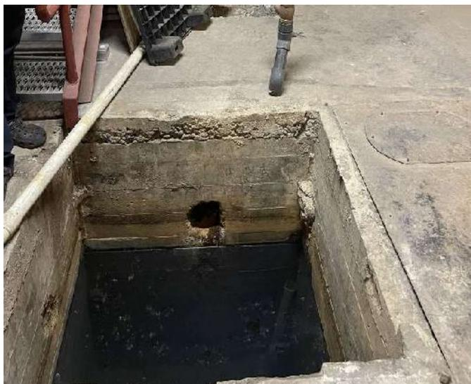
Sump #2 is located to the bottom right of the stairs seen in the previous picture. Sump #2 will also be enclosed similarly to Sump #1 with temporary air ducting between the two sumps being hung from overhead to minimize disruption to MWH activities.
