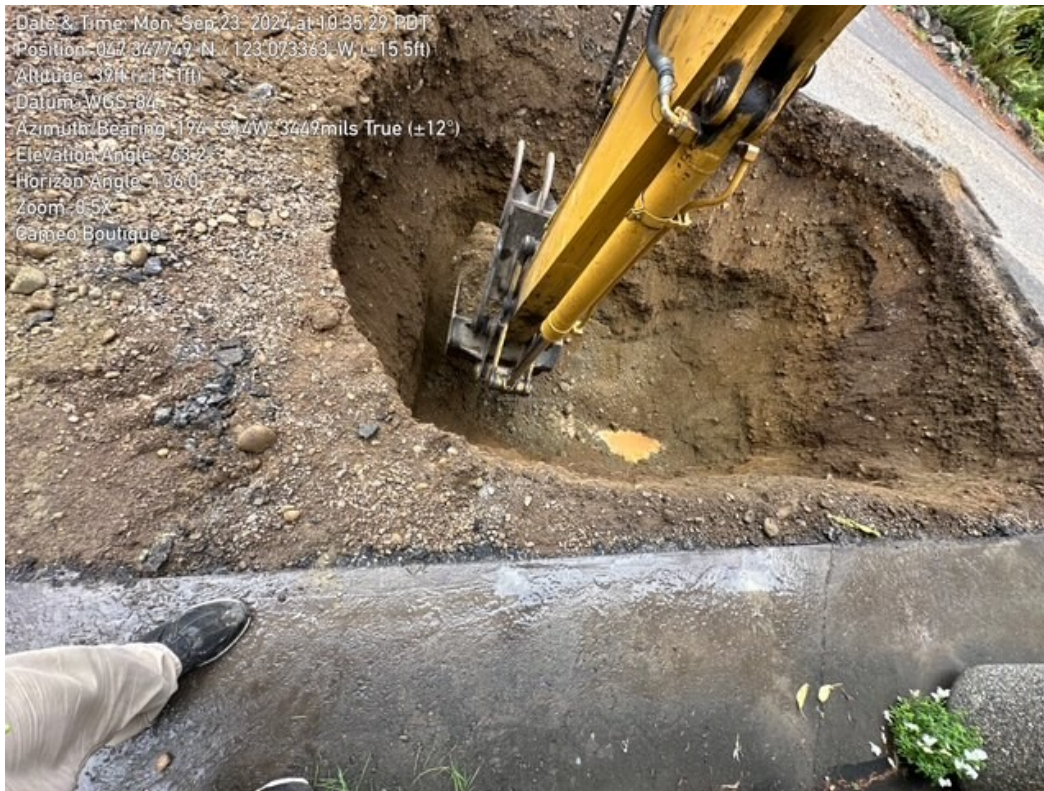
Photograph 4.3 The remedial excavation proceeded until a thin lens of GRO impacted soil was removed directly above the static water level.
