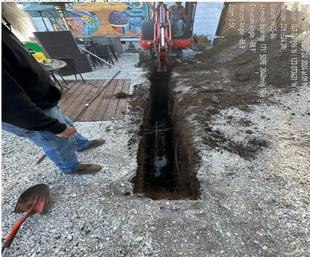
Photograph 4.8. View of trench excavated to install the northern sparge line.
