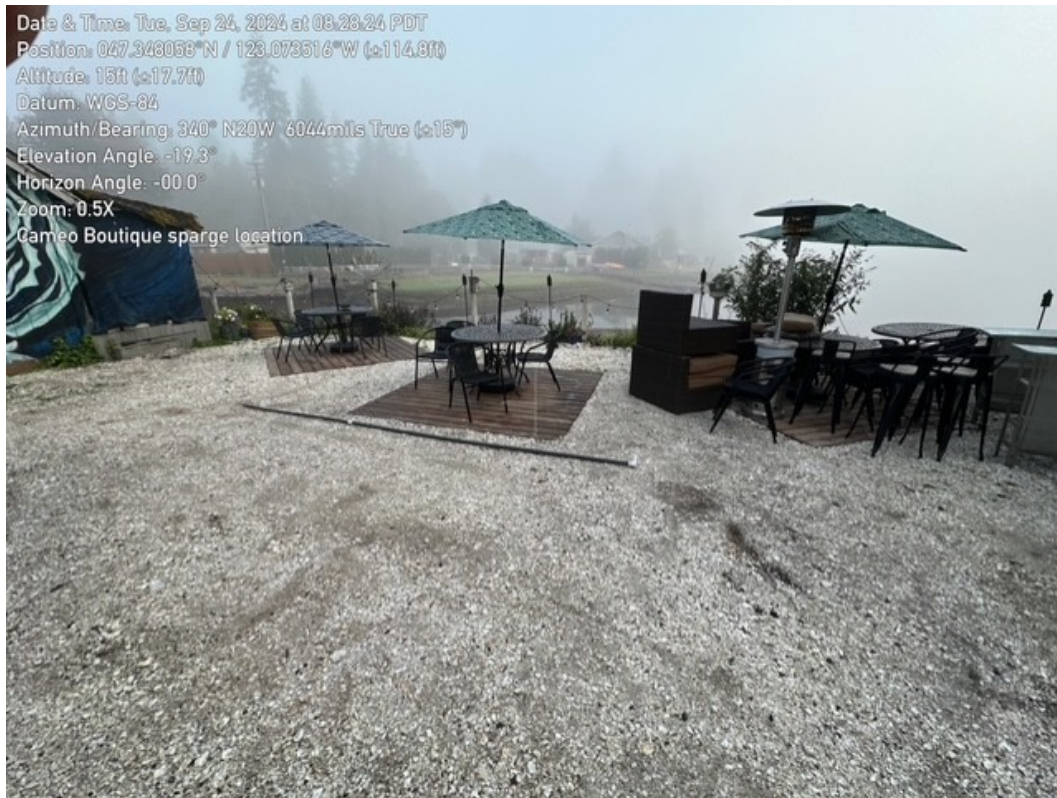
Photograph 4.7. View of the northern air sparging line laid out prior to the excavation of the sparging trench.
