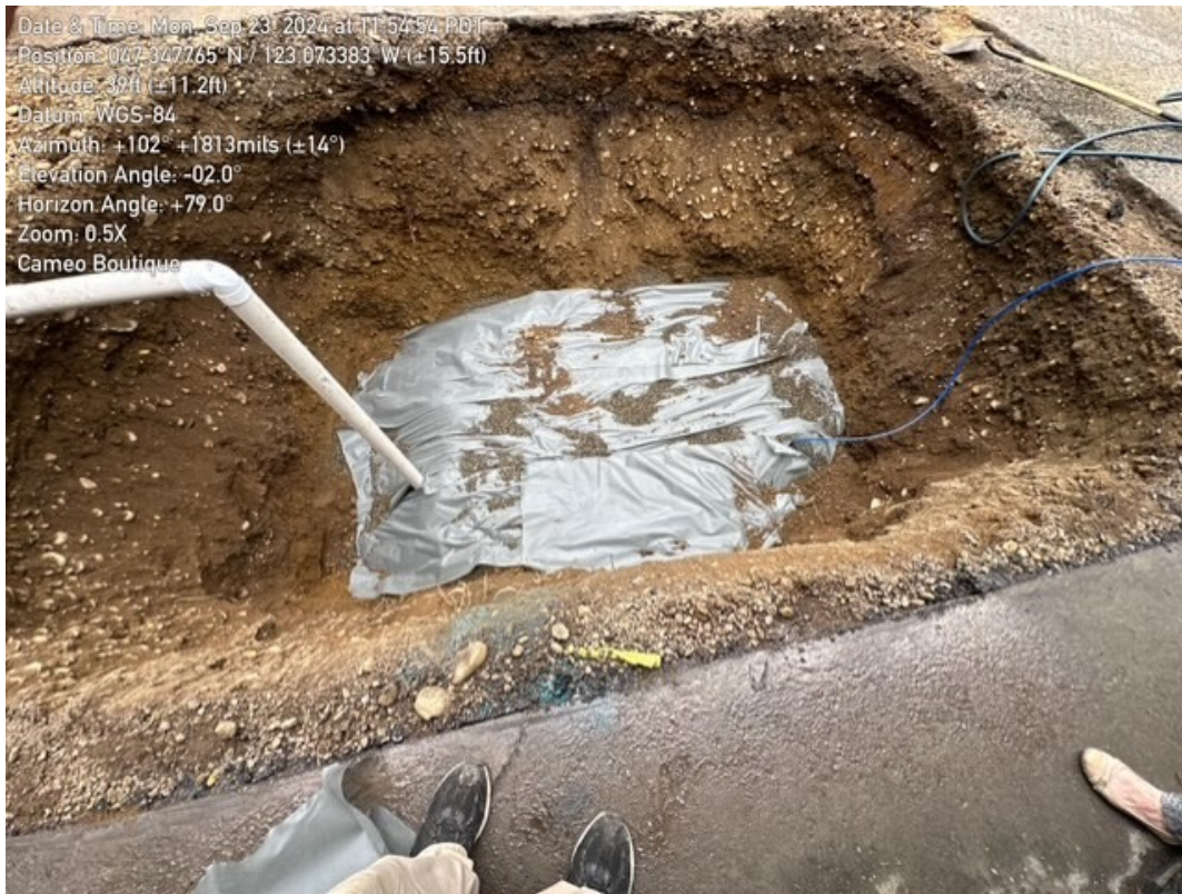
Photograph 4.5 The pea gravel was filled up above the water level, then a 4-inch diameter passive air return was installed, and covered with filter fabric.
