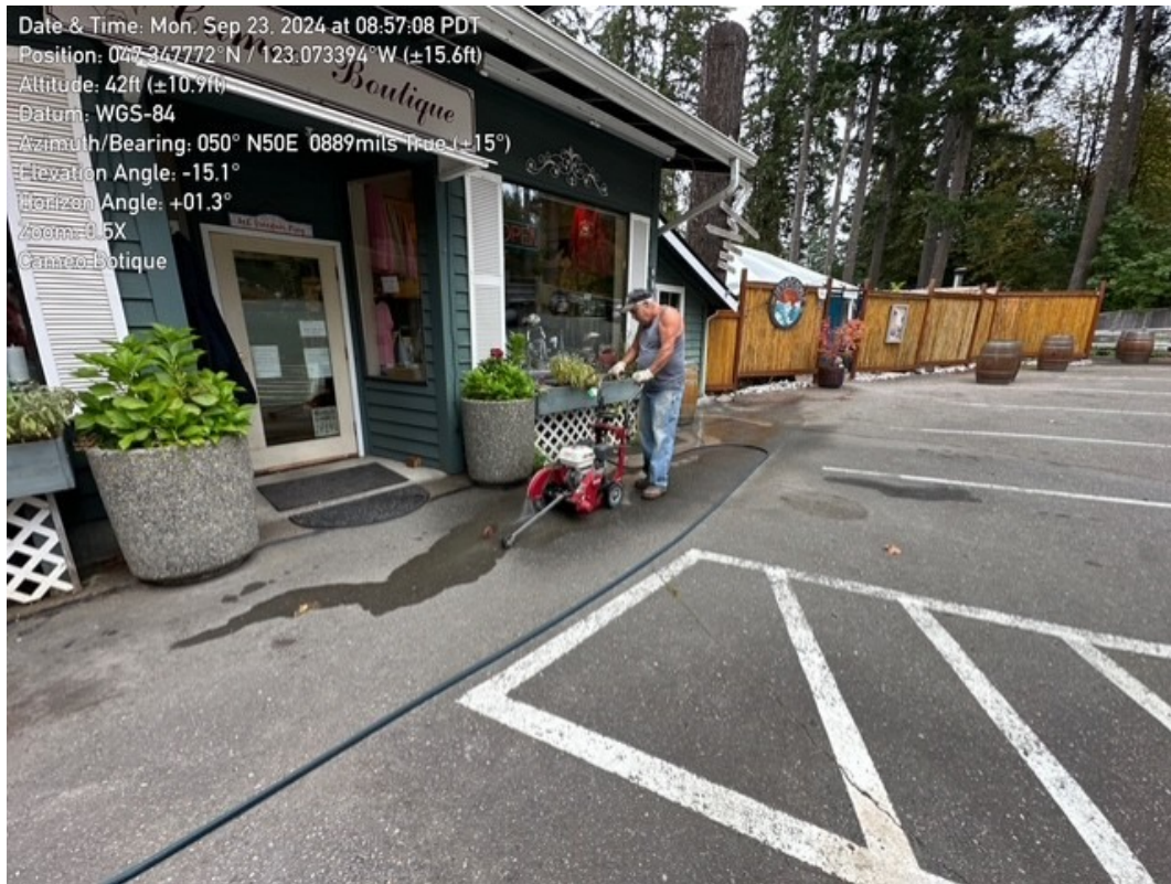
Photograph 4.1 View looking east of the project area. The asphalt was saw cut to prevent cracking.
