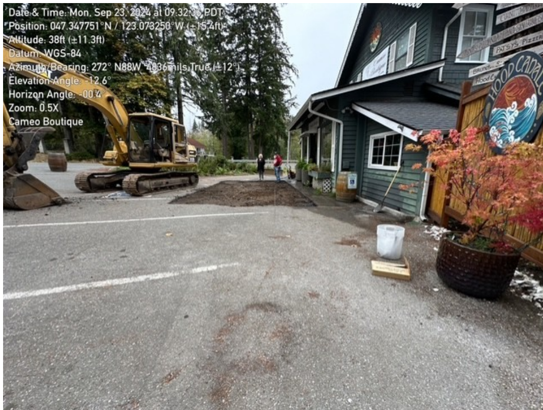
Photograph 4.2 The asphalt cover was removed from the project area.
