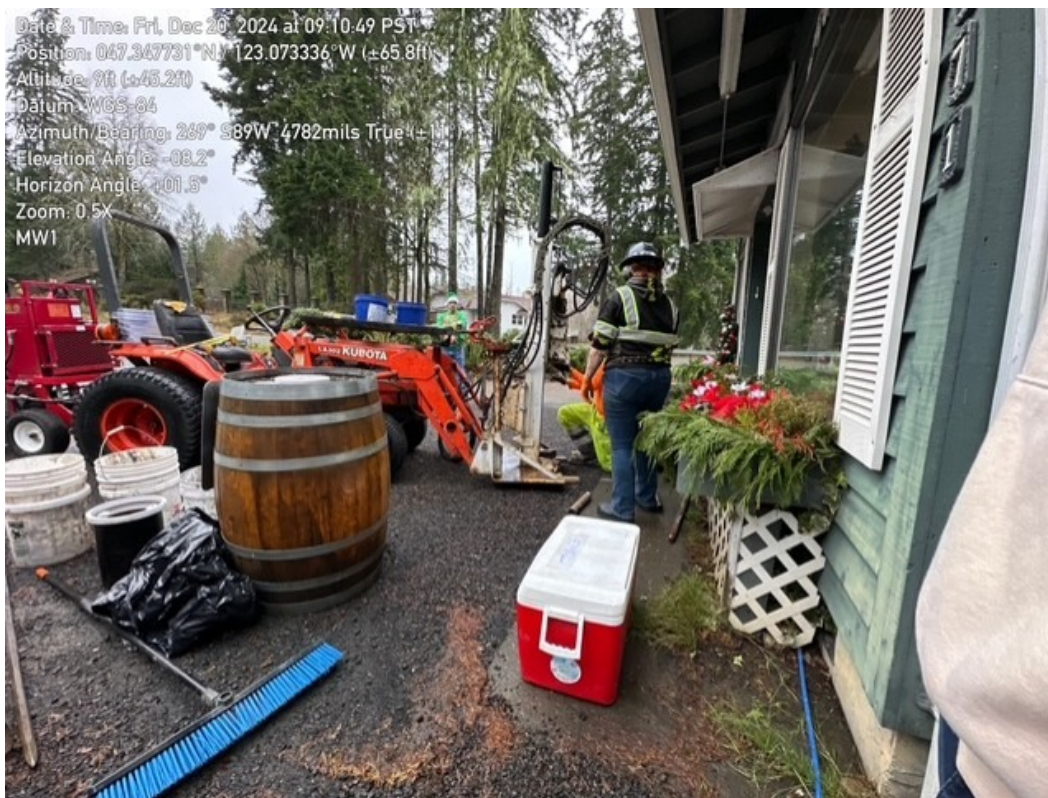
Photograph 4.9. View of Monitoring Well MW1 being installed.
