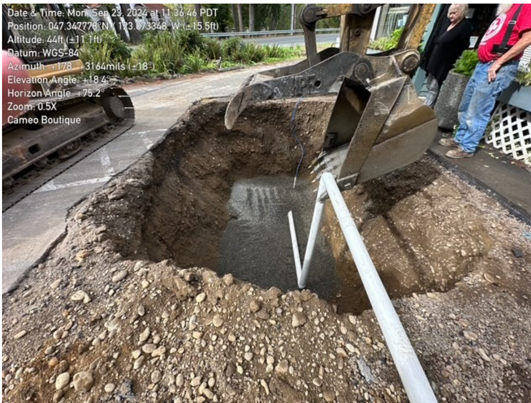
Photograph 4.4 View of the air sparging line being placed in a bed of pea gravel.
