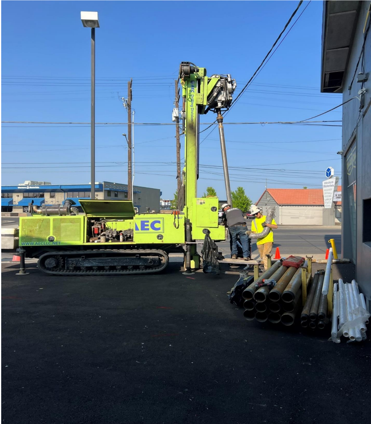
Photograph 2 – Anderson Environmental Contracting (AEC) employee carrying a soil sample bag from the drill rig to the geologist’s field table on May 19, 2023 (facing west).
