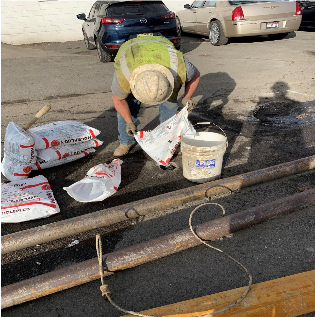
Photograph 12 – Driller’s helper pouring bentonite pellets into soil boring SB2, subsequent to soil sample collection.
