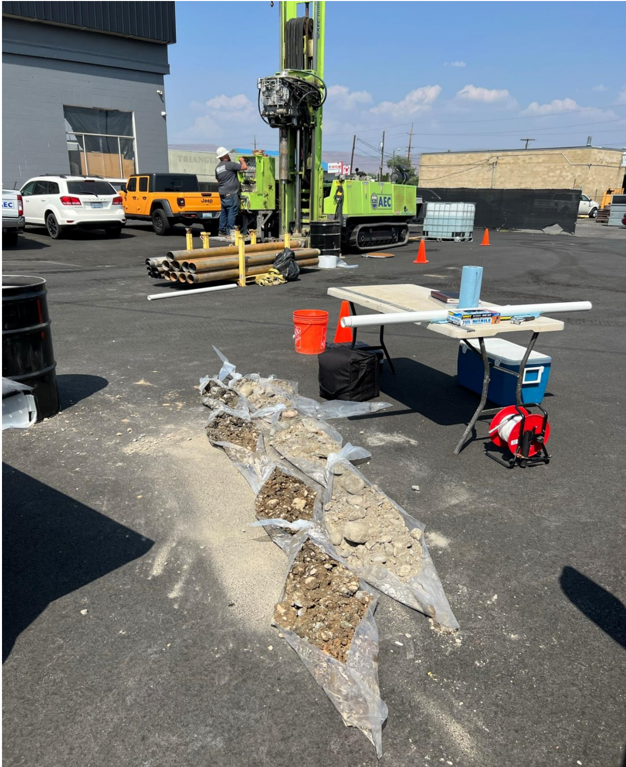
Photograph 8 – Soil lithology from 1 – 20 feet bgs in boring MW3A on May 19, 2023 (facing NE). Ten feet of soil cuttings still in the ground.
