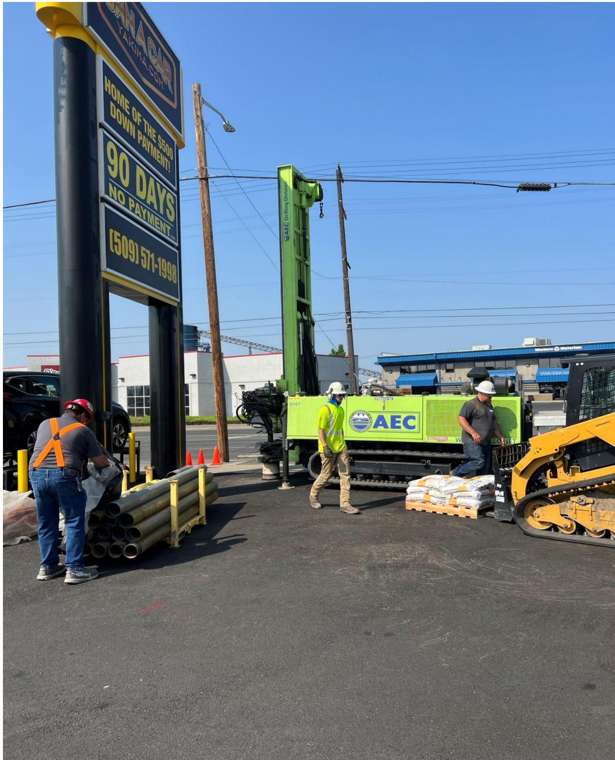
Photograph 3 – Terra sonic drilling rig set-up to advance boring MW8 on May 19, 2023 (facing west).
