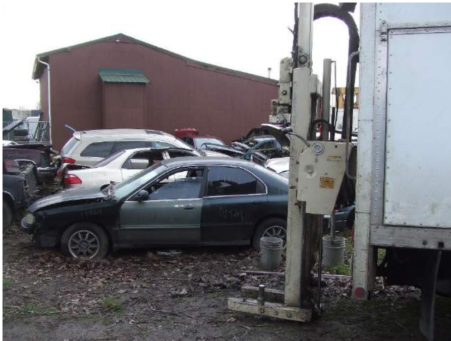
Photo 22. A view of the soil boring – B10.
