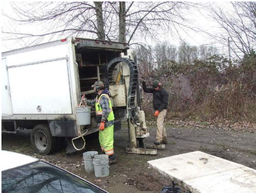
Photo 20. A view of the soil boring – B8.
