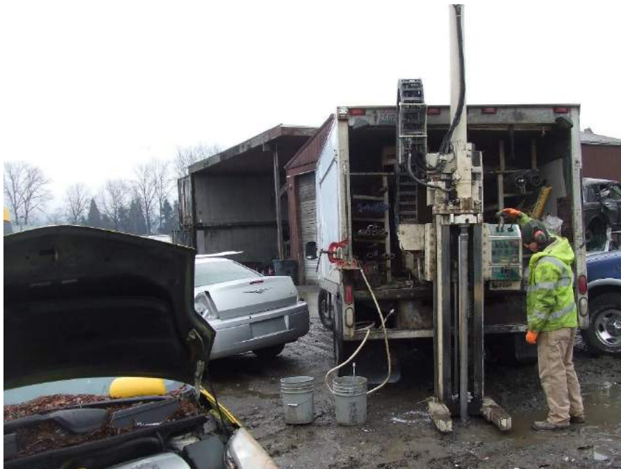
Photo 18. A view of the soil boring – B6.
