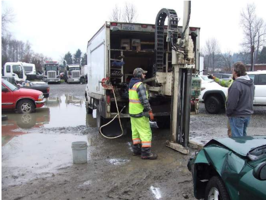
Photo 15. A view of the soil boring – B3.
