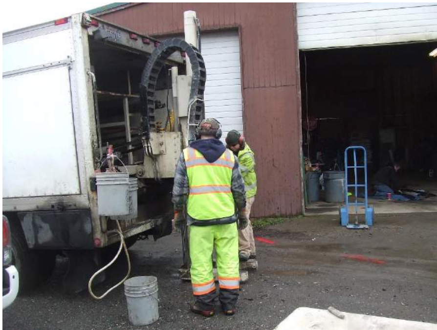
Photo 16. A view of the soil boring – B4.
