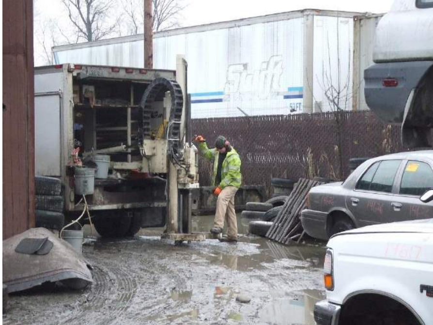
Photo 17. A view of the soil boring – B5.
