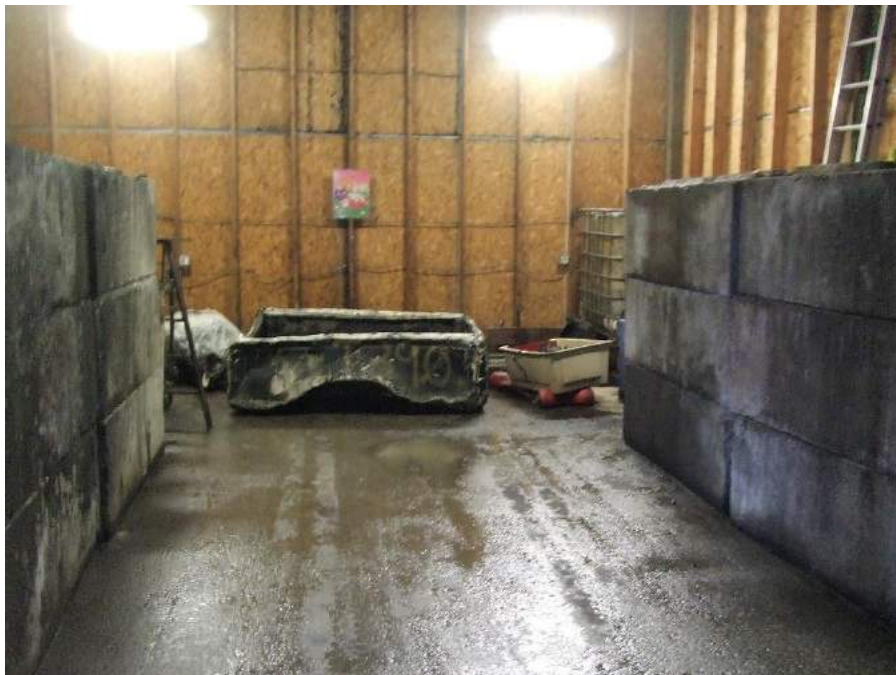
Photo 8. An inside view of the dismantling building.
