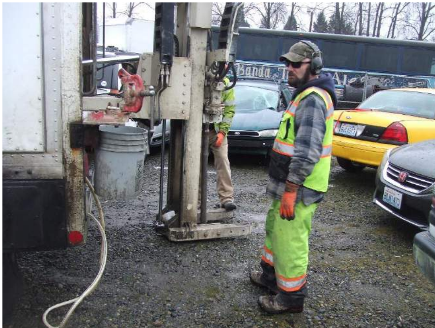
Photo 14. A view of the soil boring – B2.
