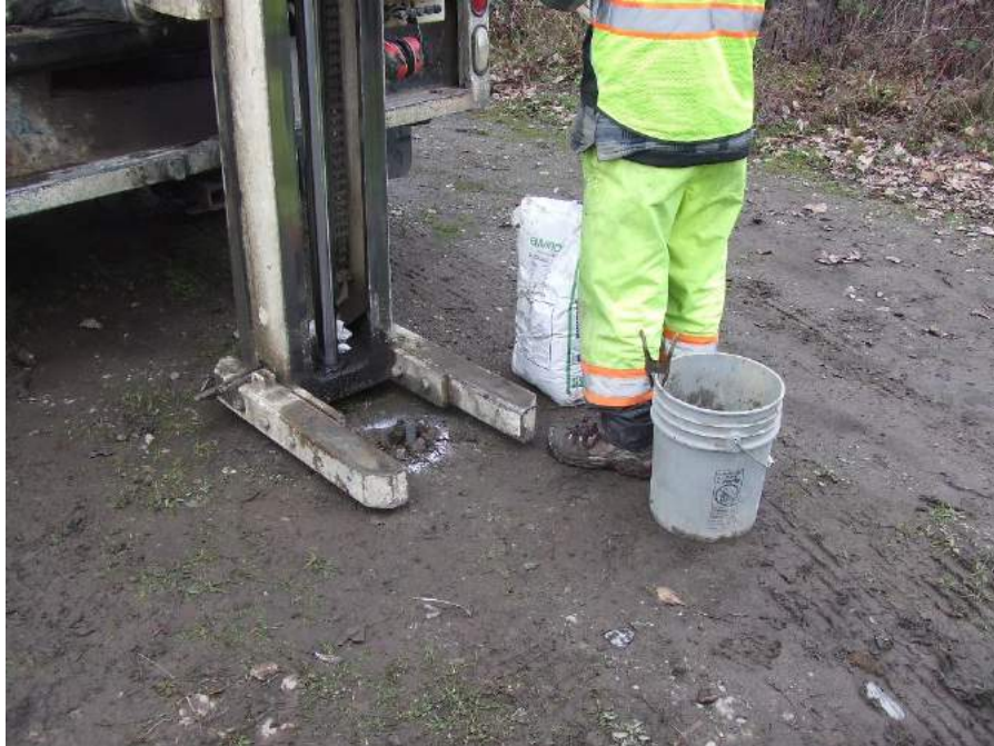
Photo 21. A view of the soil boring – B9.
