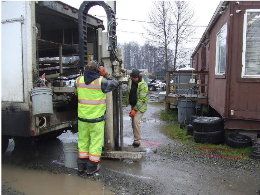
Photo 13. A view of the soil boring – B1.
