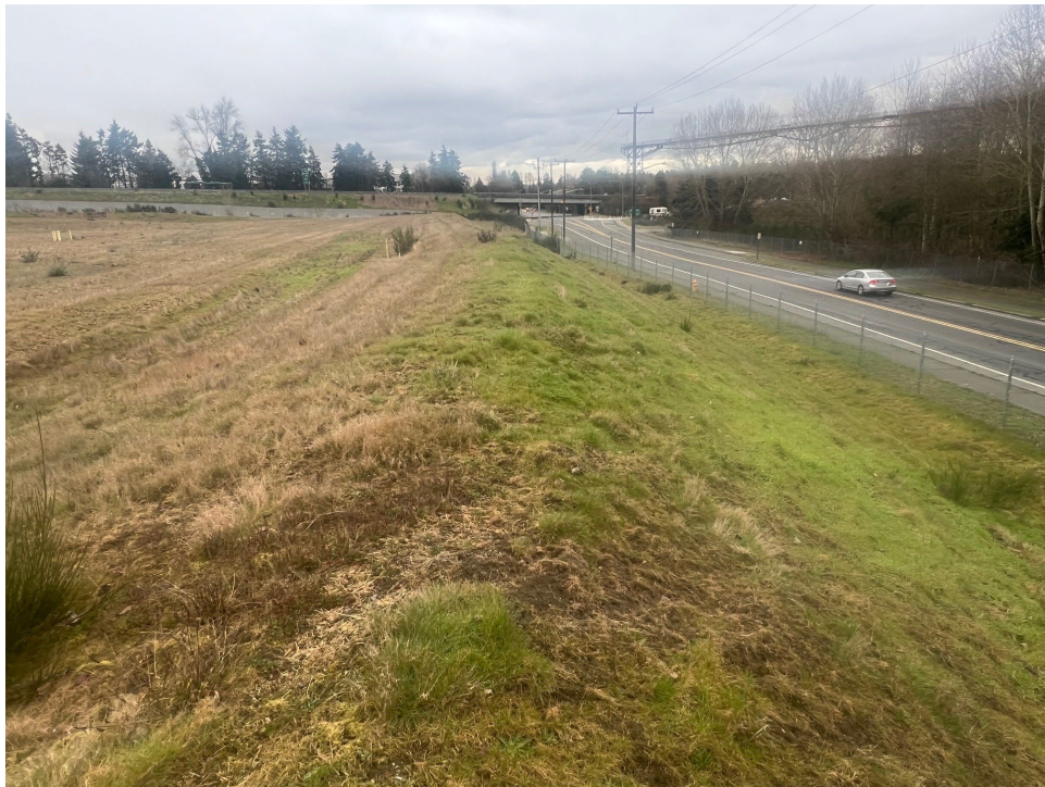
Photograph 6. Reseeded area near Station LLA 16 at the Lora Lake Apartments Parcel looking north. The area previously showed signs of exposed underlying soil, animal burrowing, and loss of barrier material.
