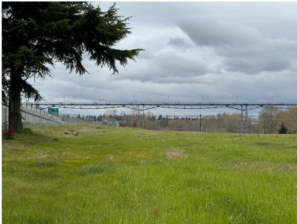
Photograph L2. Stations LLA 03, LLA 04, and LLA 05 in good condition.
