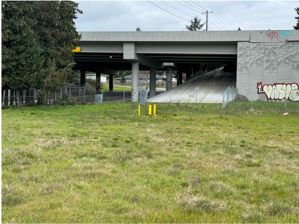
Photograph L3. Stations LLA 07, LLA 08, LLA 09, and LLA 10 in good condition.
