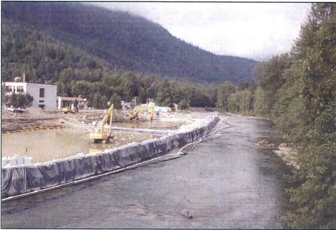
Figure 3. Overview of the western end of the Interim Action showing the coffer dam along the left bank of the South Fork Skykomish River.
