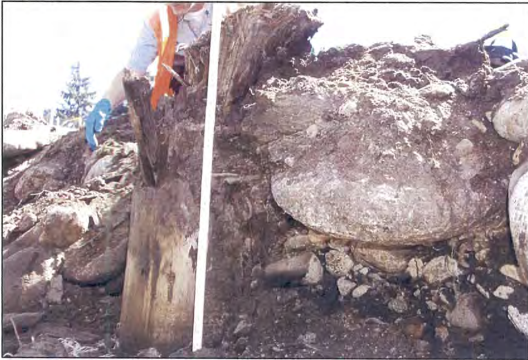
Figure 7. Remains of a buried wooden retaining wall in Area A.
