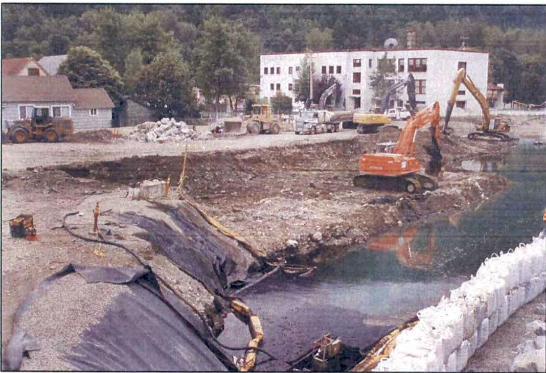
Figure 4. Example of the terraced configuration used to excavate contaminated sediments.
