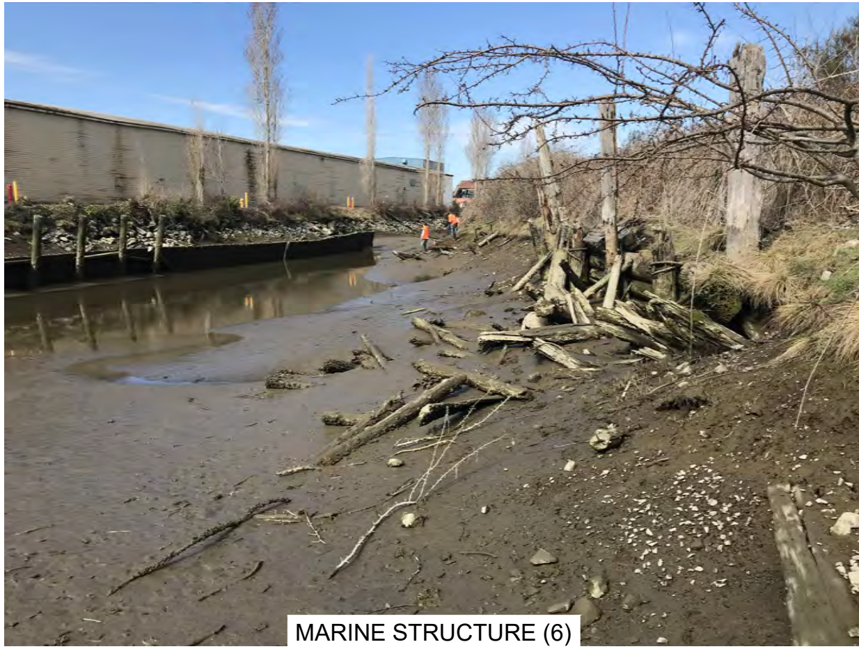
MARINE STRUCTURE (6) VIEW 2
