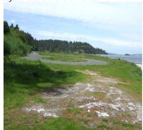
Photo 1: Nearshore fill area looking North
