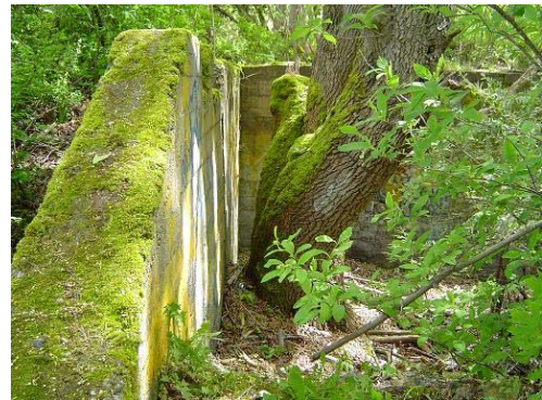
Photo 3: Typical building foundation remnant
