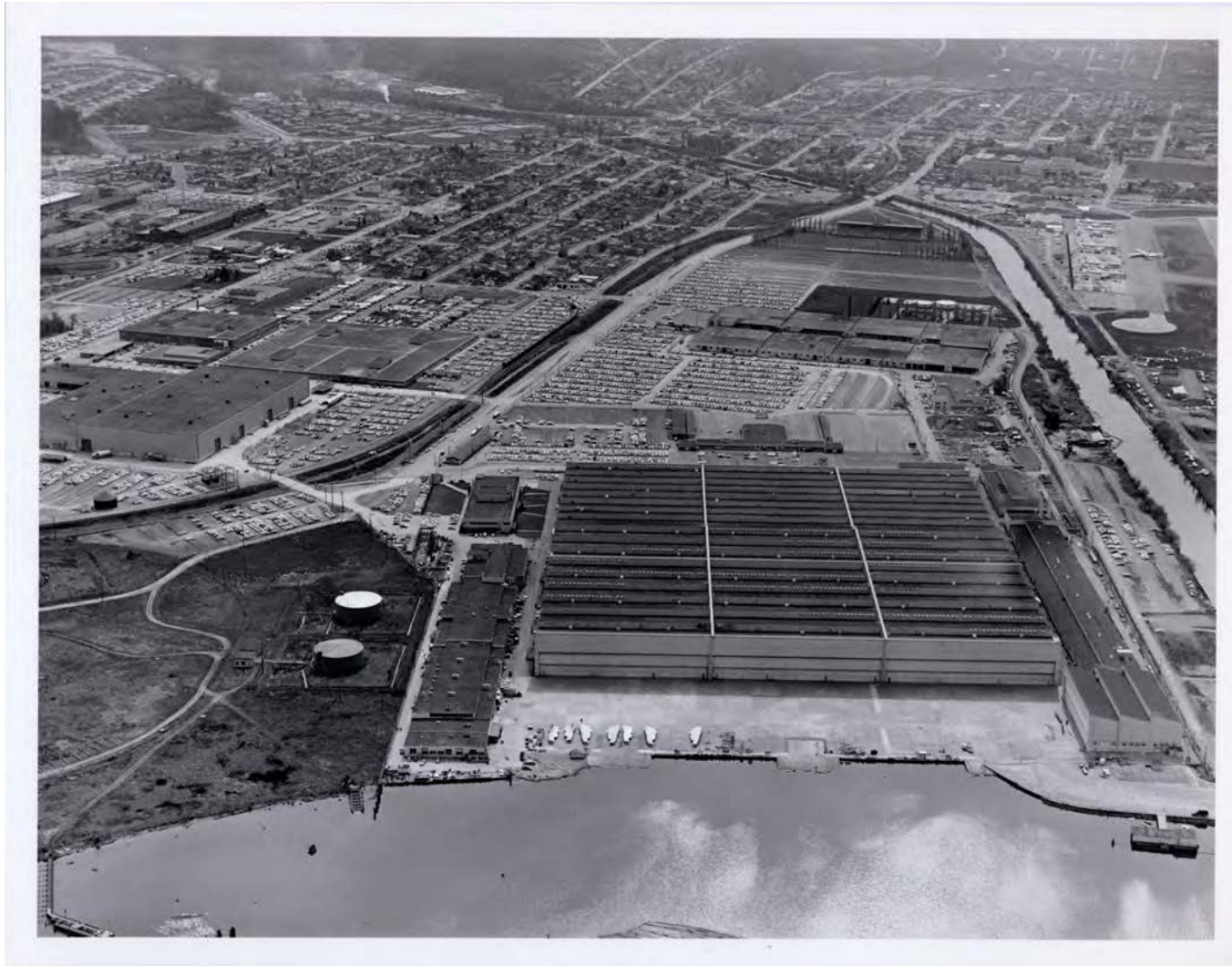
Photo 2. Aerial photo from approximately 1960 of the area containing a portion of the current Boeing Renton Facility. Important structures in the photo include the presence of the fueling dock (bottom left) and two large oil tanks for Shuffleton power plant, with associated pump house and containment berms. The pipelines are above ground by the tanks as they bend over the berms and 2 fuel lines appear to be above ground to the fueling dock. Some type of structure exists on land at end of the fueling dock and is included on 1967 drawings. This 1960 aerial photo is before Boeing Buildings 4-81/82 and Apron R were constructed in 1967.
