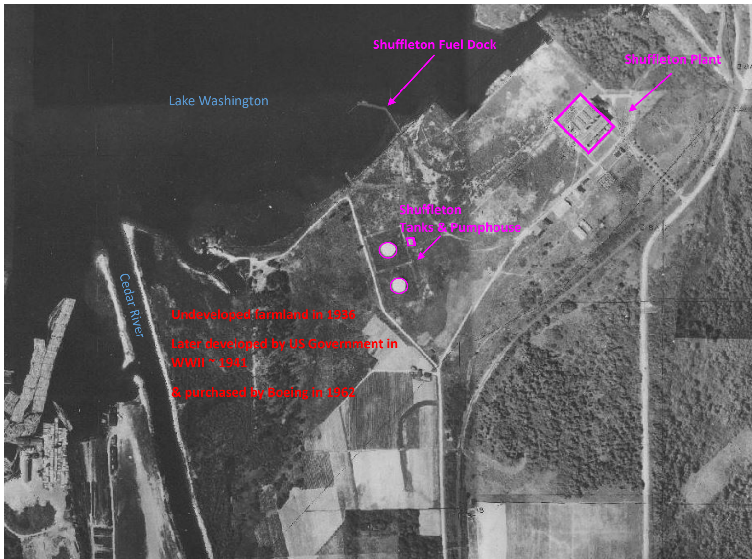
Photo 1. Aerial photo from 1936 of the area, this pre-dates Boeing and is all as farmland. Important structures in the photo are the Shuffleton power plant with the associated fueling dock and two large oil tanks.
