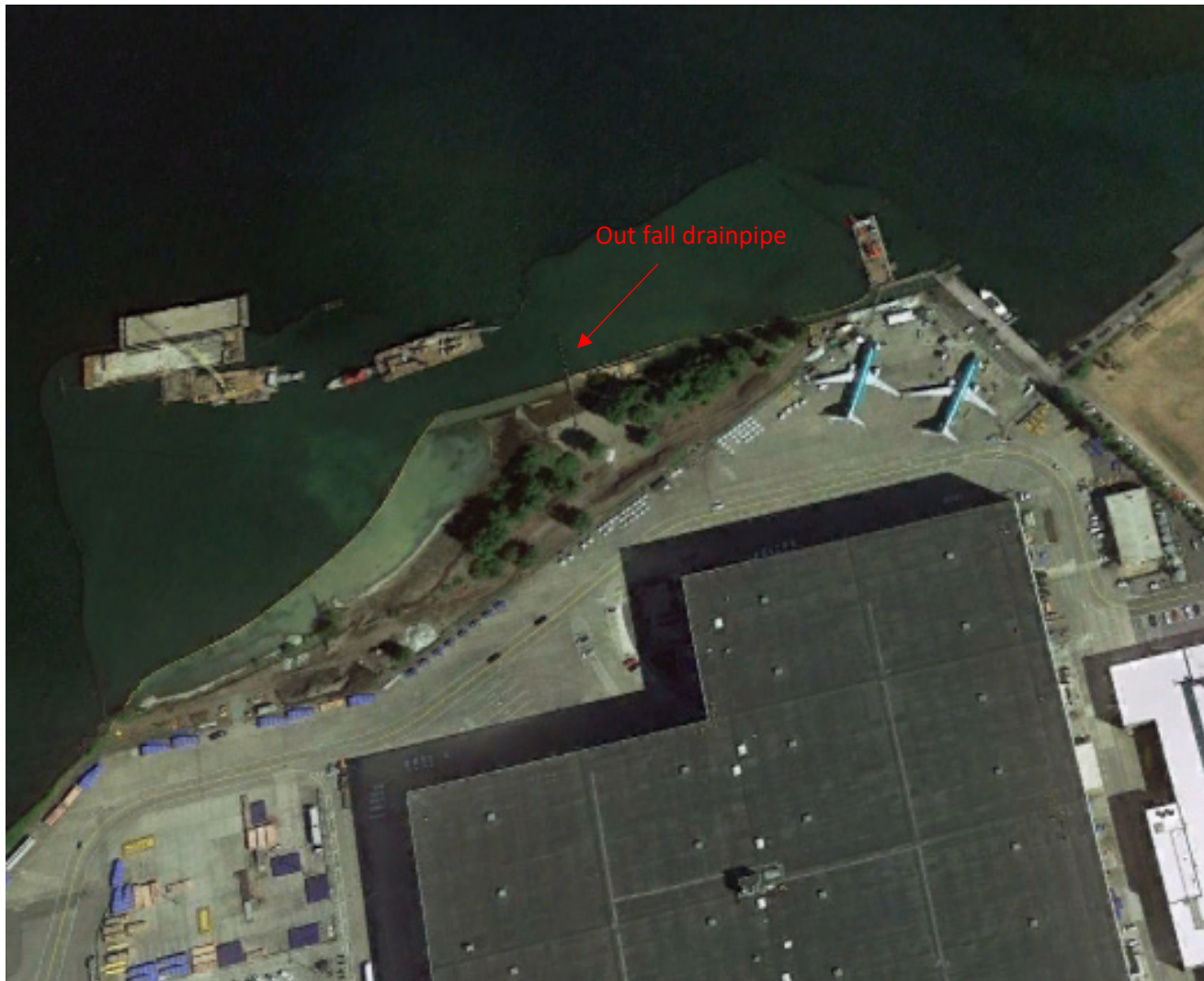
Photo 6. 2014 Aerial photo of Apron R and Building 4-81/82. The storm drain outfall is visible during the removal of the cooling water discharge channel from the Shuffleton Power plant (this work was completed by others at the start of the Southport redevelopment)
