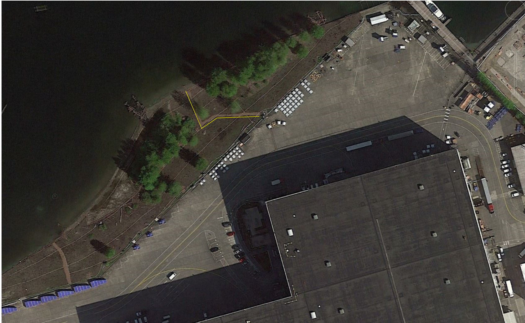
Photo 7. 2015 Aerial photo of Apron R and Building 4-81/82. With a visible excavation line in the DNR lease parcel (leased to PSE) where the storm water drain has been buried. The location of the storm water lines to outfall would have crossed path with any historical lines from the prior Shuffleton refueling dock.
