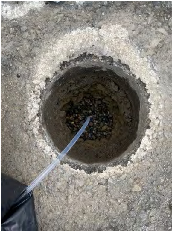
Figure 2 – Pea gravel placed to the top of the vapor pin screen
