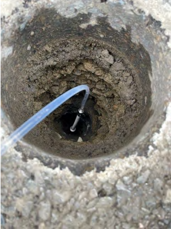
Figure 2 – Pea gravel placed to the top of the vapor pin screen
