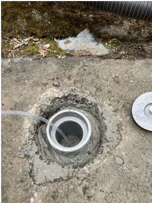
Figure 4 – Monument set with cement, compression seal cap to the side.
