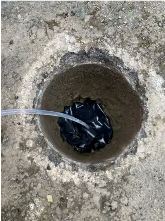
Figure 4 – Monument set with cement, compression seal cap to the side.
