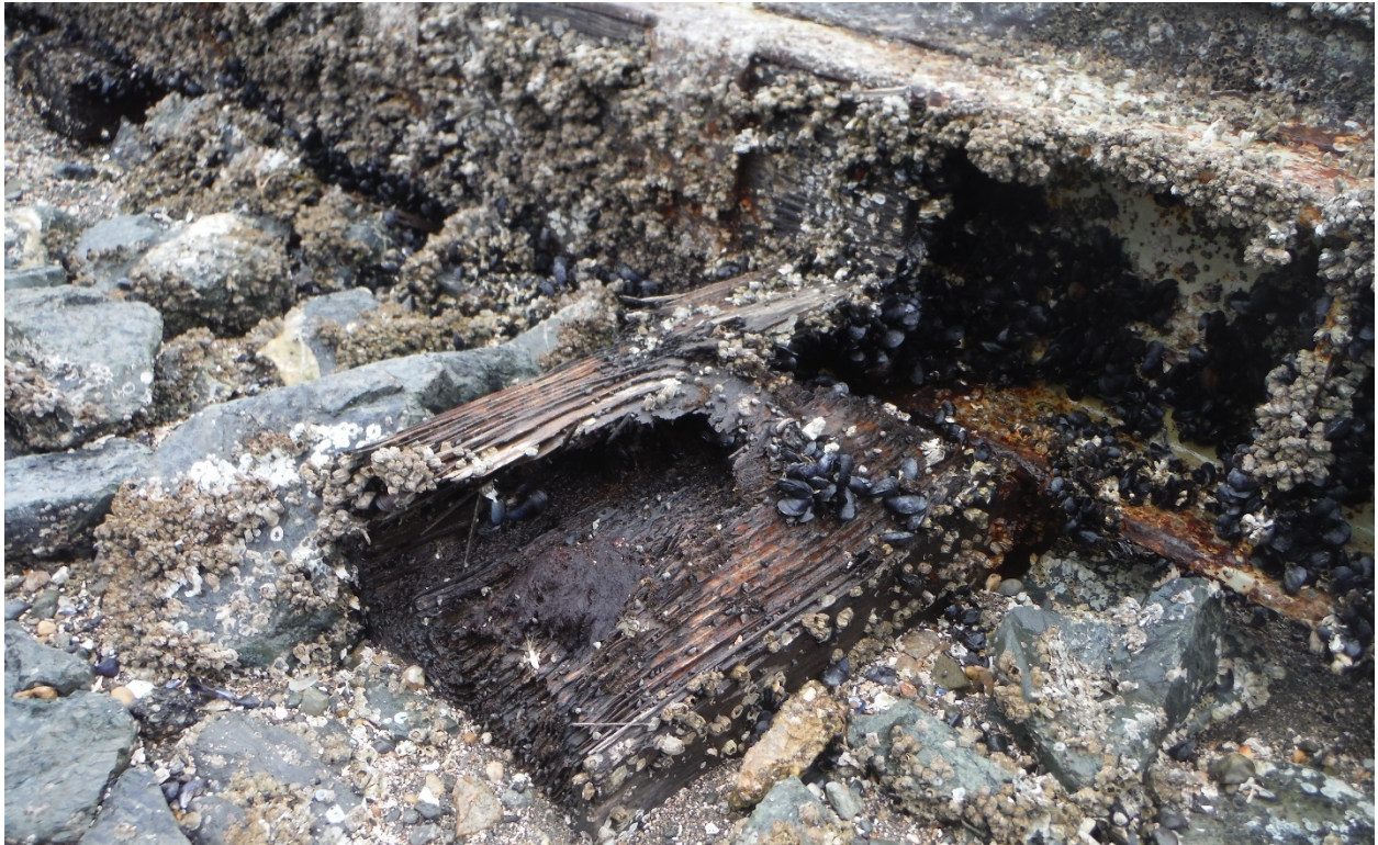
Photo 15 – Rotted Timber Tie
