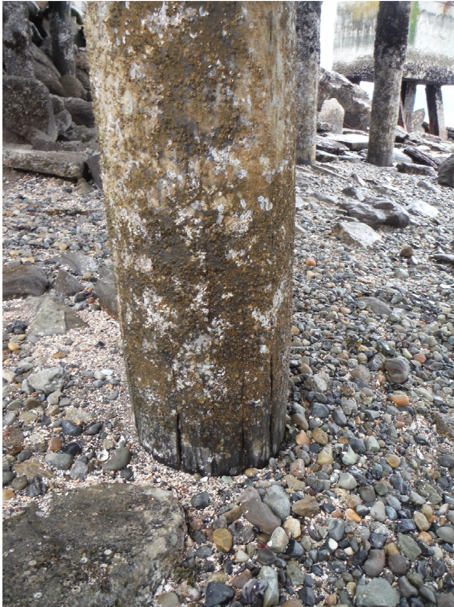
Photo 3 – Typical Pile with Minor Damage
