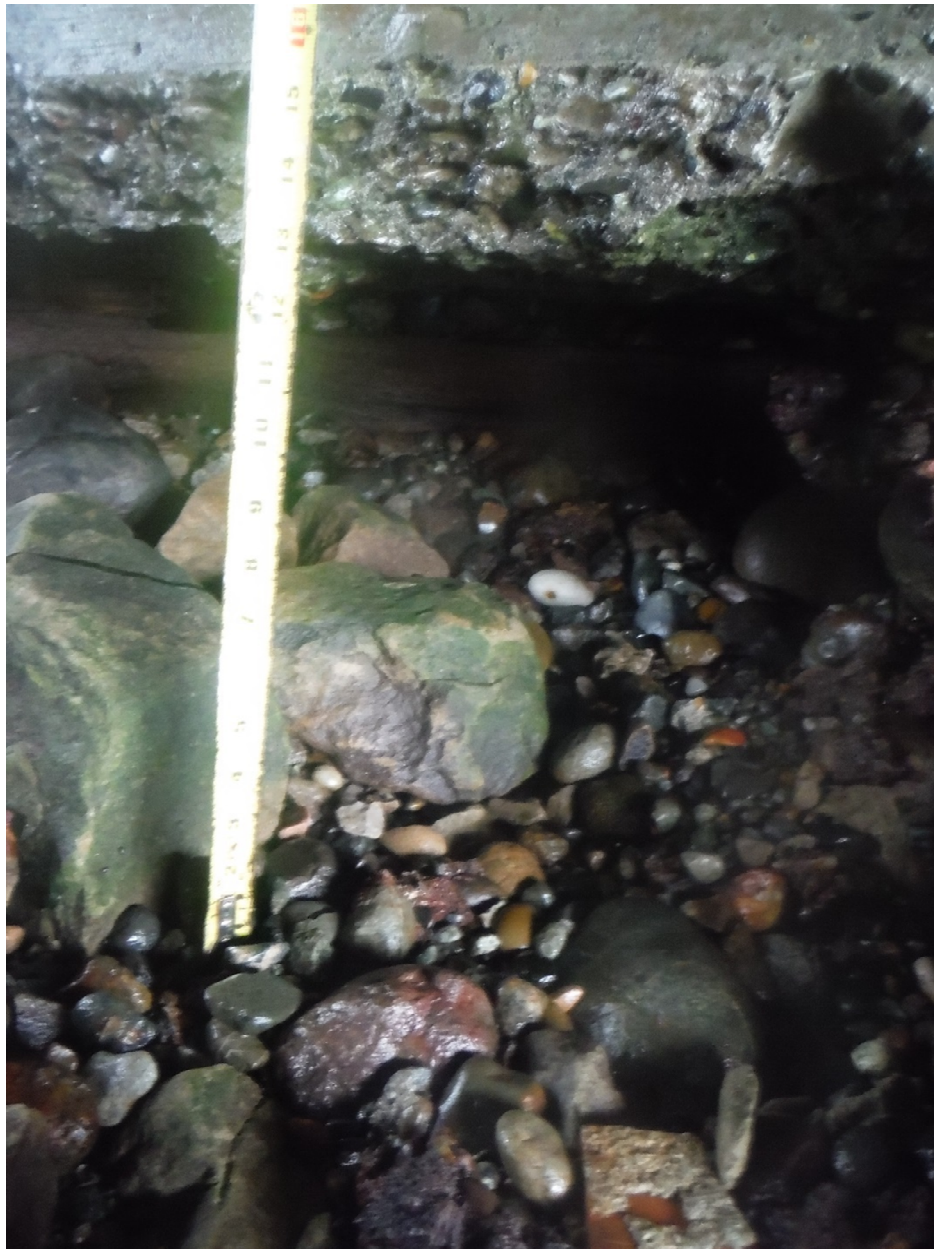
Photo 8 – Soil Undermining Bulkhead Wall
