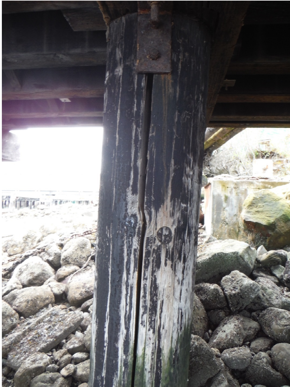
Photo 5 – Bent 2 Pile C (Mechanical Split)
