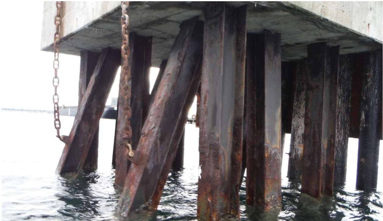
Photo 9 – Northwest Dolphin Corroded and Buckled Pile
