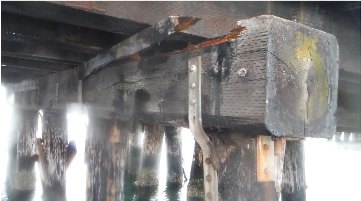
Photo 6 – Bent 10 (Splitting and Crushing)
