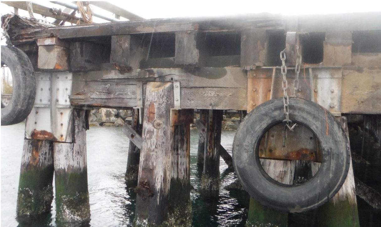
Photo 7 – Bent 11 (Mechanical Damage)
