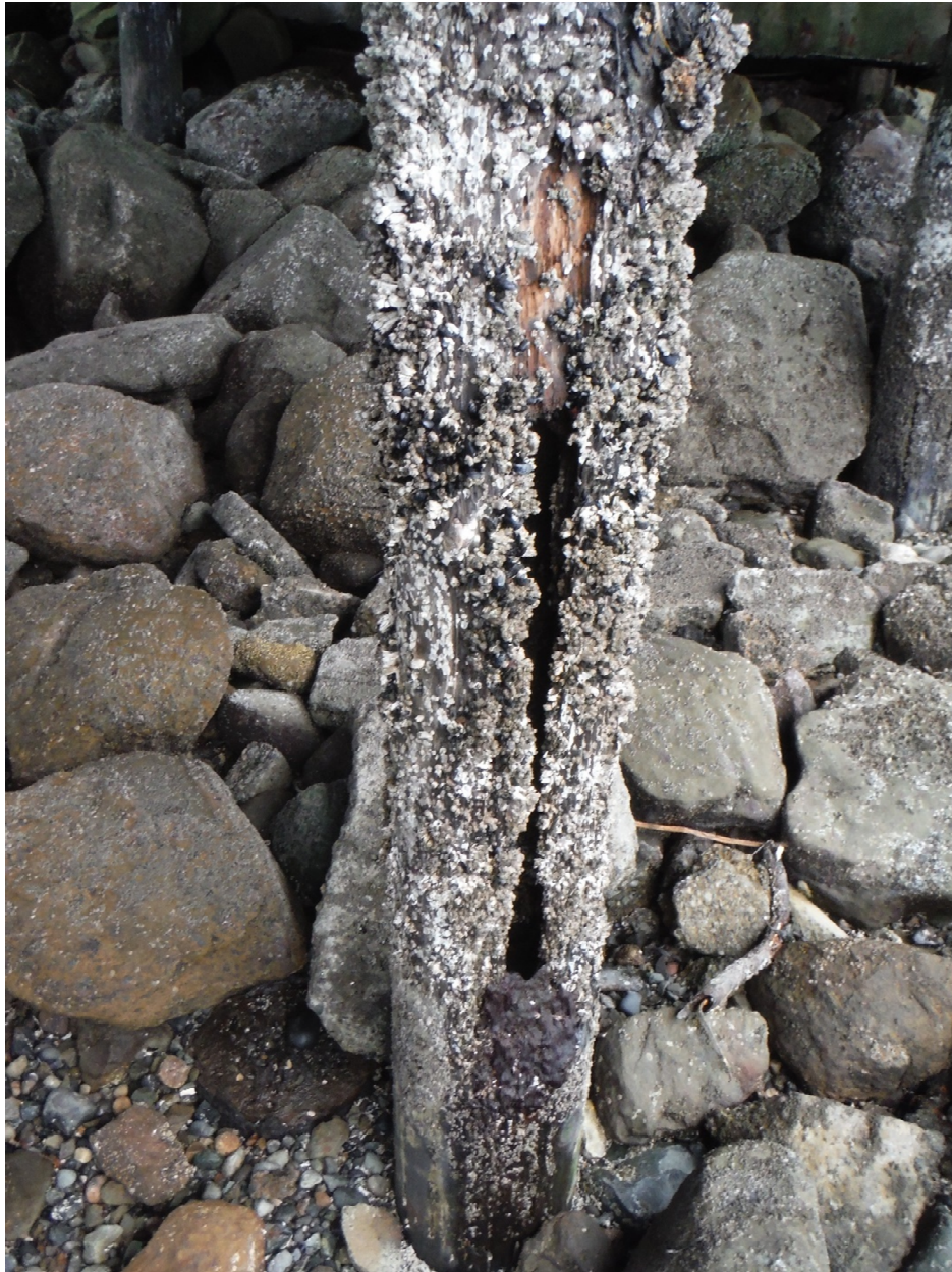
Photo 4 – Bent 2 Pile D (80% Section Loss)
