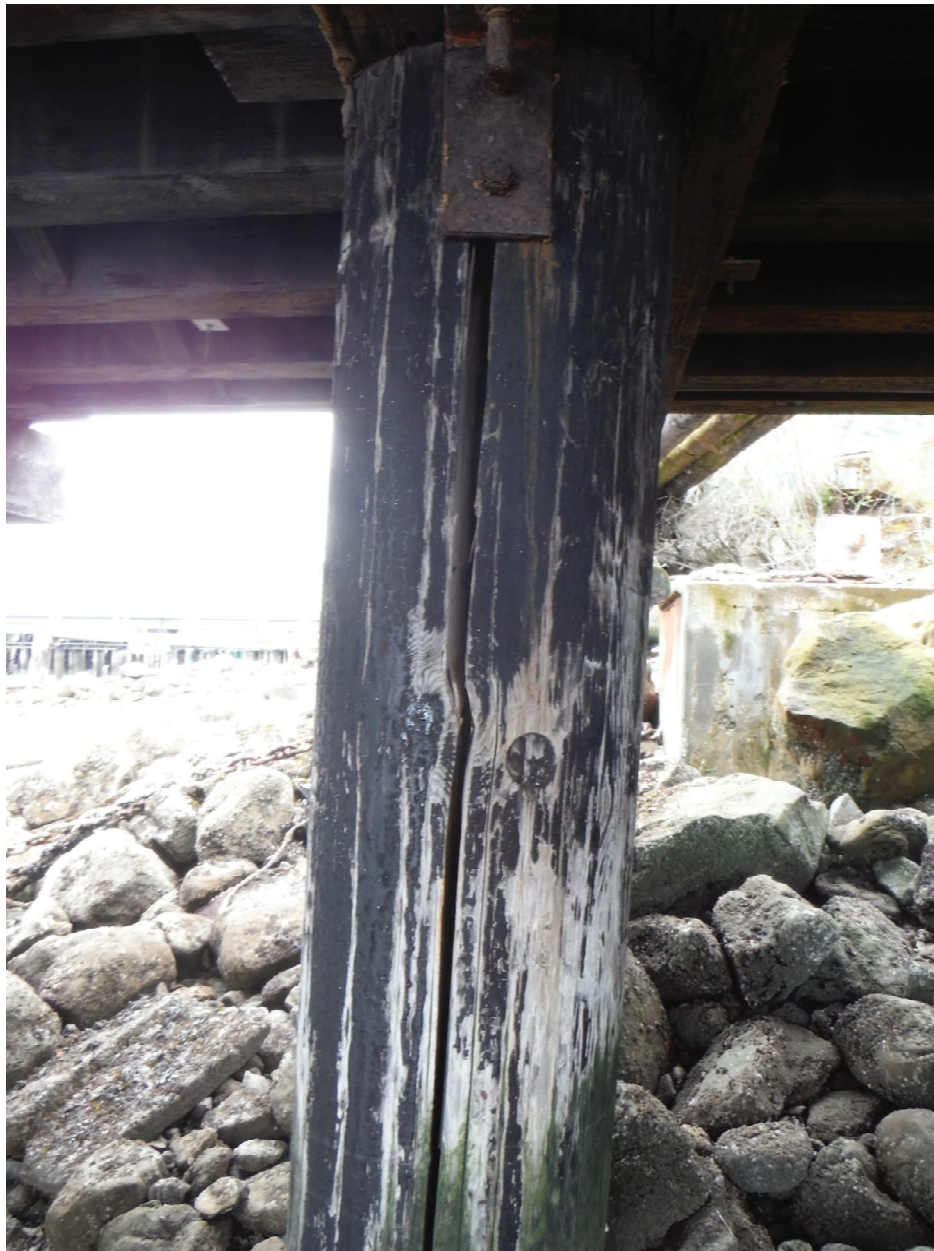
Photo 5 – Bent 2 Pile C (Mechanical Split)
