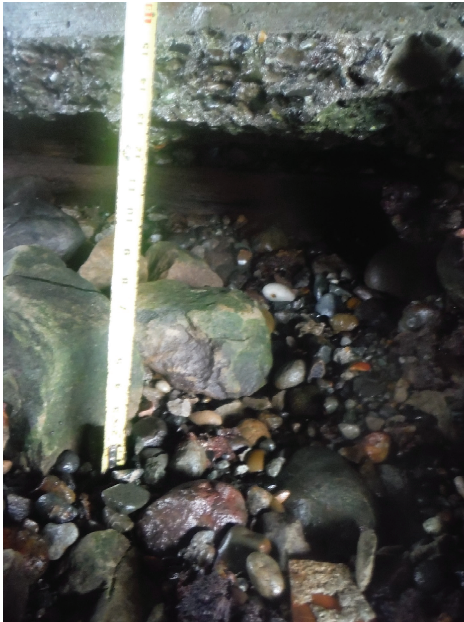
Photo 8 – Soil Undermining Bulkhead Wall
