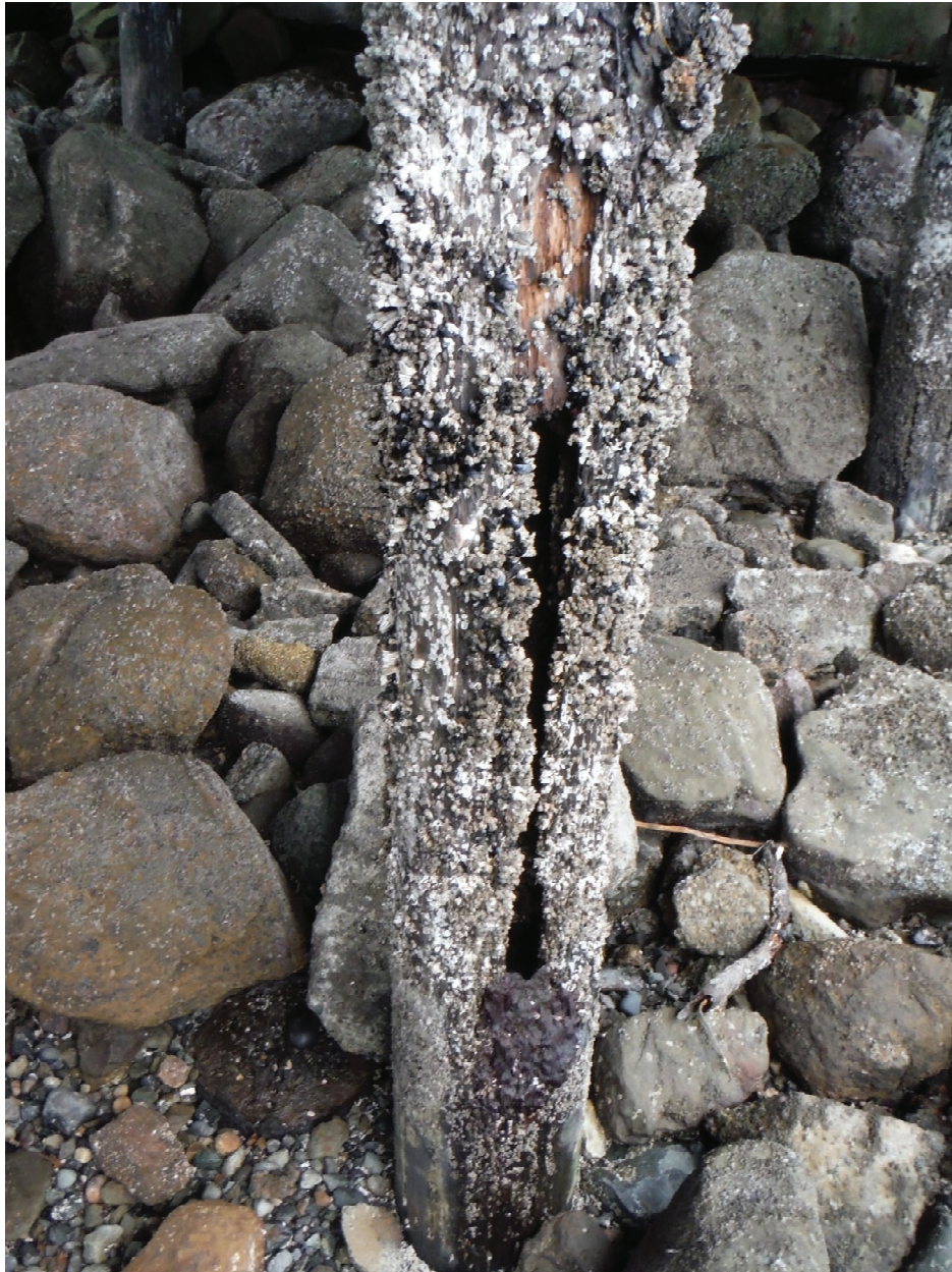
Photo 4 – Bent 2 Pile D (80% Section Loss)
