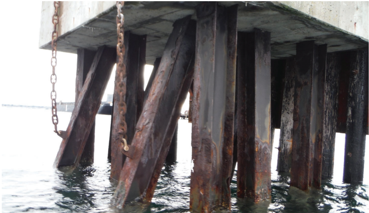
Photo 9 – Northwest Dolphin Corroded and Buckled Pile
