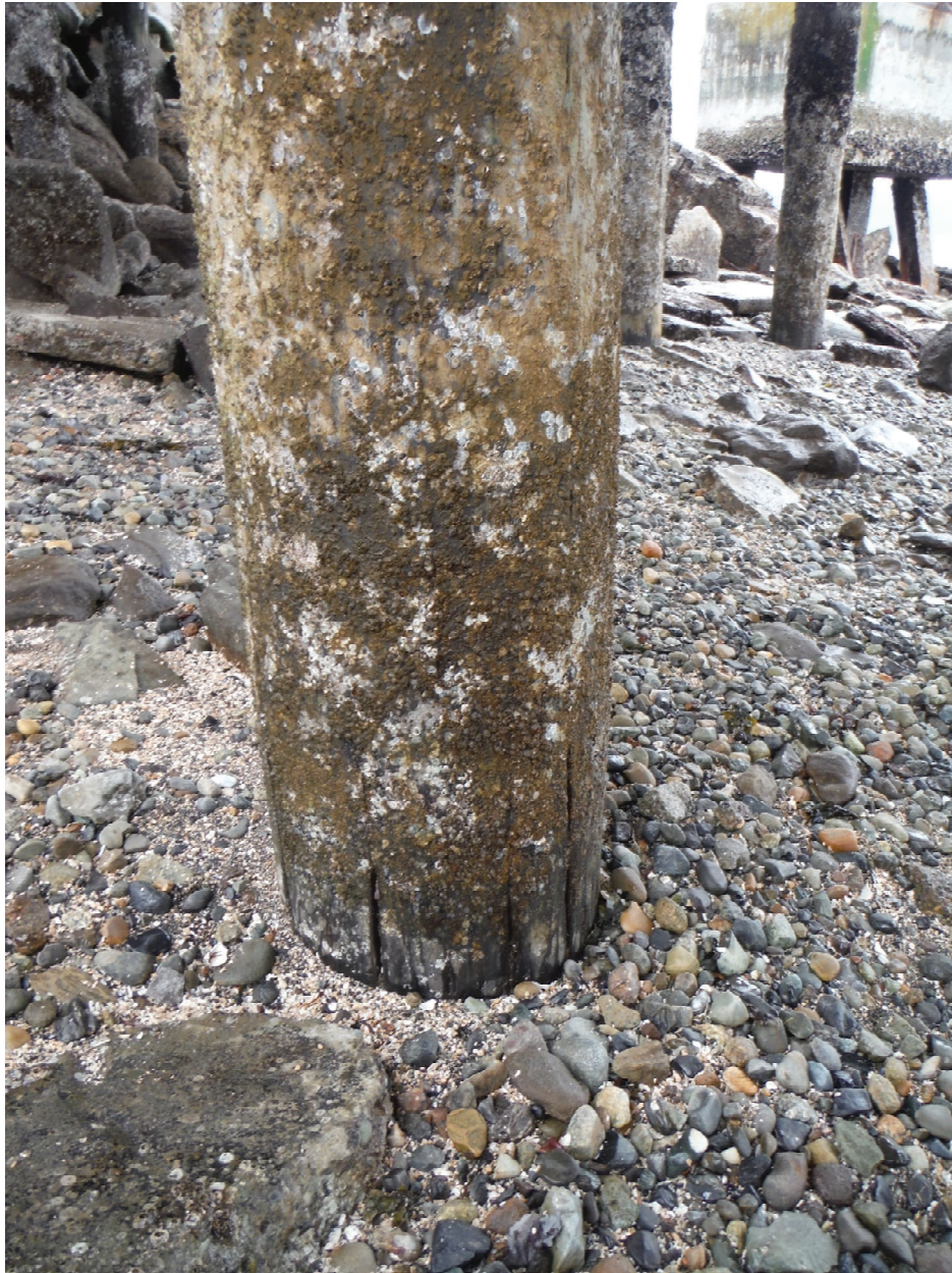
Photo 3 – Typical Pile with Minor Damage
