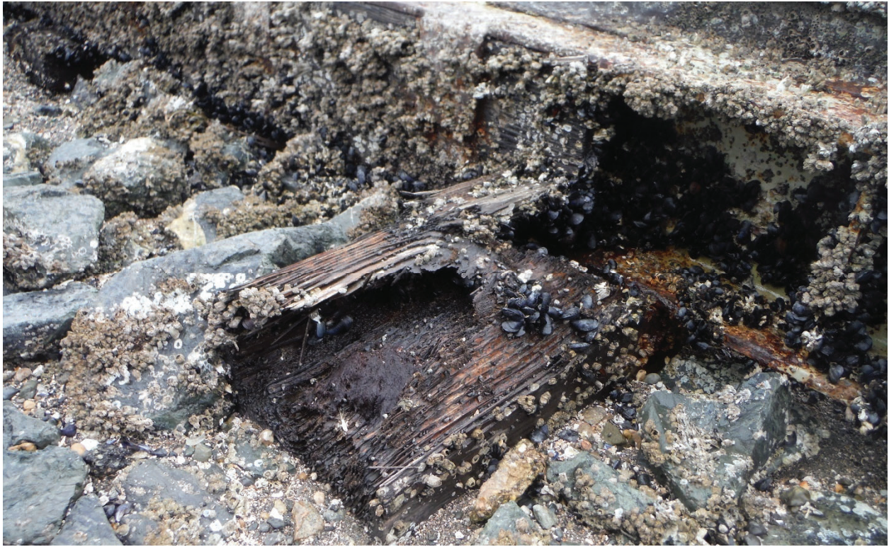
Photo 15 – Rotted Timber Tie
