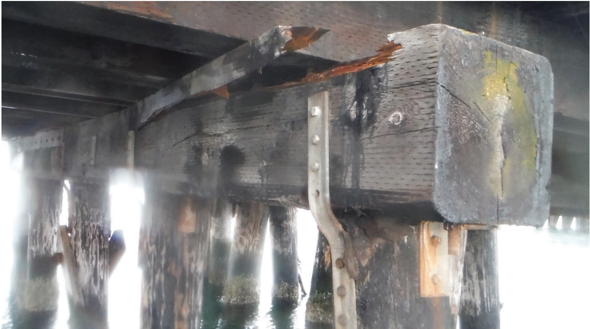
Photo 6 – Bent 10 (Splitting and Crushing)
