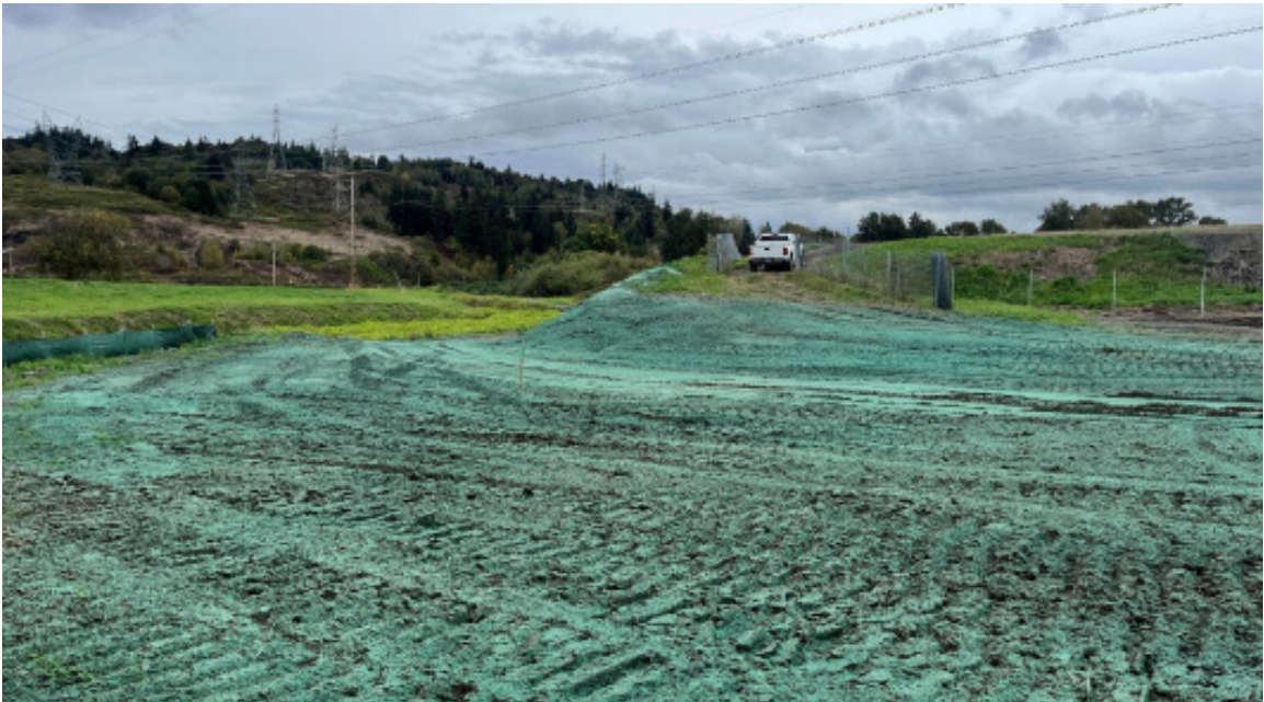
Hydroseed placement and chain-link fence reinstallation along segment 2
