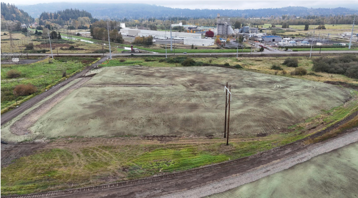
Hydroseeding and silt fence removal
