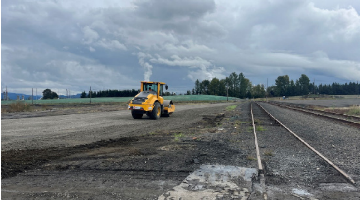
Compaction of crushed surfacing gravel material over select fill
