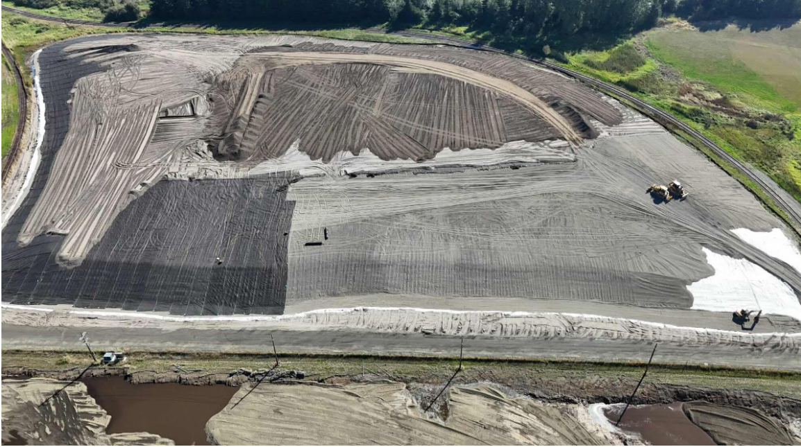
Cap installation: placement of drainage layer material, non-woven geotextile, general fill, and topsoil
