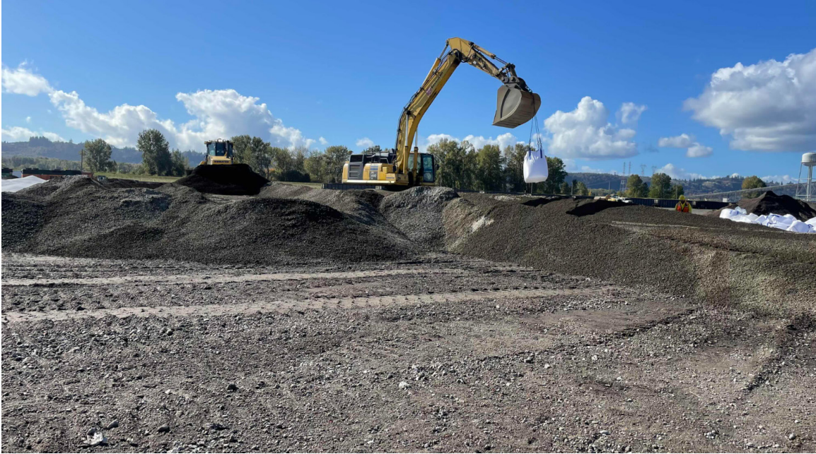
Mixing reactive backfill for placement into SU3
