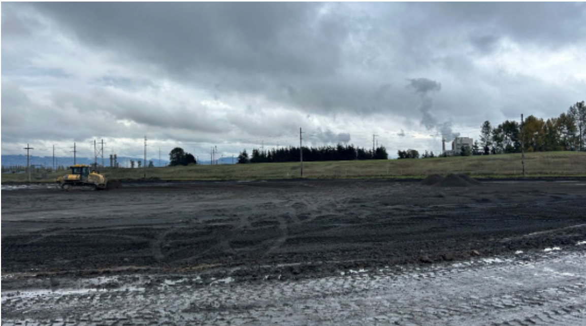
Placement of select fill over reactive backfill
