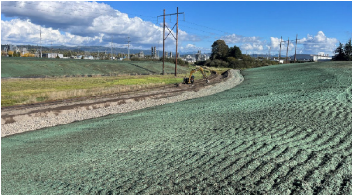
Northern perimeter ditch construction and hydroseed placement
