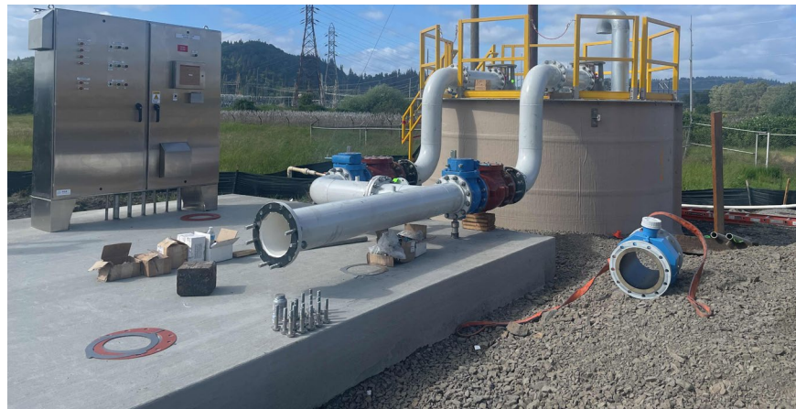
Catworks Construction (Catworks), installed East Landfill No. 1 Pump Station wet well, piping, and flow meters (facing northwest).
