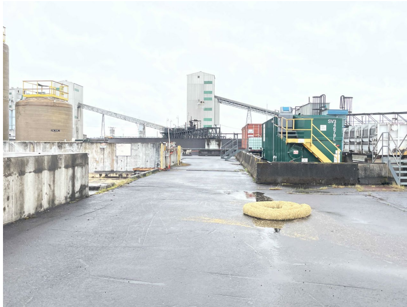
Envirocon installed stormwater inlet protection near Facility 71 (facing southeast).
