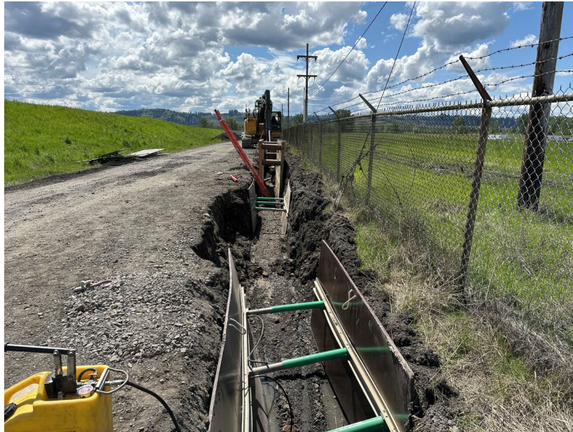
Catworks trenching for installation of east force main piping along Berth Road (facing southwest).
