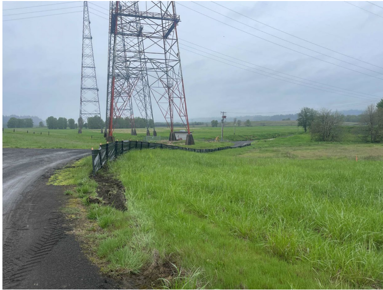
Envirocon installed silt fence along West Landfill perimeter (facing west).
