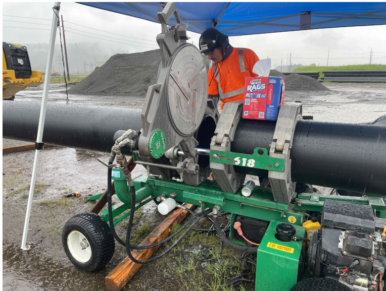
Fusing of east force main HDPE piping joints.
