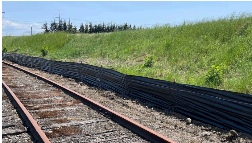
Envirocon installed silt fence around northern perimeter of East Landfill No. 2 (facing southeast).
