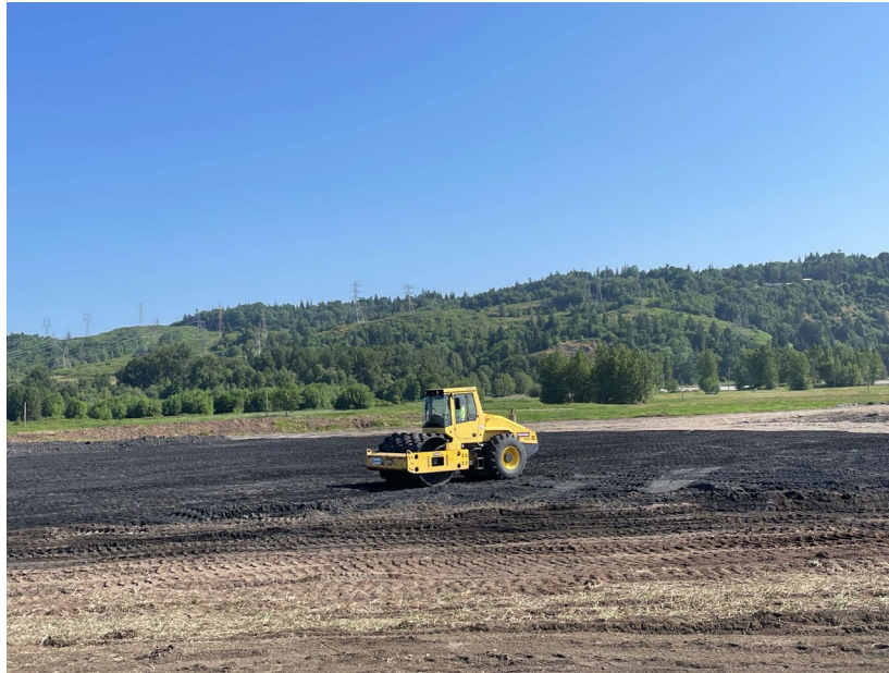
Envirocon roll compacting West Landfill (facing northeast).
