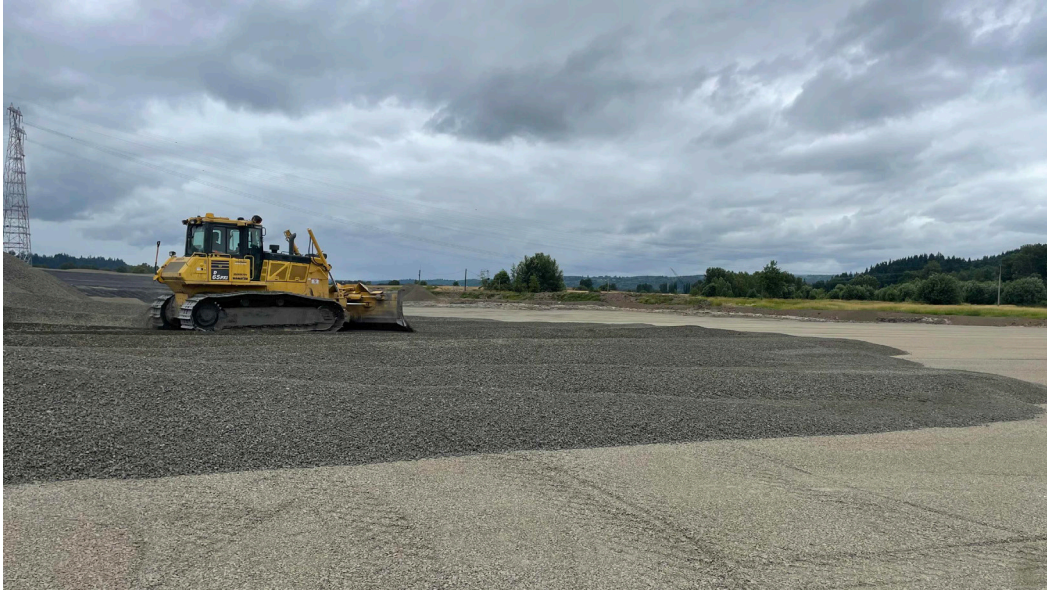
Envirocon placing select fill on top of reactive backfill in SU2 (facing east).
