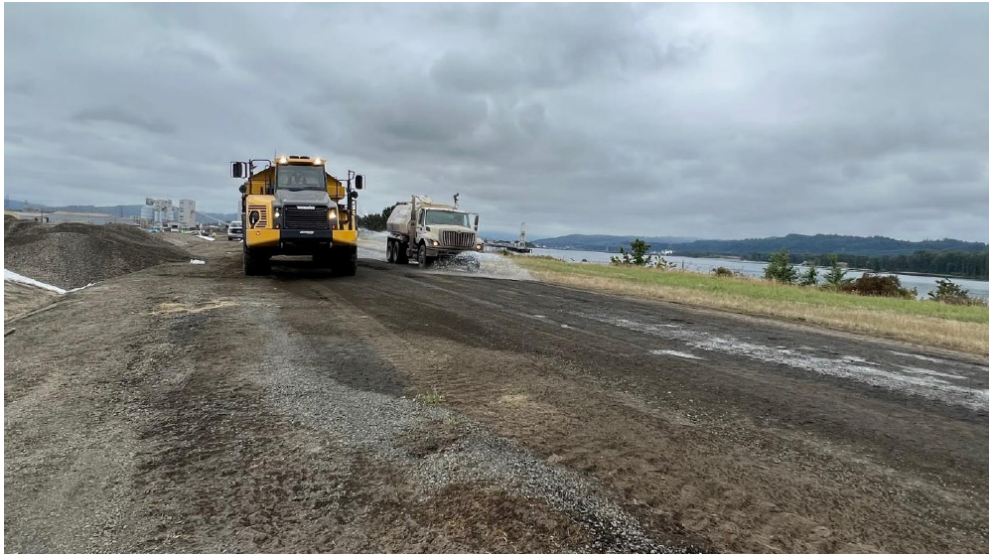
Envirocon, Inc., performing dust suppression control along Dike Road (facing southeast).
