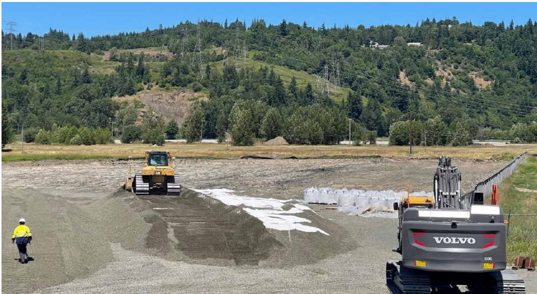
Photograph 12 West Landfill – Reactive Backfill Mixing
