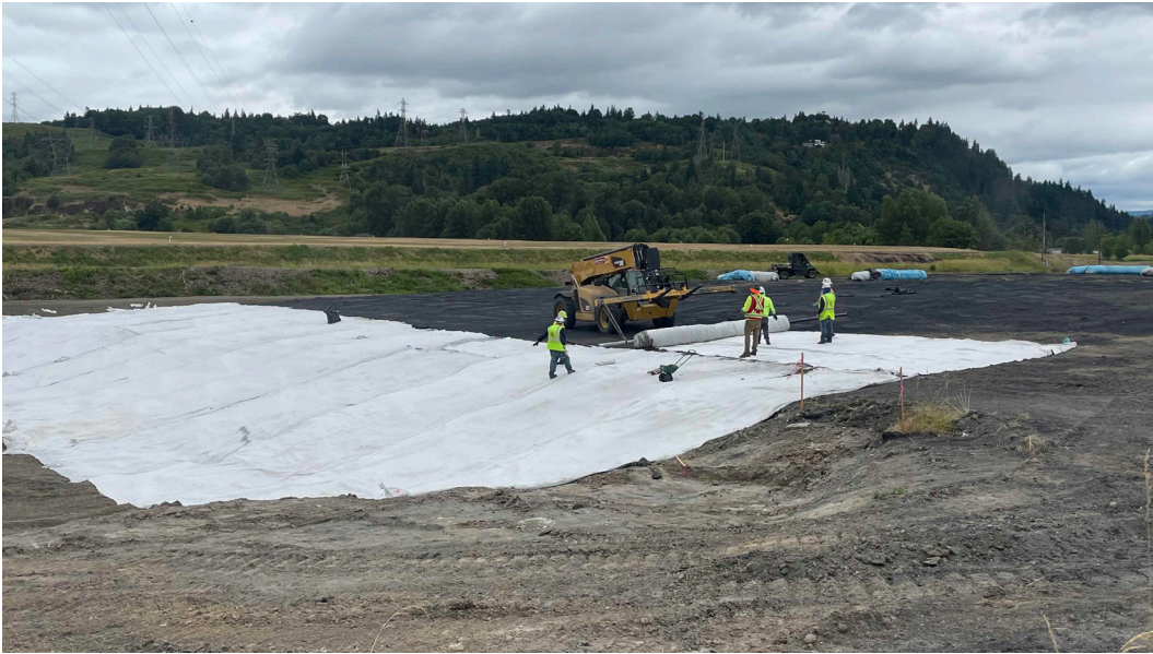
Northwest Linings & Geotextile Products, Inc., placing geotextile clay layer (GCL) membrane in West Landfill (facing northeast).
