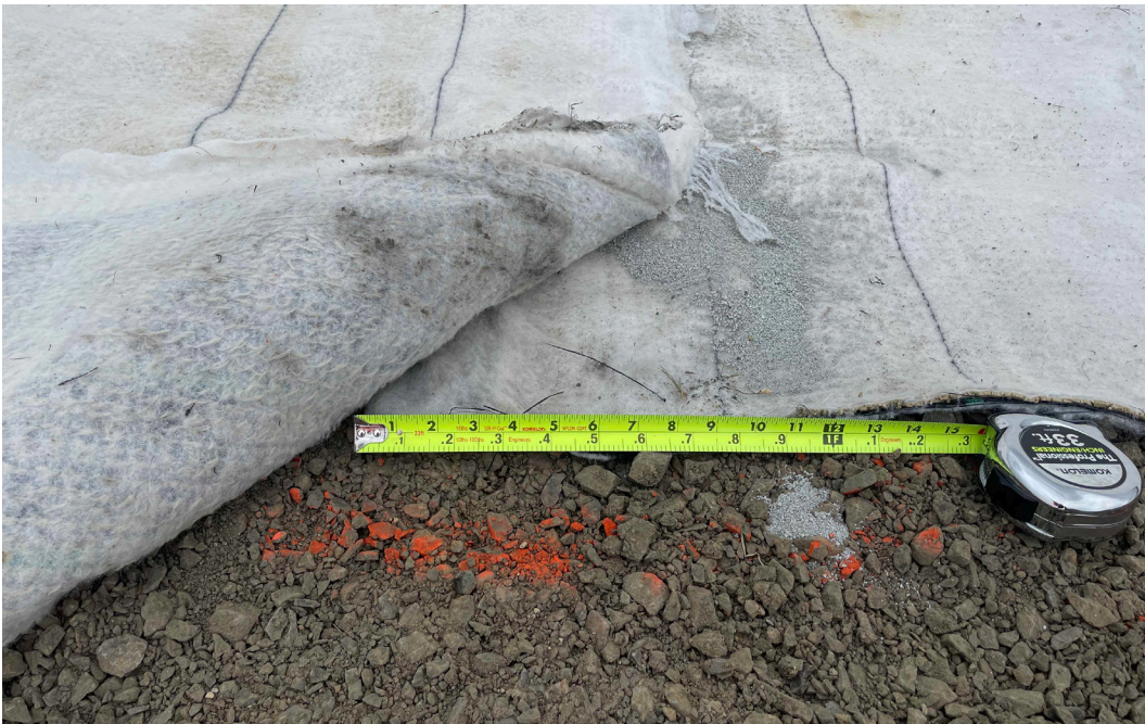
Granular bentonite used as a seal along the GCL 9-inch overlap seam.
