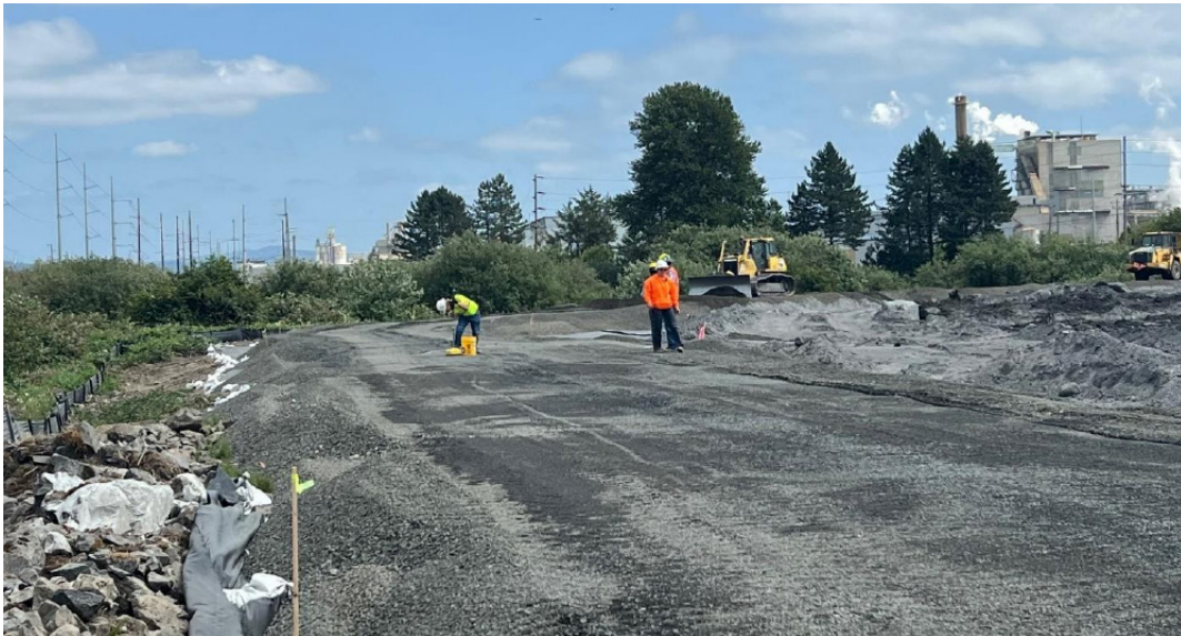
Professional Service Industries, Inc., performing compaction testing of Select Fill berm material (facing southeast).
