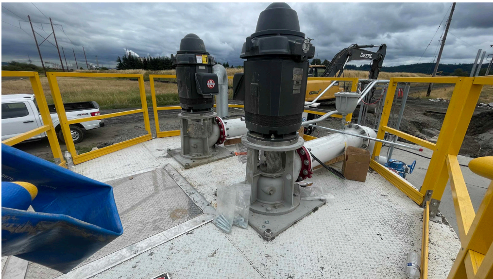
Catworks Construction installed a mechanical electrical pump at the East Force Main wet well (facing south).
