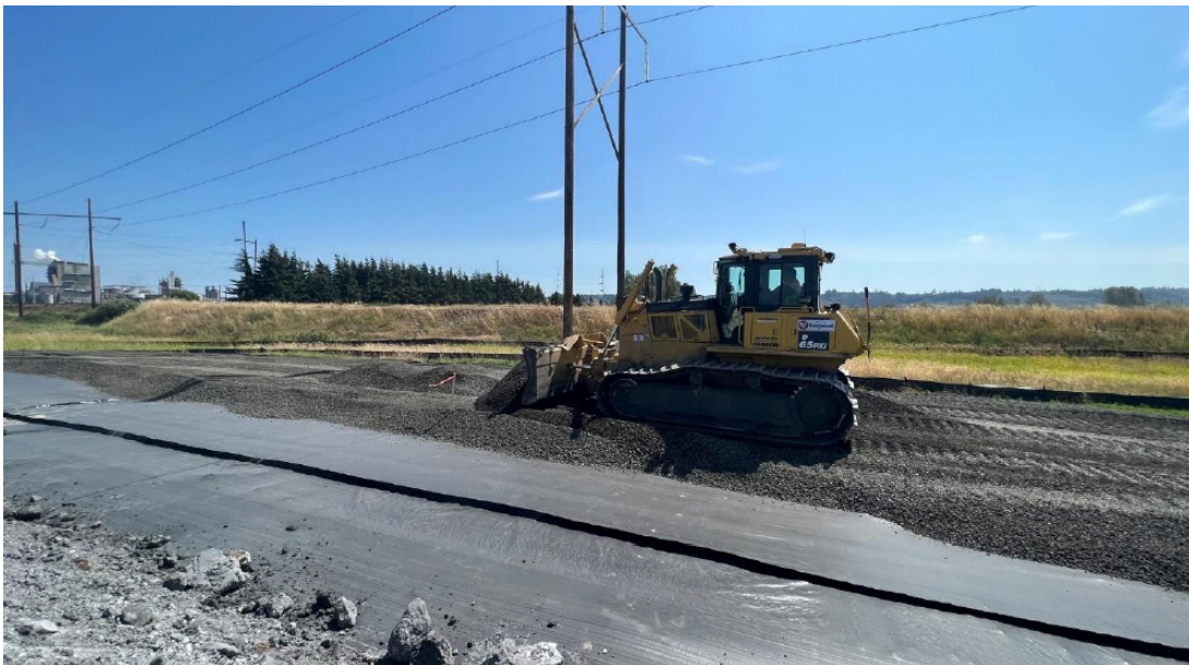
Envirocon installing Select Fill berm around the perimeter of East Landfill No. 1. Material was placed above geotextile fabric (facing east).
