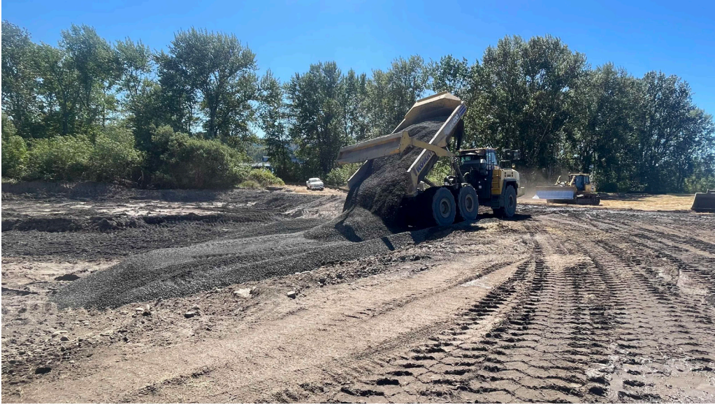
Envirocon backfilling the SU10 excavation with Select Fill (facing southeast).
