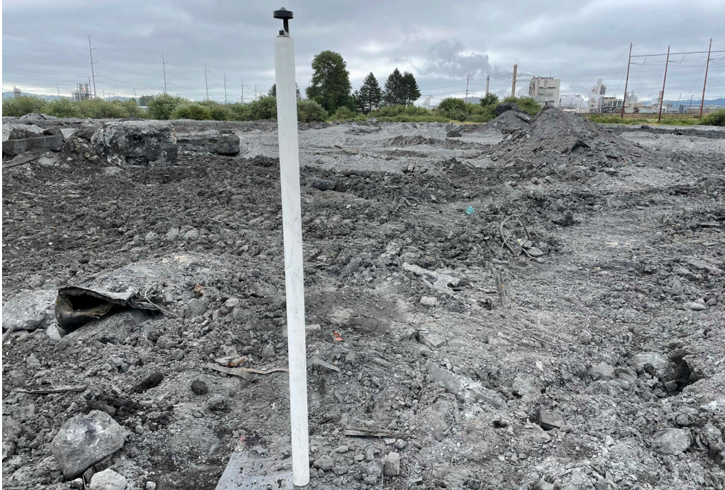
Photograph 11 East Landfill No. 1 – Settlement Plates
