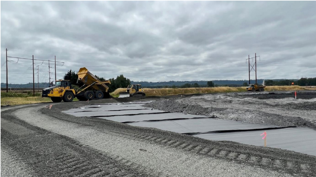
Envirocon installing Select Fill berm around perimeter of East Landfill No. 1. (Facing southwest).
