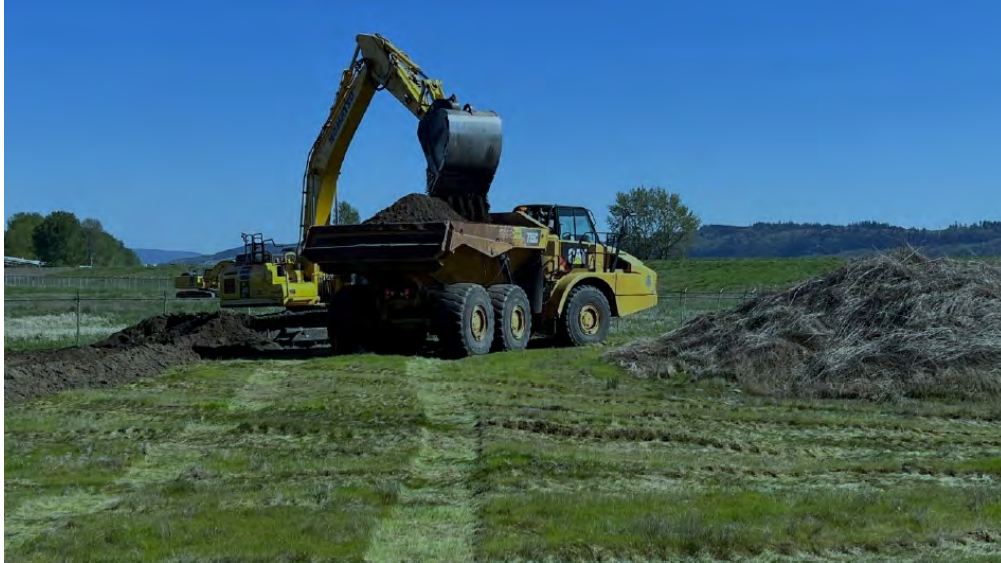
Photograph 11 Landfill (SU2) grubbing
