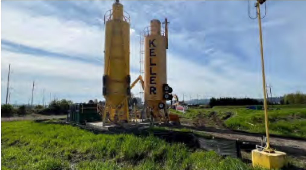
Photograph 1 Ground Stabilizing Subcontractor Setting Up Material at East Landfill No. 1
