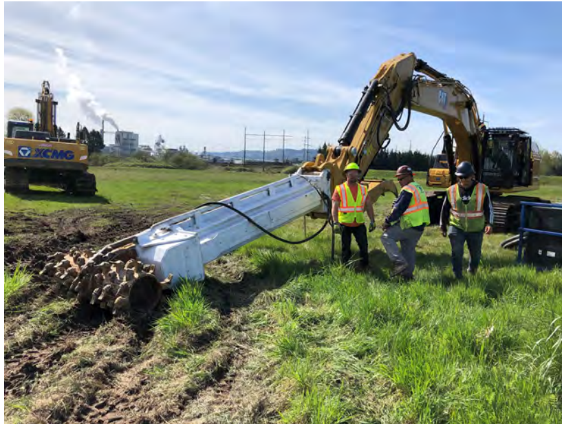
Photograph 6 East Landfill No. 1 Ground Improvement
