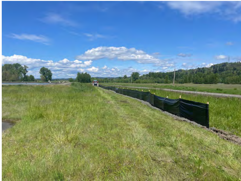
Photograph 4 U-Ditch silt fence installation.
