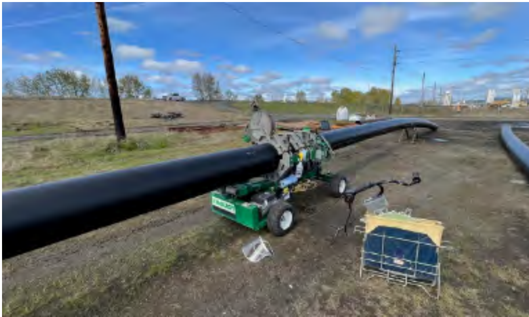
Photograph 2 East force main pipe fusion welding
