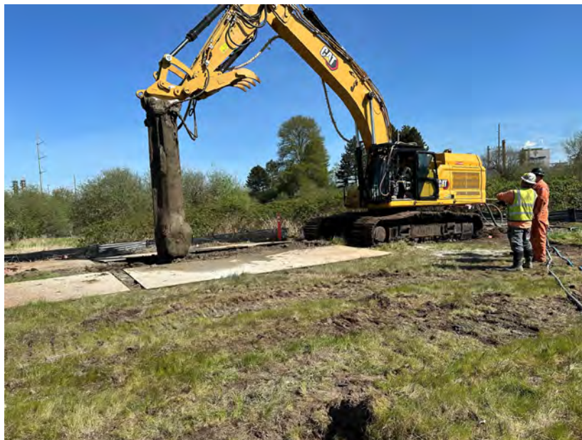
Photograph 7 East Landfill No. 1 Ground Improvement
