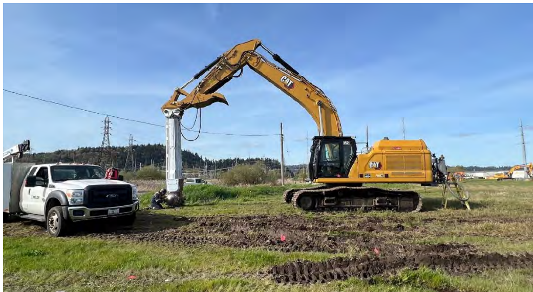
Photograph 5 East Landfill No. 1 Ground Improvement
