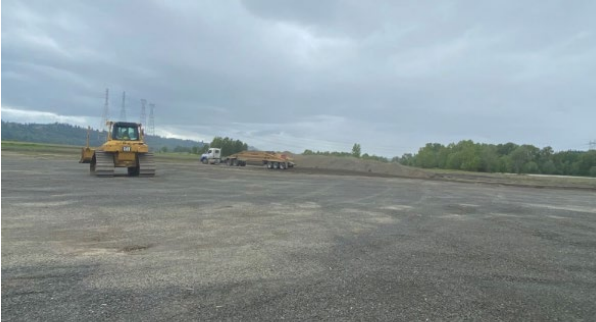
Delivery and maintenance of import select fill at East Staging Area
