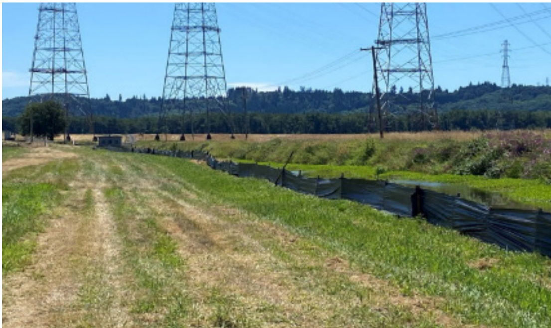
Silt fence installation along segment 1 (looking south)
