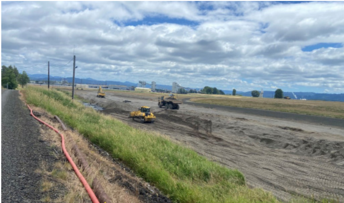
Placement and grading of general fill
