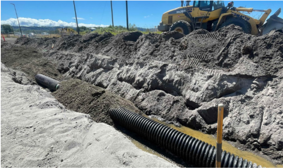
Installation of 12-inch CPE pipe along Berth Road
