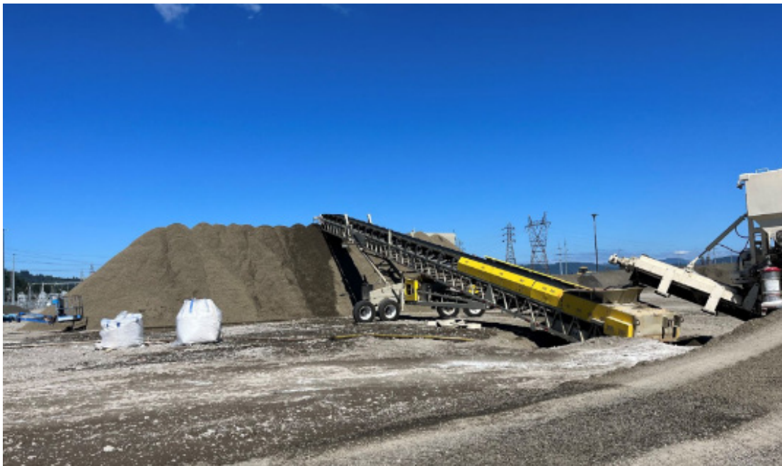
Mixing 3.4% dosage reactive backfill for use in SU3
