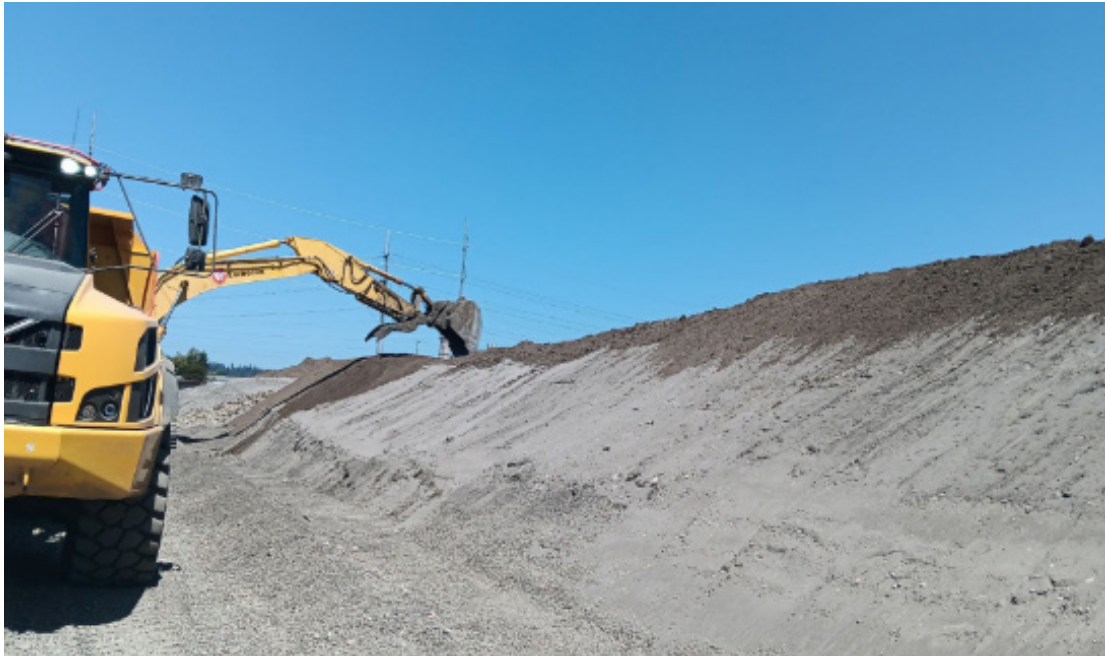
Topsoil placement along western slope
