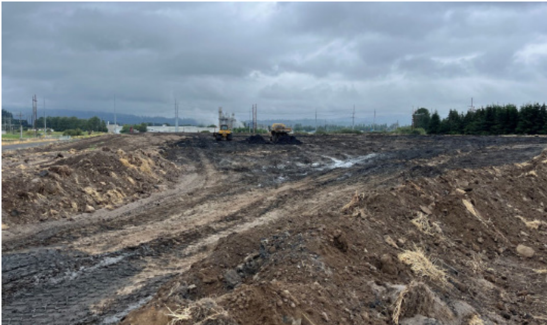
Grading and consolidation of waste material removed from SU3
