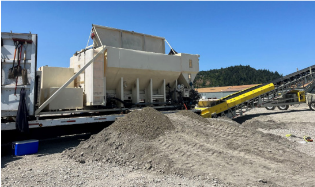
Mixer and conveyer mobilization and startup
