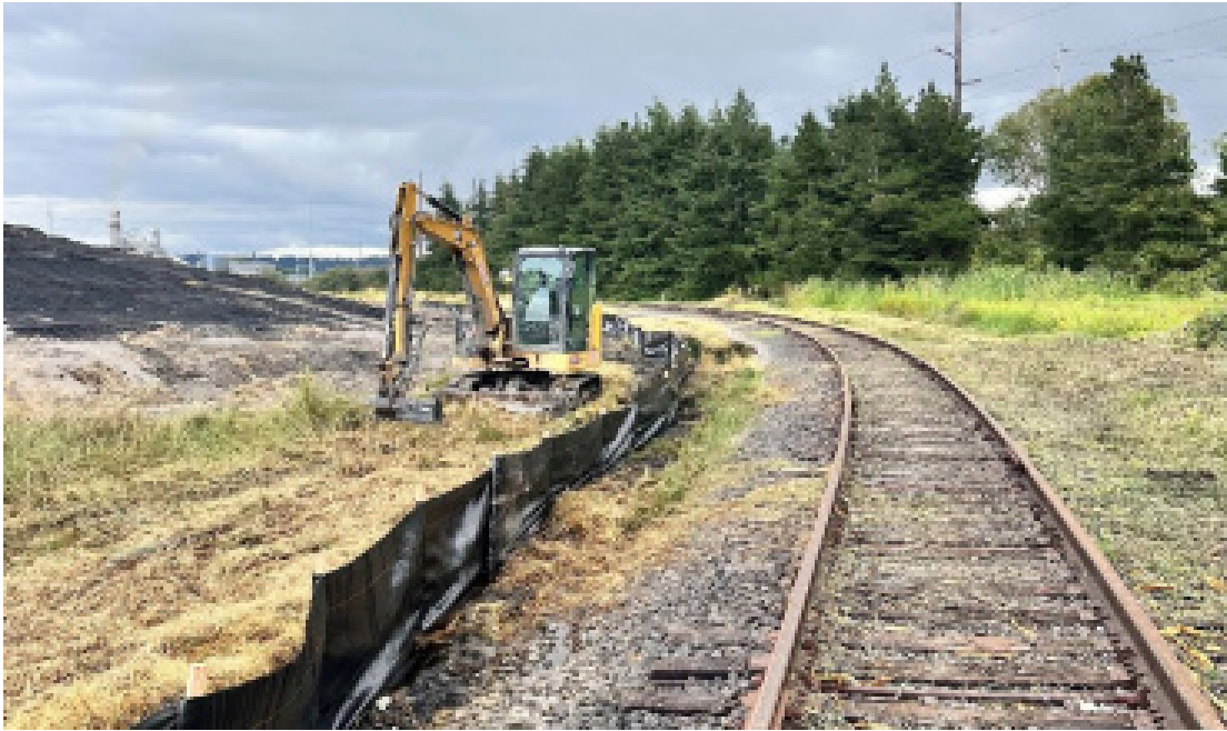
Silt fence installation along toe of southern slope
