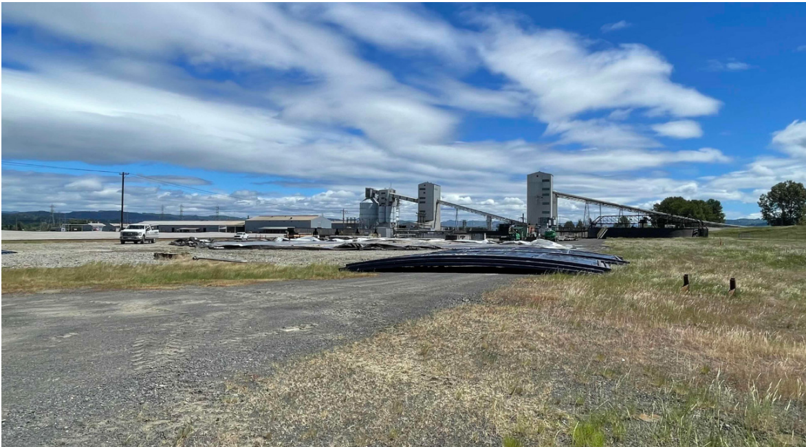
Deinstallation of 1-million-gallon extension tank
