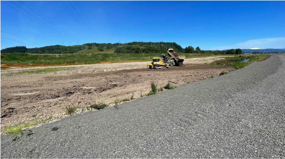
Start of final regrading
