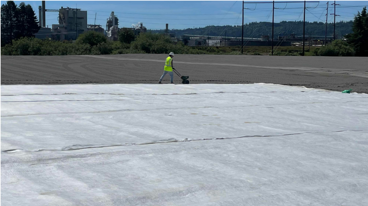
Placement of granular bentonite at GCL seams
