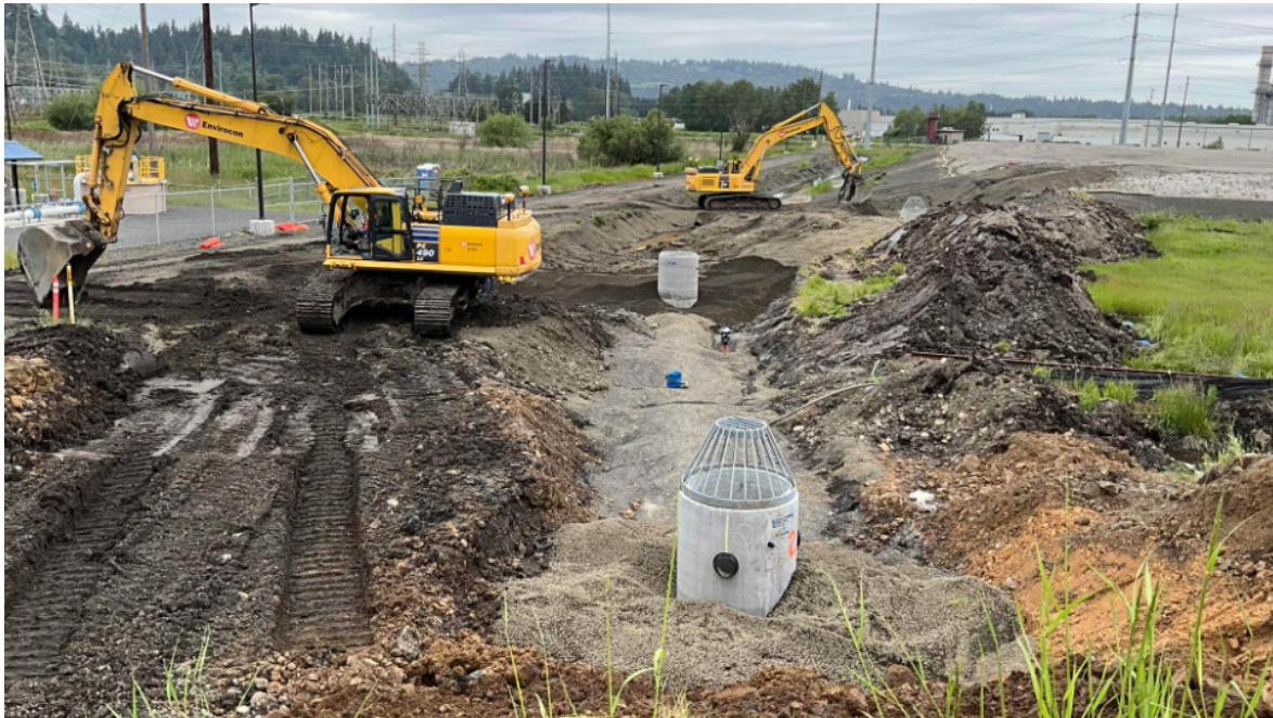
Placement of select fill over 24-inch CPE pipe
