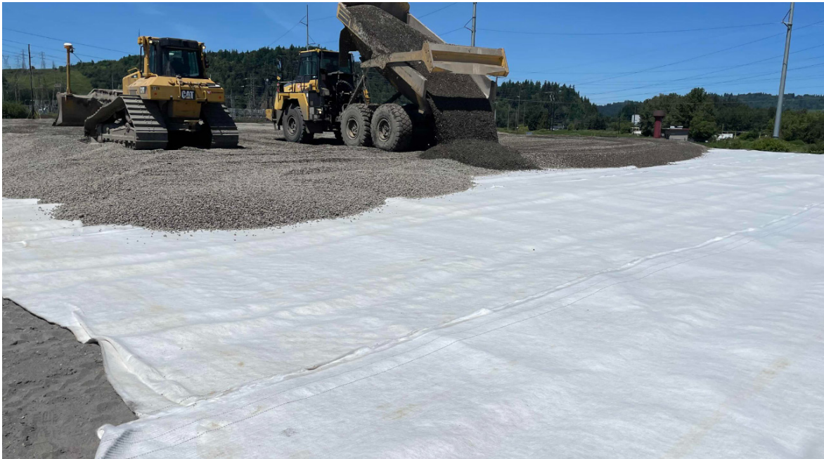
Placement and distribution of drainage layer material over GCL
