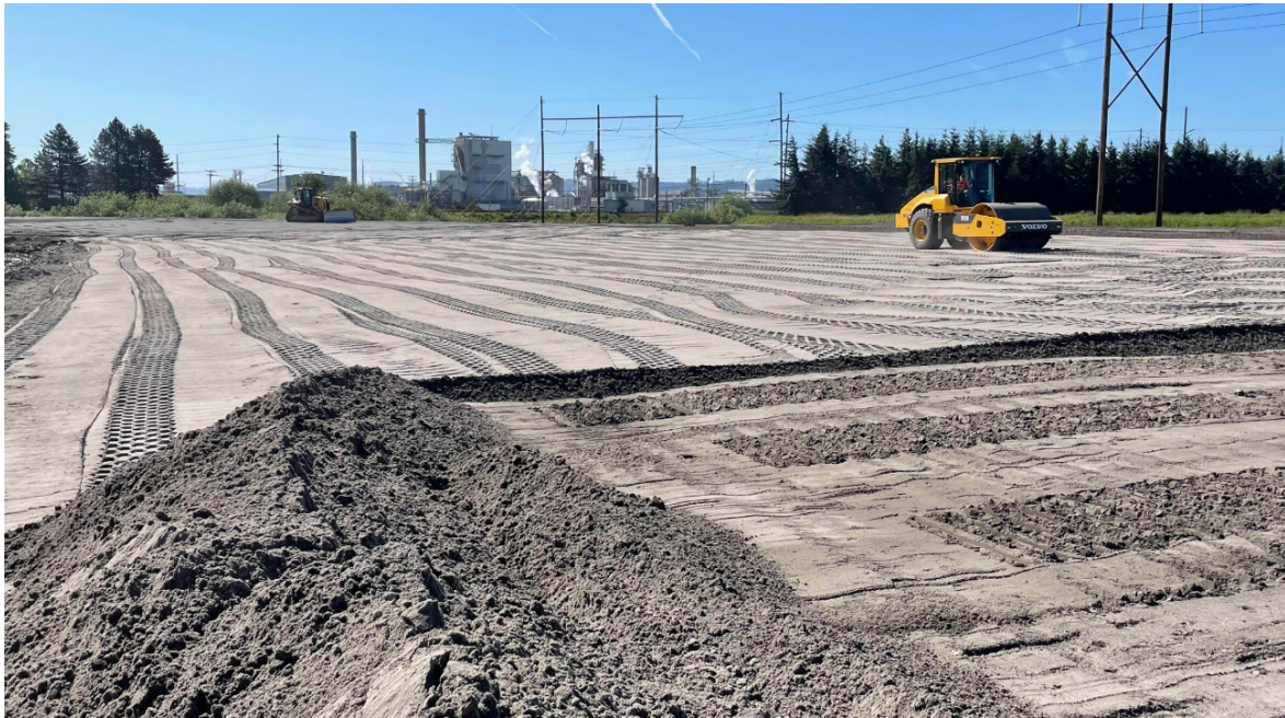
Proof-rolling general fill final grade
