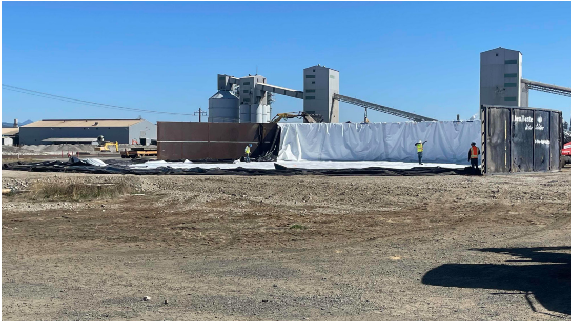
Denbeste Water Solutions installing 1-million-gallon water tank extension at Facility 77.
