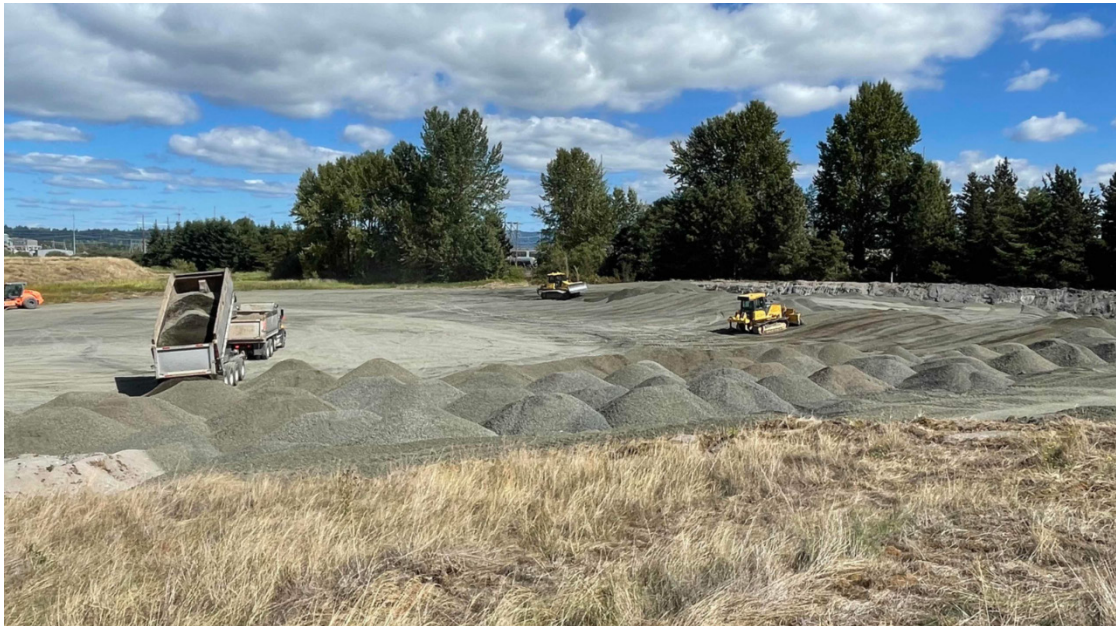
Delivery, placement, and compaction of select fill in SU8.
