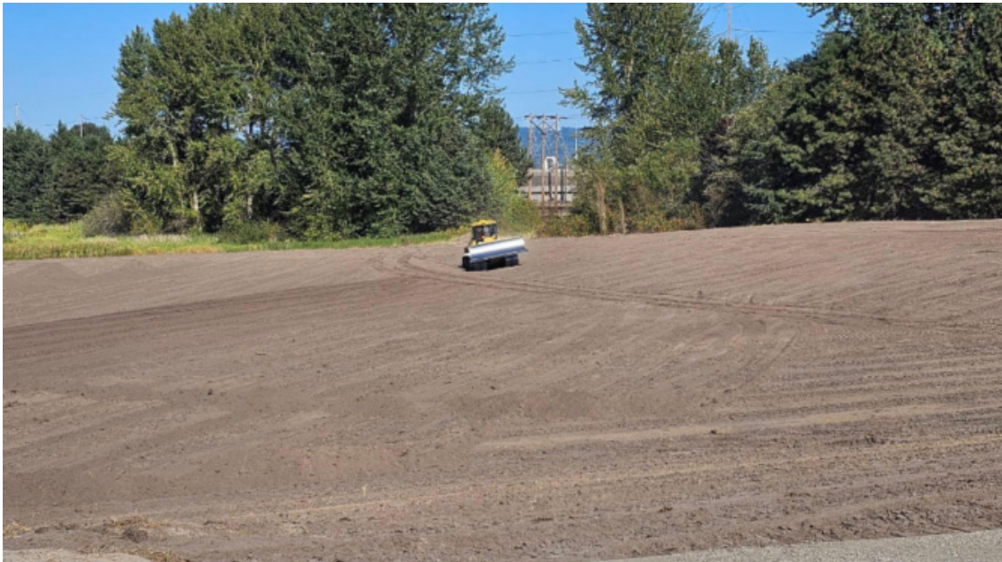
Envirocon, Inc., placing general fill above geotextile fabric at SU8 (facing east).
