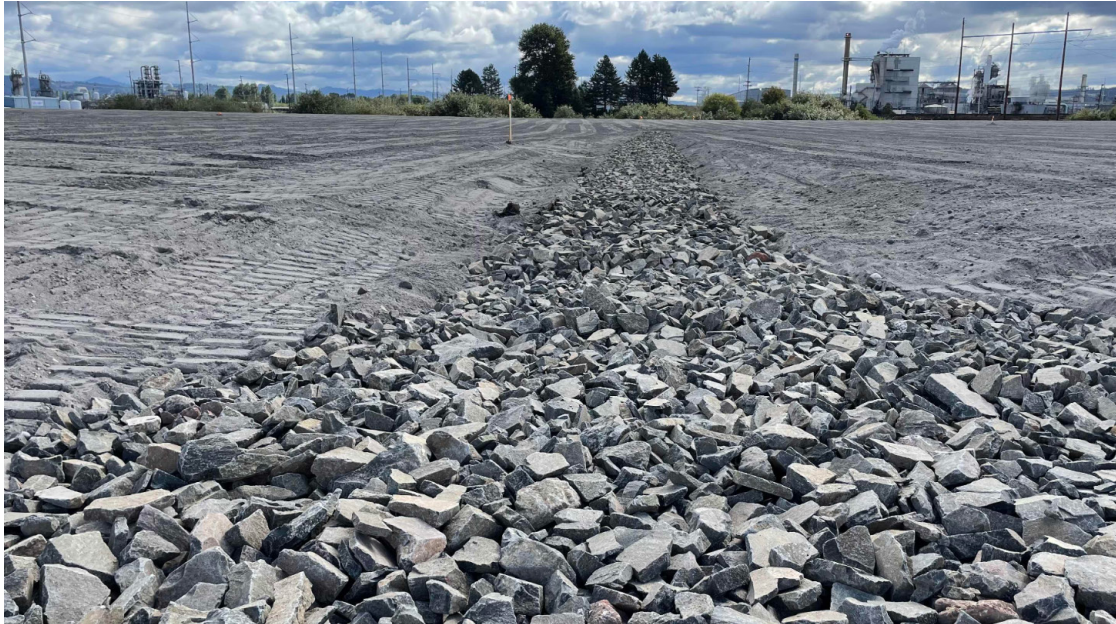
Construction of Season 1 drainage channel in East Landfill No. 1.
