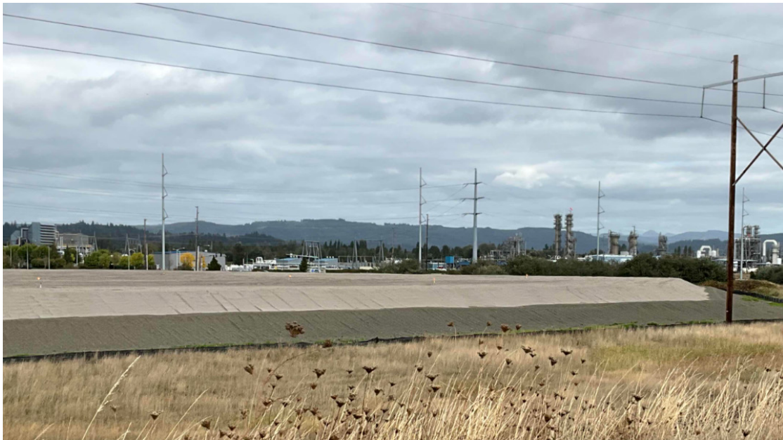
Placement of general fill over compacted, consolidated waste material in East Landfill No. 1.
