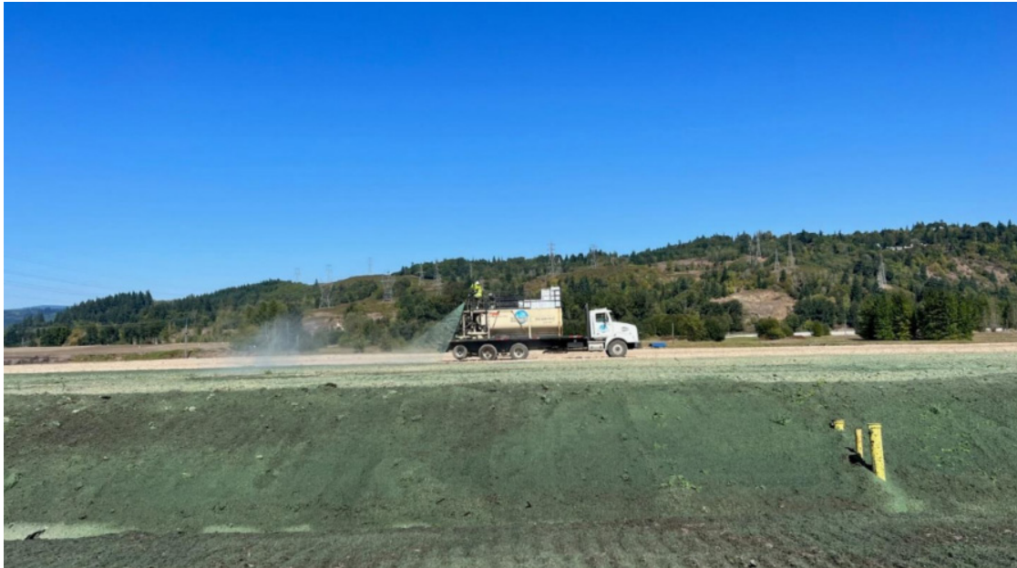
Application of Hydroseed Mix No. 2 over topsoil in West Landfill.
