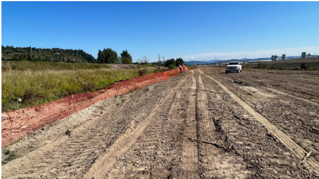
Installation of temporary construction fence along southern edge of U-Ditch.
