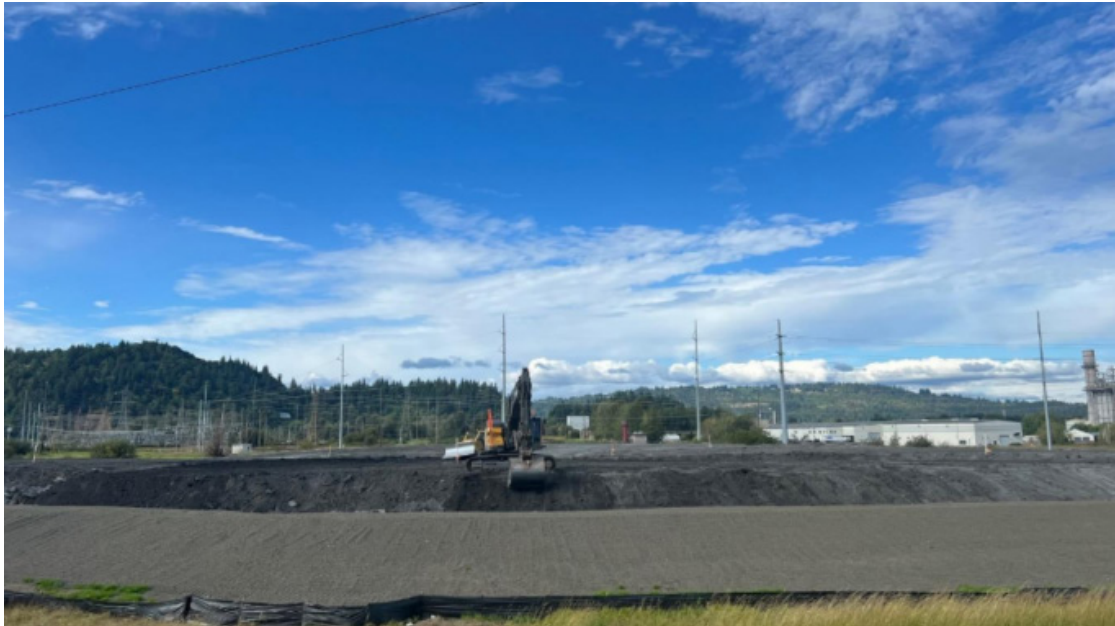
Final grading of consolidated waste material in East Landfill No. 1.
