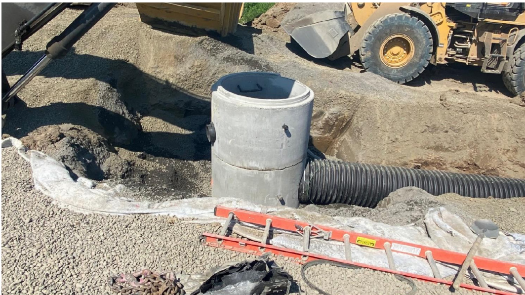
Installation of 48-inch-diameter concrete manhole with 24-inch-diameter corrugated polyethylene pipe.
