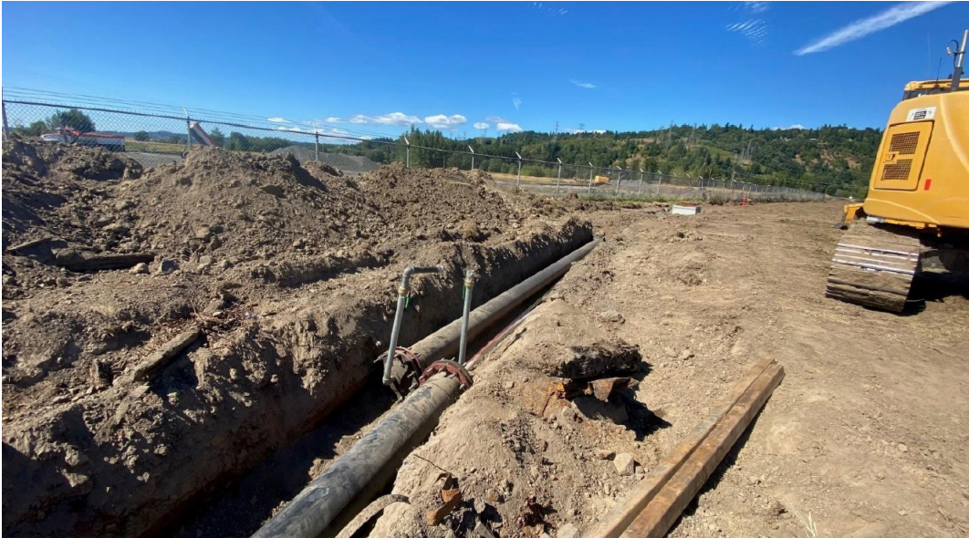
Installation of 14-inch flange valves in preparation for hydrostatic pressure test.
