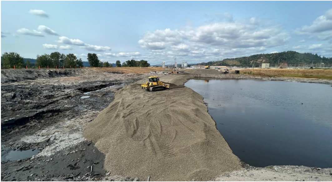
Envirocon backfilling at SU8 (facing northwest).
