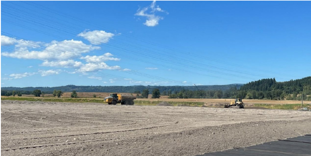
Envirocon placing general fill above geotextile fabric at West Landfill (facing north).
