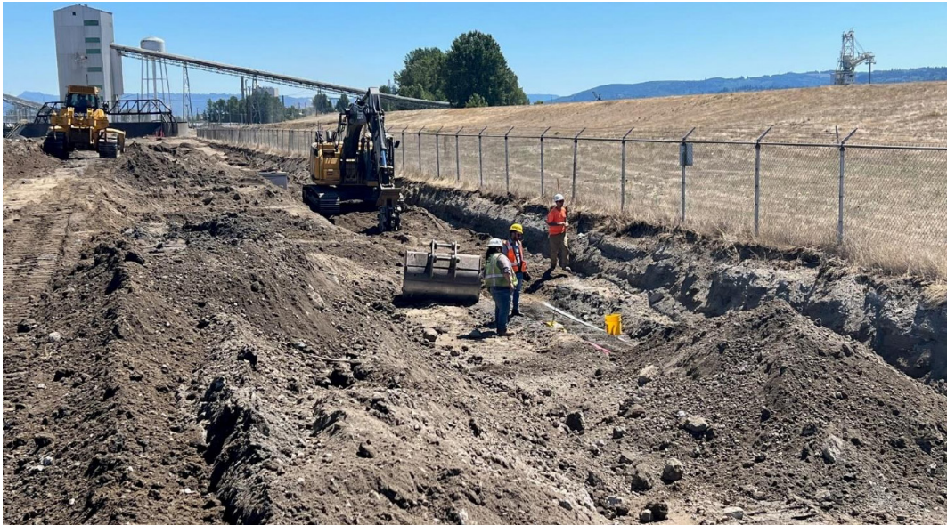
Compaction testing being performed along west force main backfill material (facing southeast).
