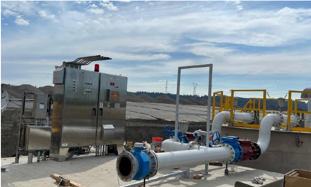
Installation of mechanical, electrical, and plumbing at West Pump Station.
