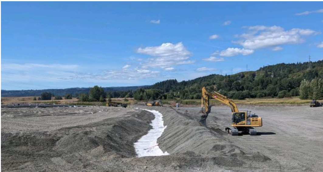
Envirocon constructing berm along the eastern area of the West Landfill. Geosynthetic clay layer was placed in drainage ditch (facing northwest).
