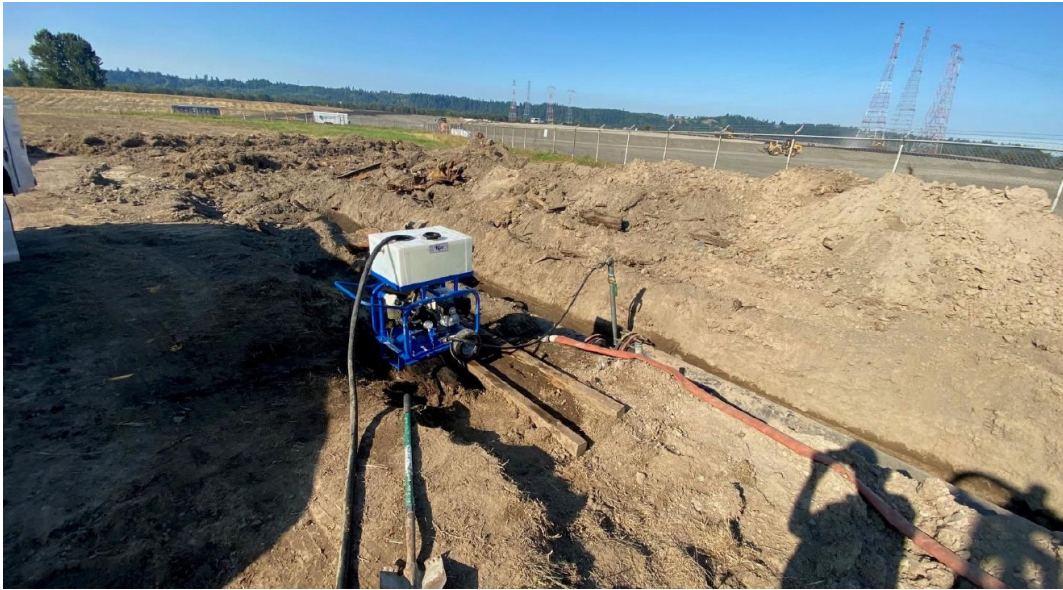
Hydrostatic pressure test being performed on west force main piping (facing southwest).
