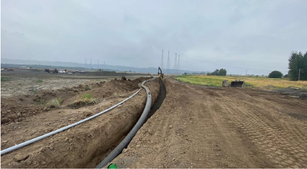
Installation of 14-inch-diameter high density polyethylene (HDPE) west force main piping (facing west).
