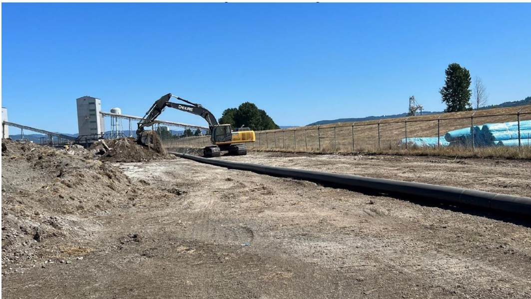
Catworks trenching along west force main alignment (facing south).
