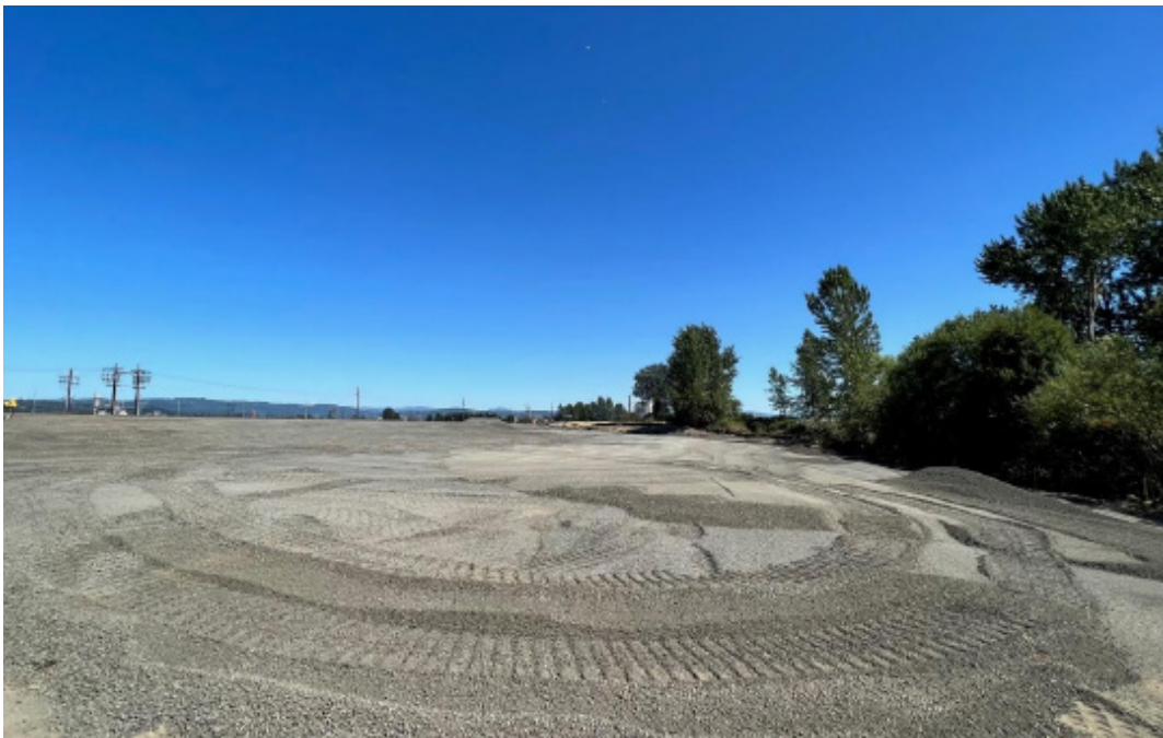
Backfill and compaction completed at SU10 (facing northeast).
