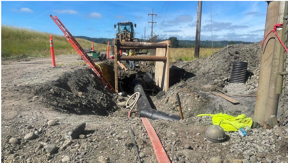
Photograph 4 East Force Main – HDPE Pipe Fusing
