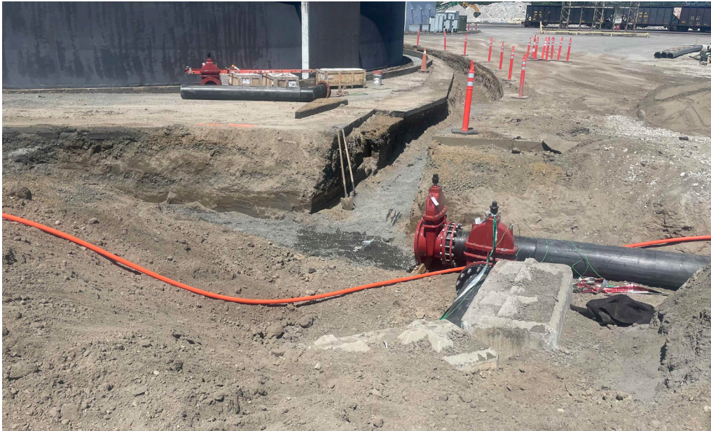
East Force Main piping being installed with gate valve near STA 236+51 (facing north).
