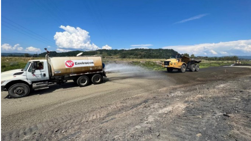
Envirocon, Inc., performing dust suppression control near U-Ditch (facing east).
