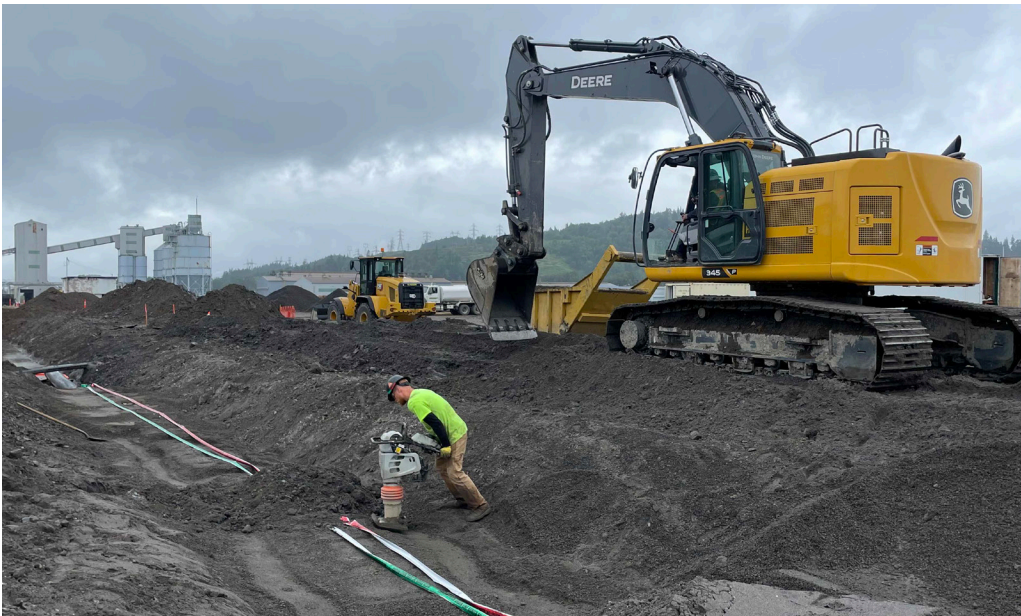
Envirocon performing compaction along East Force Main piping alignment (facing north).
