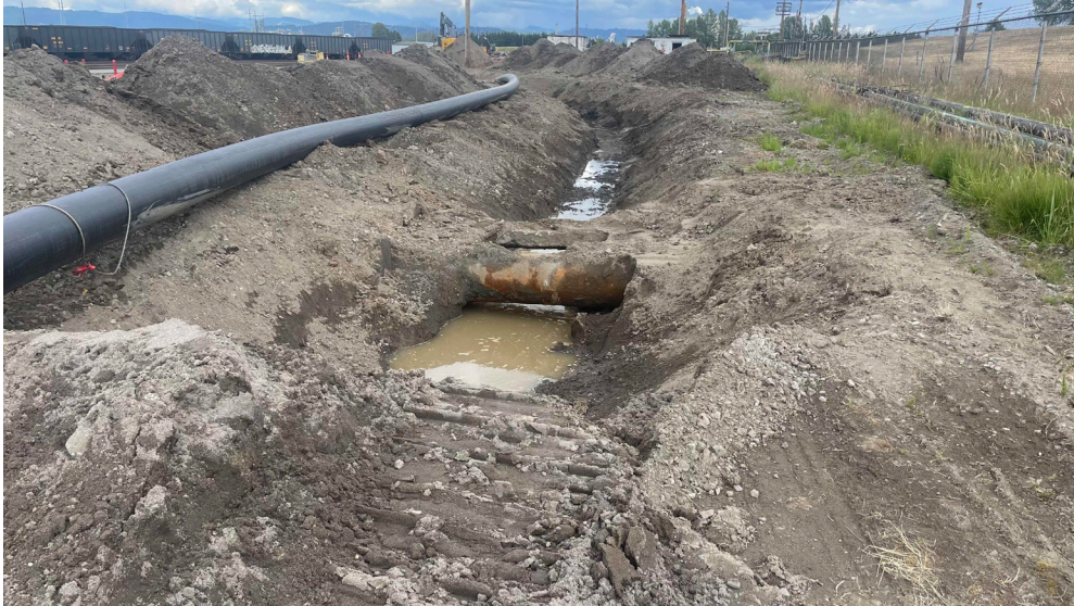
Trenching for East Force Main pipe installation near Outfall 001S (facing southeast).
