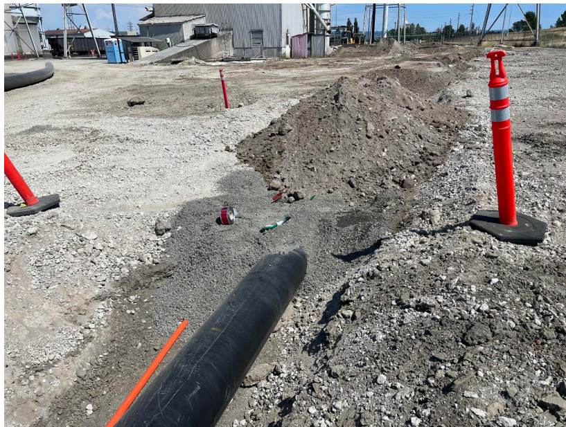
Envirocon installing 16-inch-diameter HDPE East Force Main piping approaching Facility 77. Note orange tracer line (facing east).
