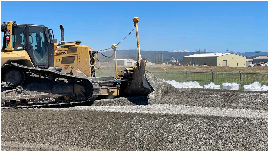
Photograph 14 West Landfill – Reactive Backfill Placement and Mixing
