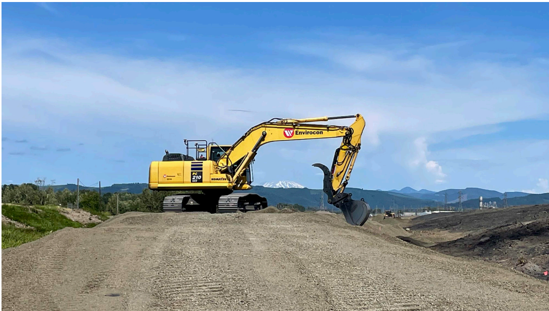
Envirocon constructing berm along the south side of the U-Ditch (facing southeast).
