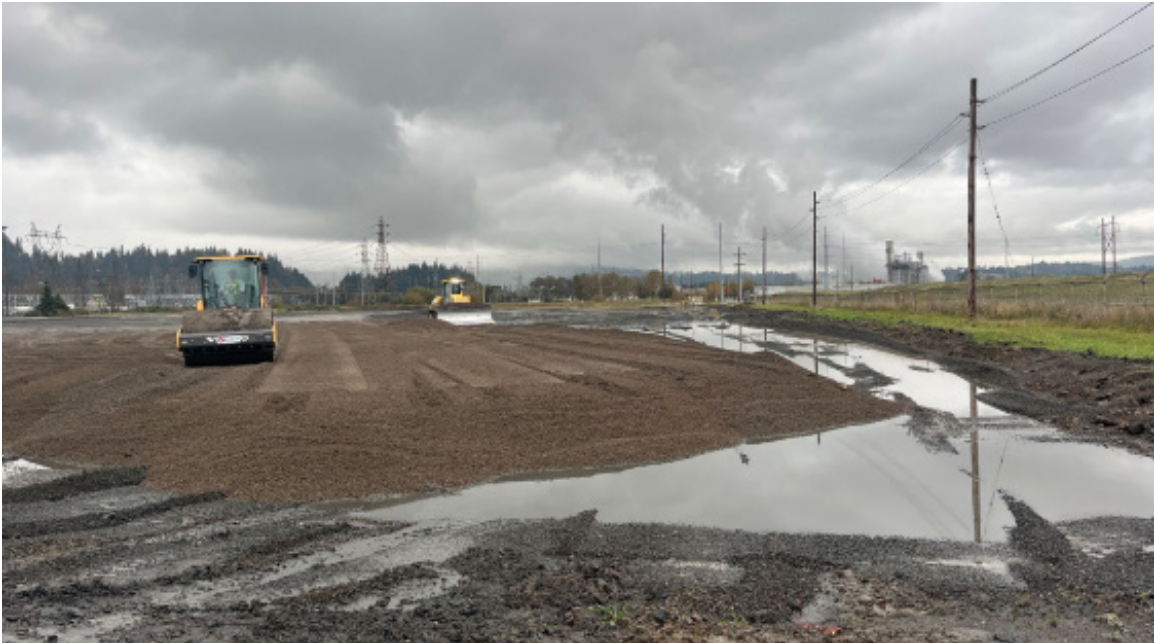
Placement and compaction of select fill
