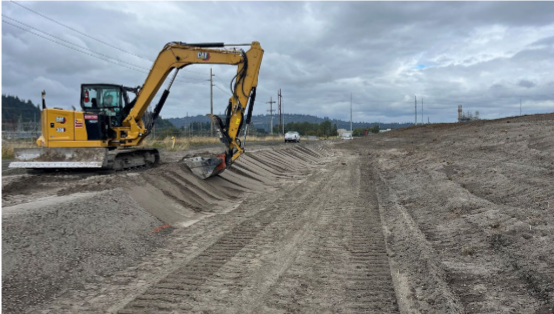
Grading west perimeter ditch
