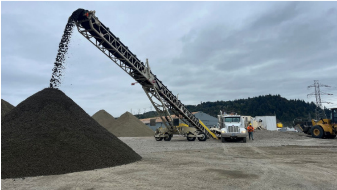
Mixing reactive backfill
