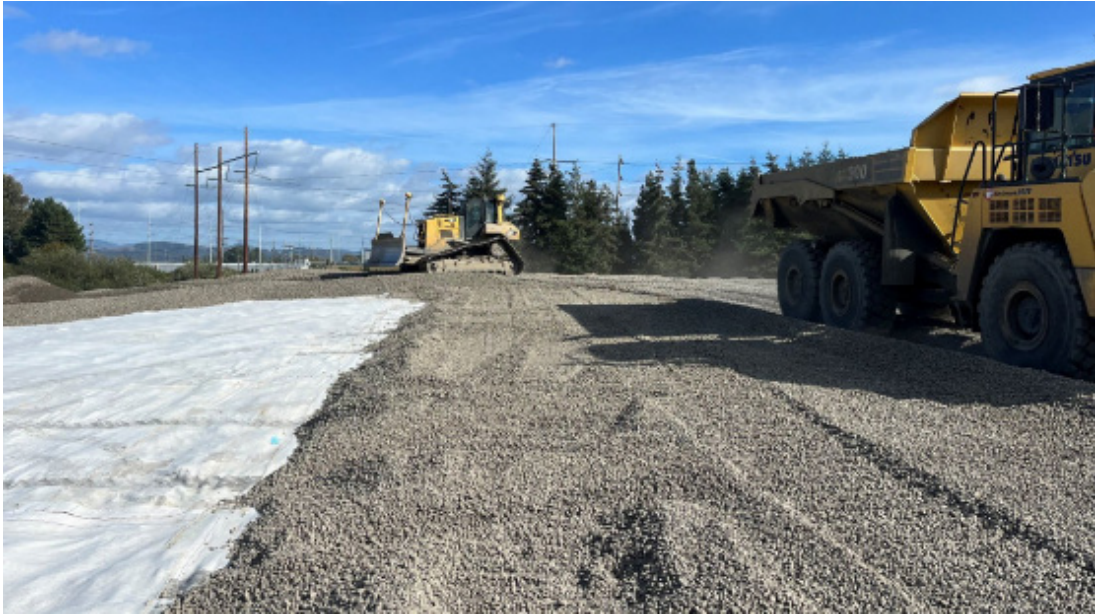
Placement of drainage layer material over GCL
