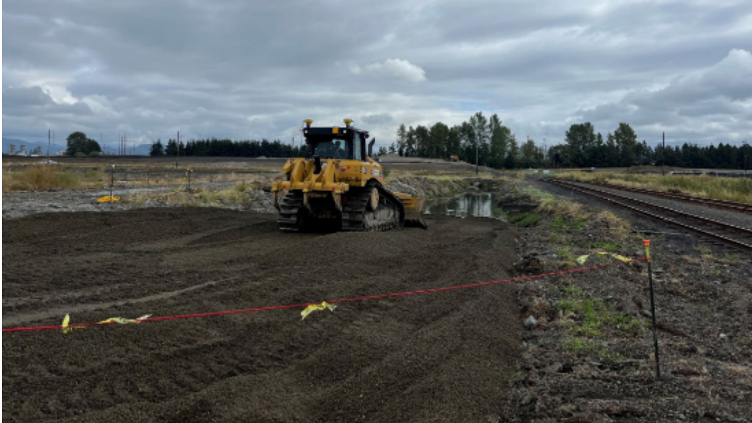
Reactive backfill placement
