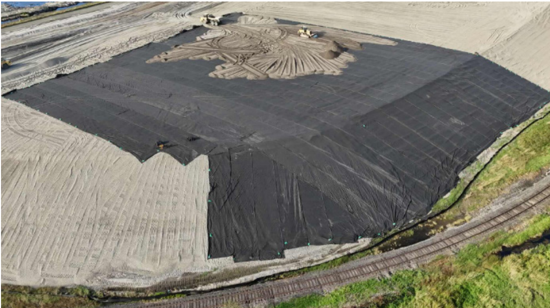
Non-woven geotextile deployment and placement of general fill
