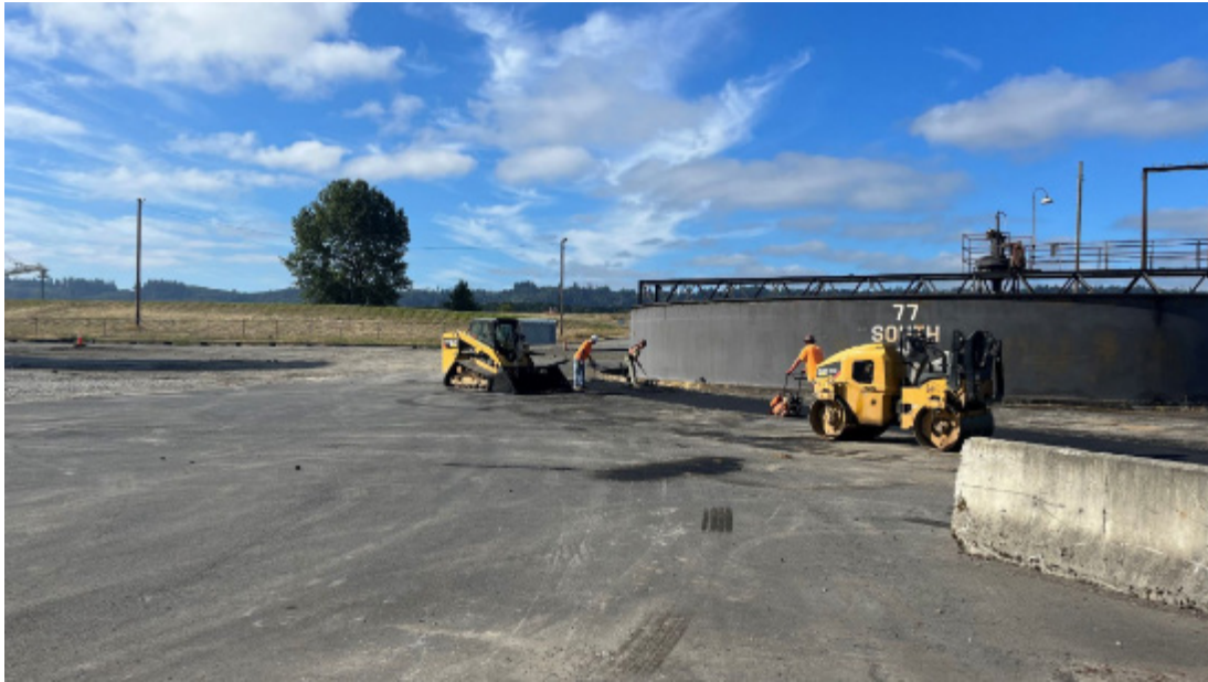
Asphalt placement over force main alignment
