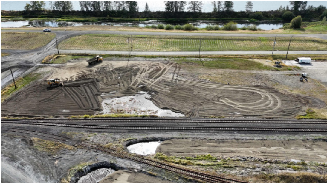
Reactive backfill placement
