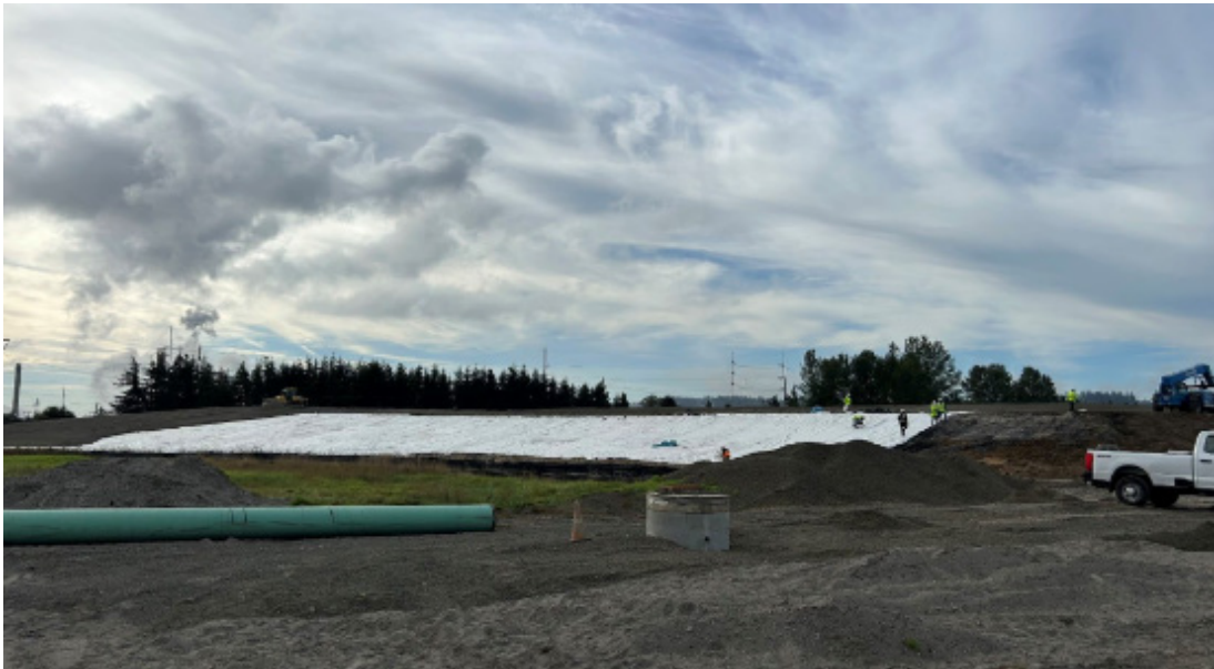
GCL deployment along northwestern slope
