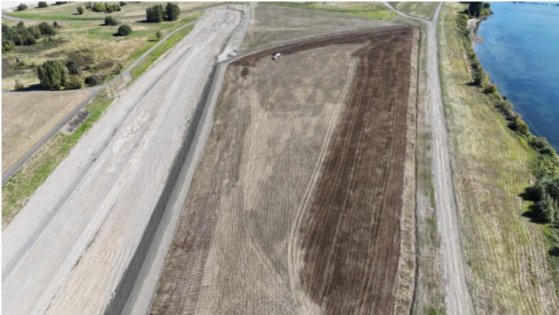
Hydraulic topsoil application
