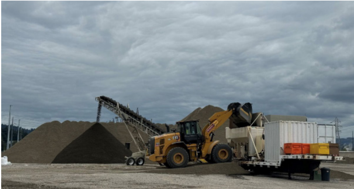
Mixing SU3 reactive backfill
