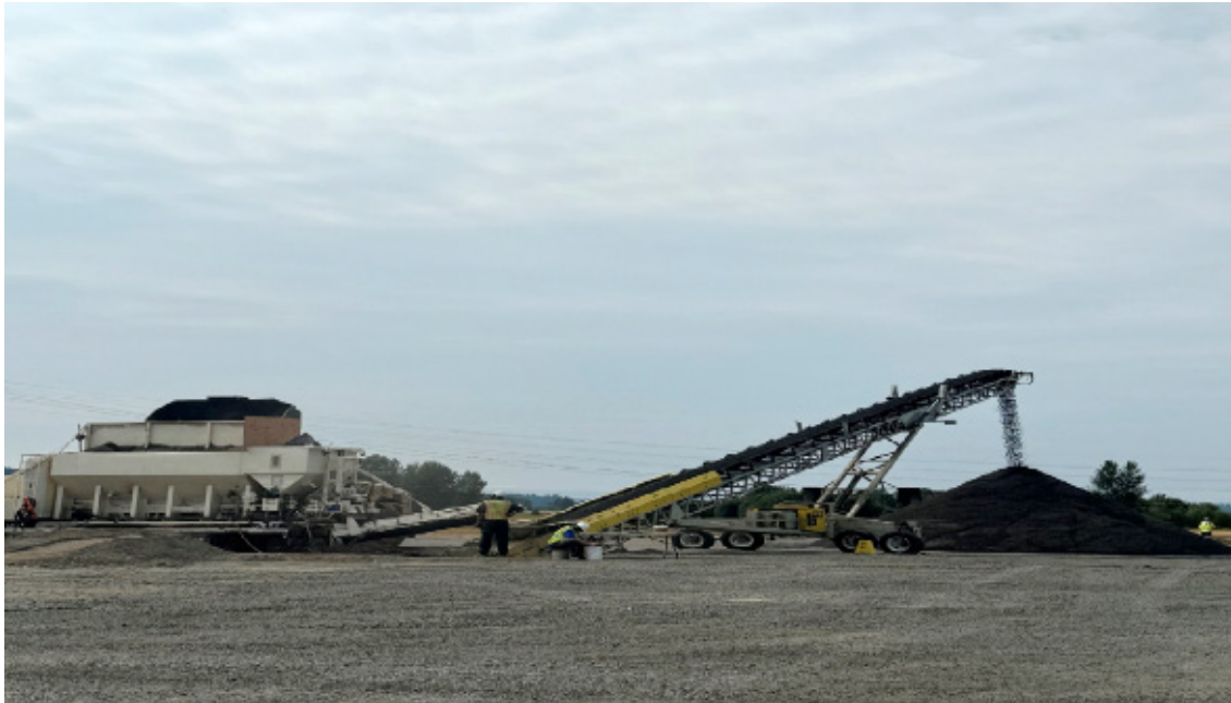
Pre-mixing coarse sand and pea gravel for the PRB
