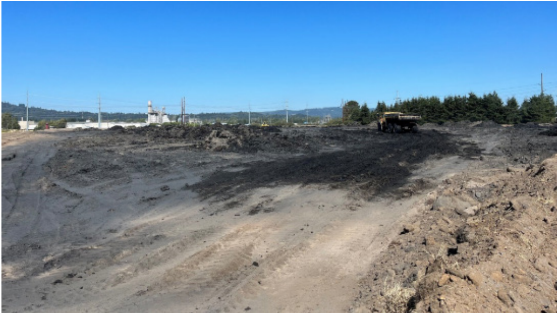
Consolidation of waste material excavated from SU3 and SU5 into East Landfill No. 2
