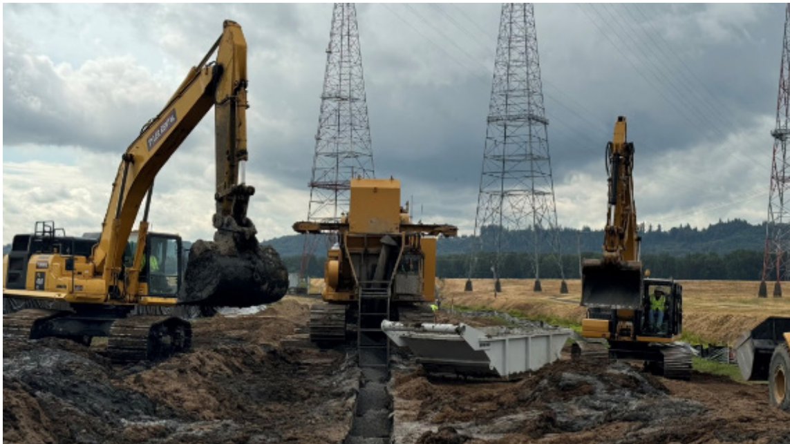
One-pass trenching installation – segment 1
