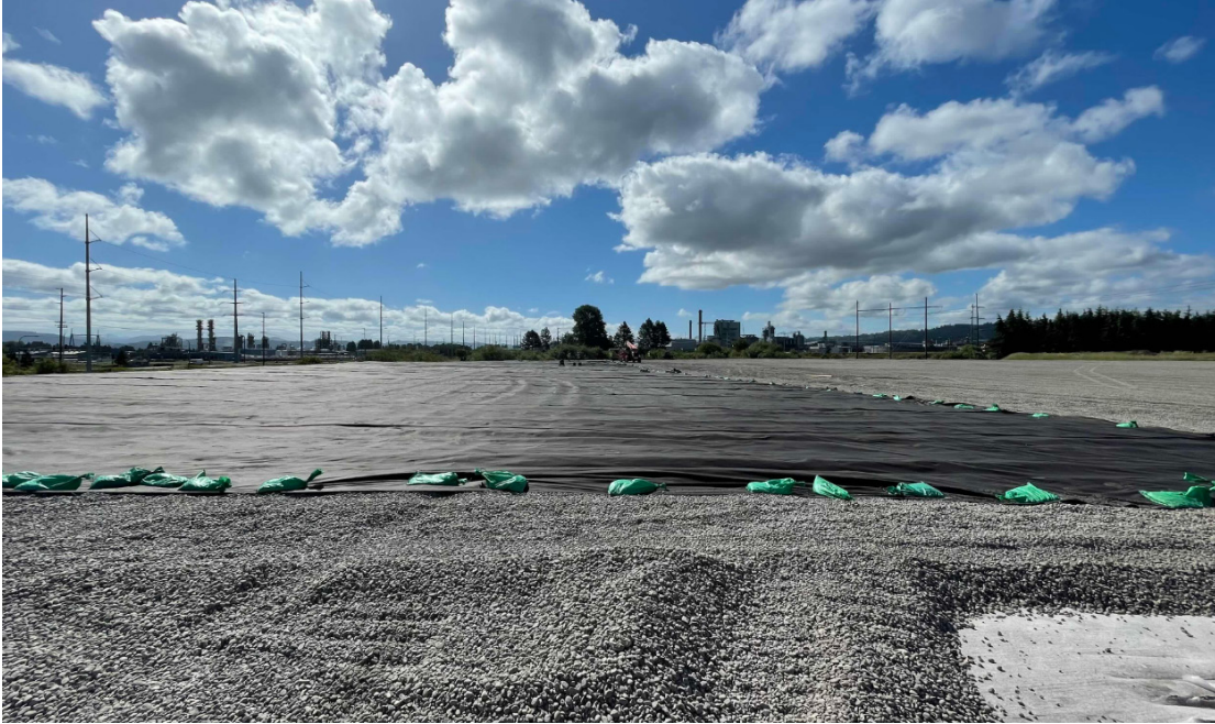
Deployment of non-woven geotextile over drainage layer material
