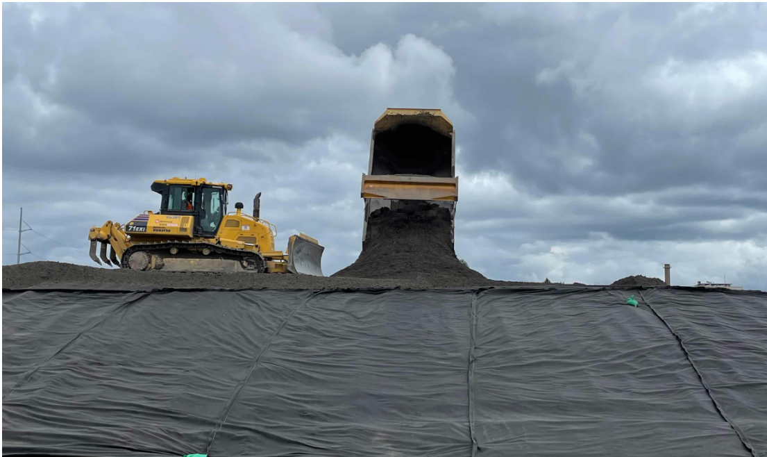
Placement and distribution of general fill over non-woven geotextile
