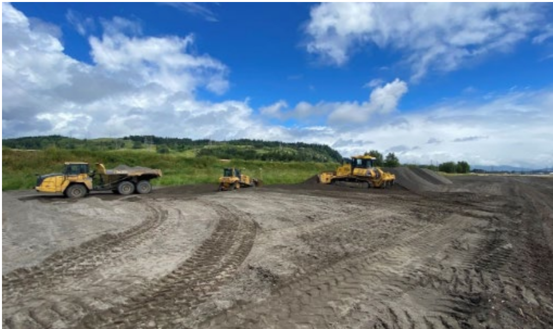
Backfill with general fill to design elevations within northern flow channel
