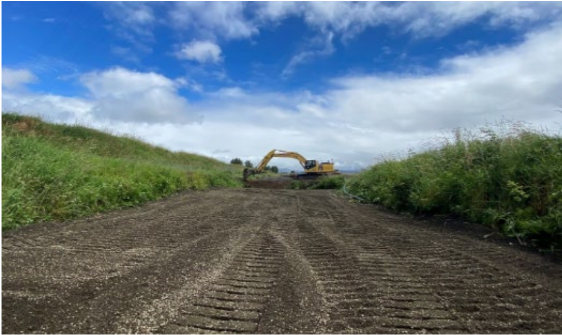
Backfill with select fill within ditch west of Outfall 006 reroute discharge line
