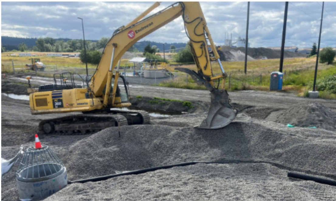
Berth Road perimeter ditch and 6-inch slotted drainage pipe
