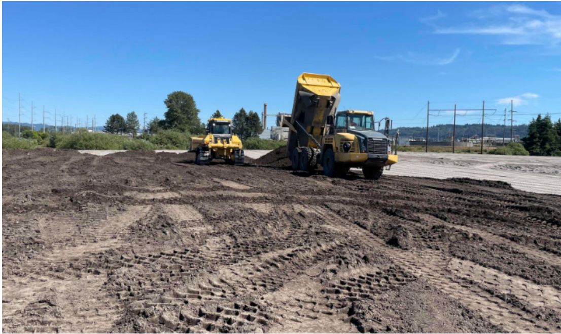
Placement and distribution of topsoil over general fill
