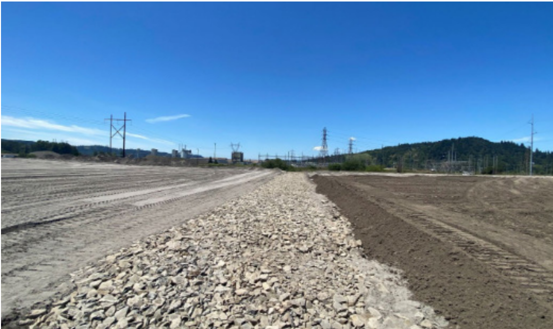
Quarry spalls within on-landfill stormwater conveyance channel
