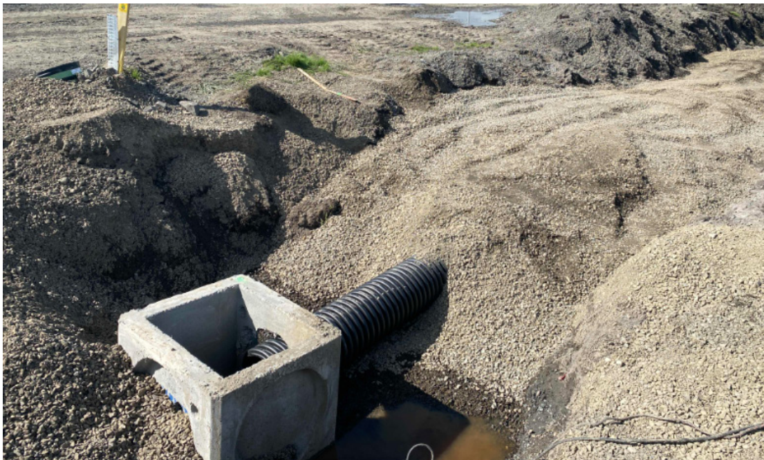
Installation of Type I catch basin and 12-inch CPE pipe
