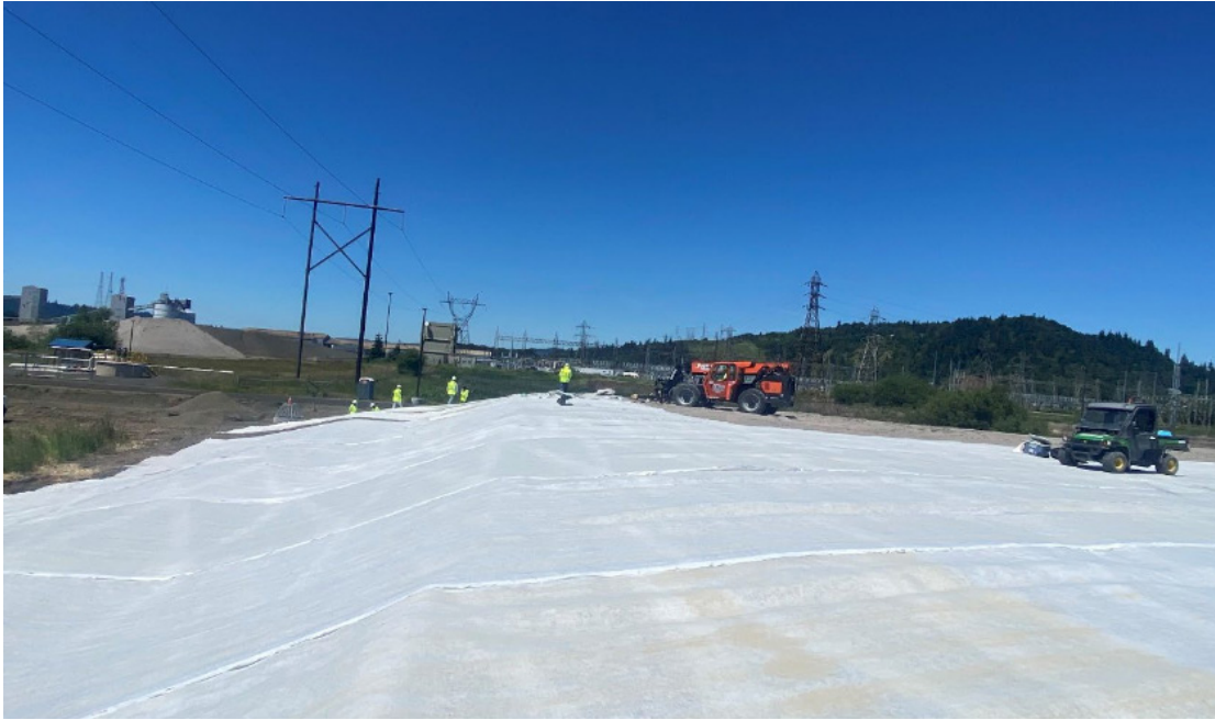
GCL deployment along southern slope
