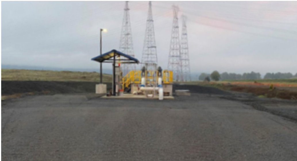
Final grading of gravel pad surrounding West Pump Station.
