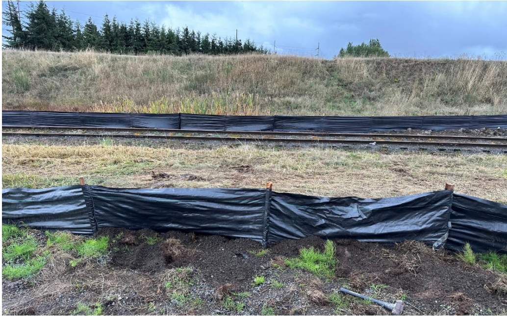
Repair of silt fencing along southern edge of East Landfill No. 1 (Site Unit [SU] 7).
