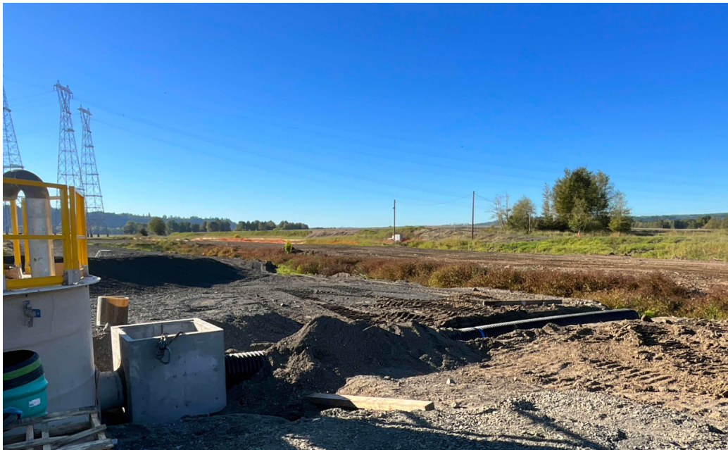
Installation of overflow vault and 18-inch corrugated polyethylene pipe (CPE).
