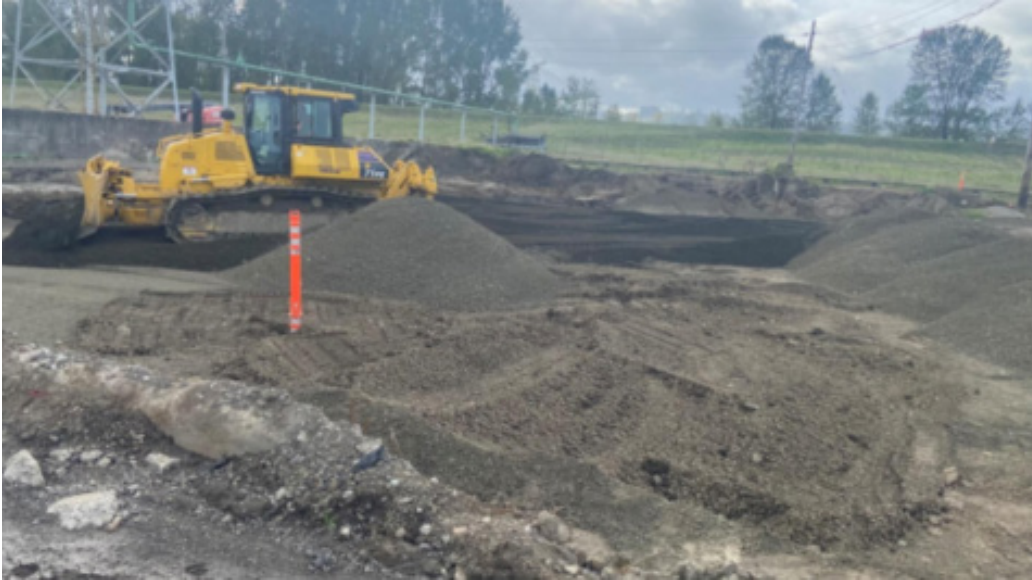
Placement of select fill in SU9.
