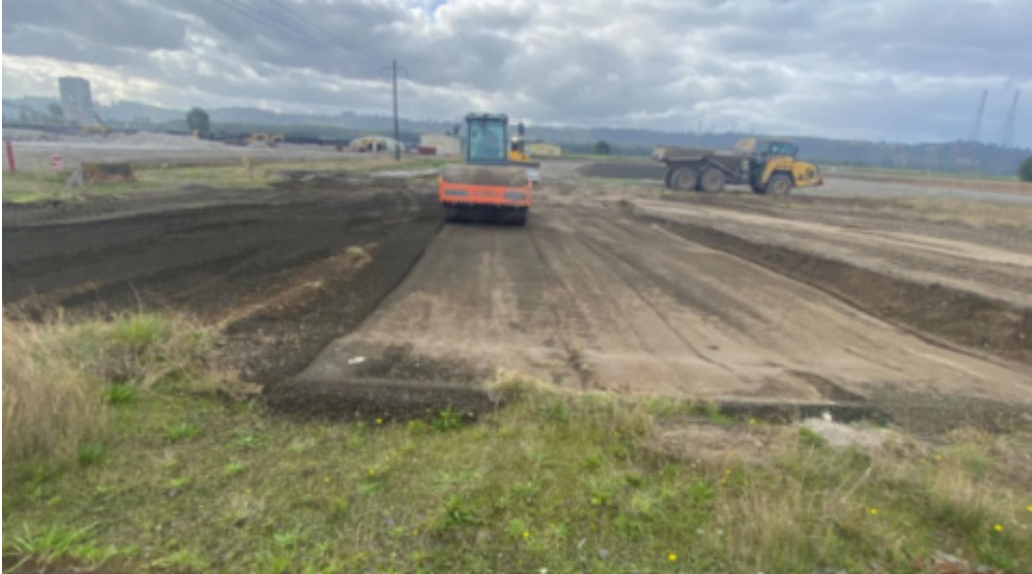
Final grading and compaction of crushed gravel surface material in SU11.
