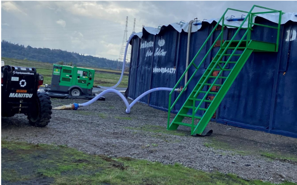
Installation of temporary connection from water storage tank to Facility 77.
