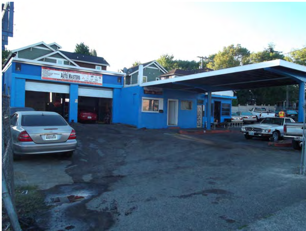
Photograph 1 – View east from the northwest corner of the fenced portion of the Property showing the canopy of the former pump islands, the two automotive repair bays, and the surface drainage pathway (lower left).
