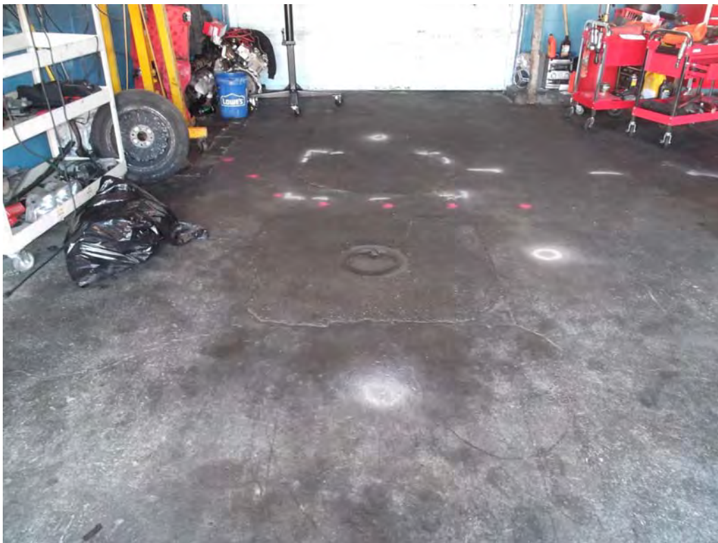
Photograph 4 – View of the interior of the northern automotive repair bay, showing the former hydraulic lift (center) and the square outline of the hydraulic oil UST. Boring KSB-2 is shown in white beyond the UST.
