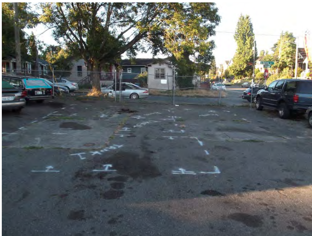
Photograph 2 – View south of the southern portion of the Property showing the painted outlines of four (4) fuel storage USTs remaining in place from the former gas station on the Property (See Figure 3).
