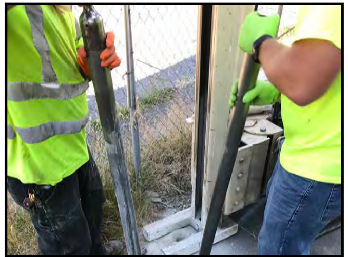
Removing boring casing
