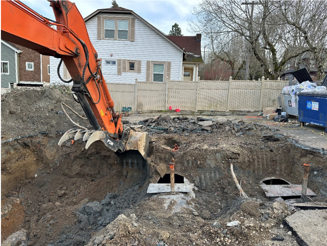
Photograph 13 – View of the former UST-1 location, PCS removal as indicated by the gray colored soil, and UST-2 (center) and UST-3 (right) awaiting removal.
