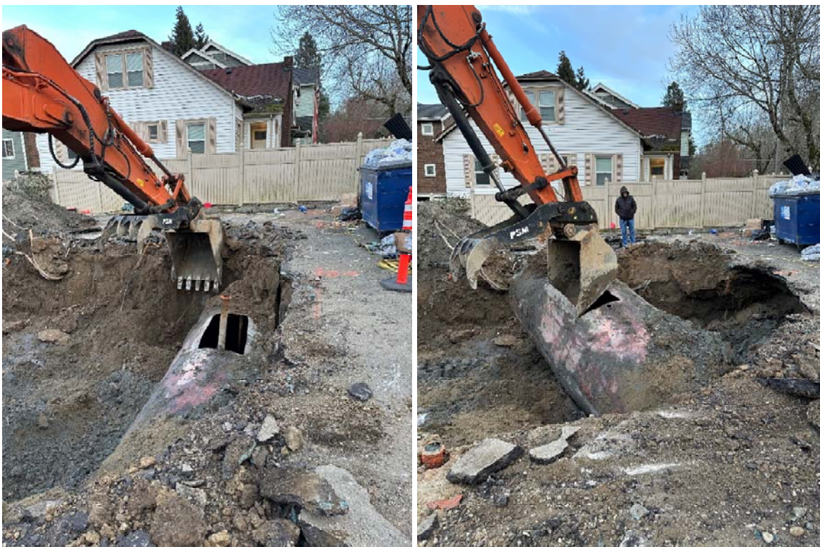
Photograph 15 – Two views of UST-3, showing it in place with top cut open (left) and being removed from the ground by the excavator (right).
