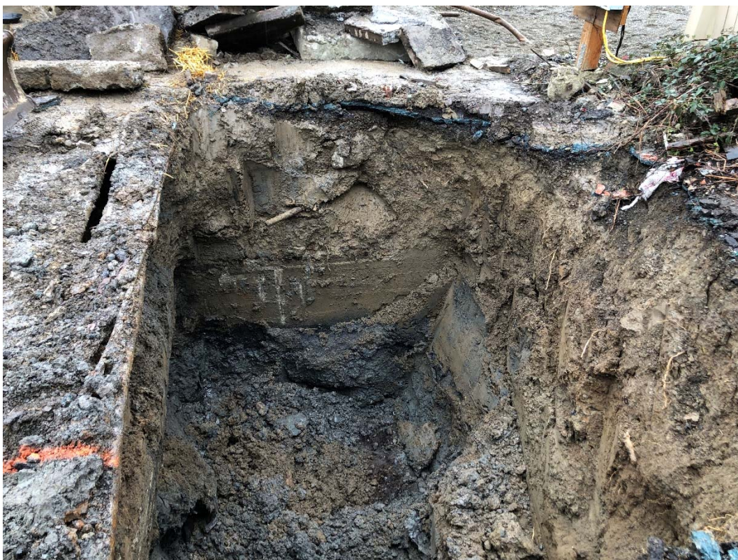
Photograph 21 – View of Heating Oil UST AOC excavation, showing the excavation extending to the depth of approximately 10 feet bgs where the dark brown silty organic soil was encountered beneath the gray PCS. Concrete debris is shown (center).
