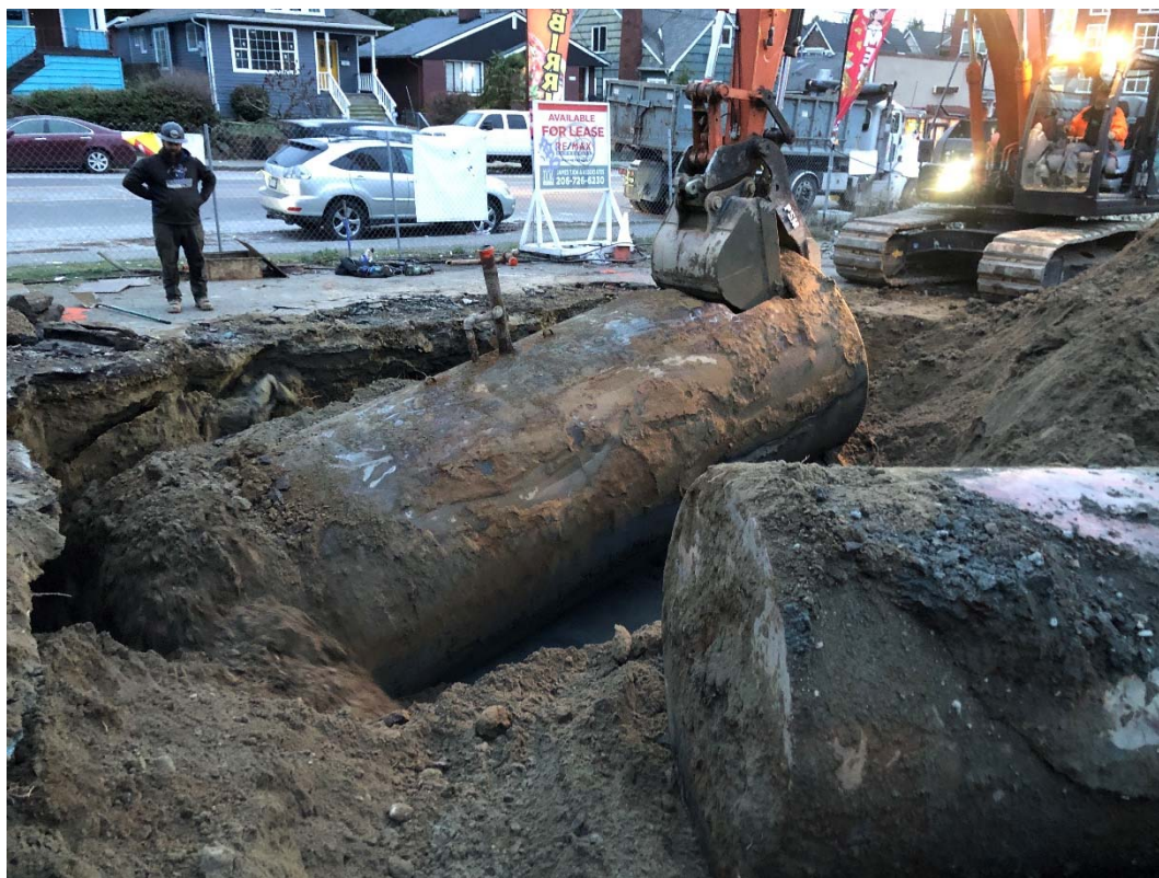
Photograph 16 – View of UST-4 being removed from the ground by the excavator.
