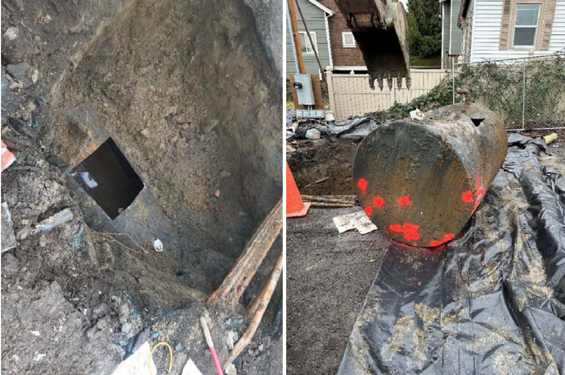
Photograph 5 – Two views showing the removal of the heating oil UST (UST-6), including in the ground with the top exposed and cut open (left), and removed from the ground with holes in the western wall of the UST painted (right).
