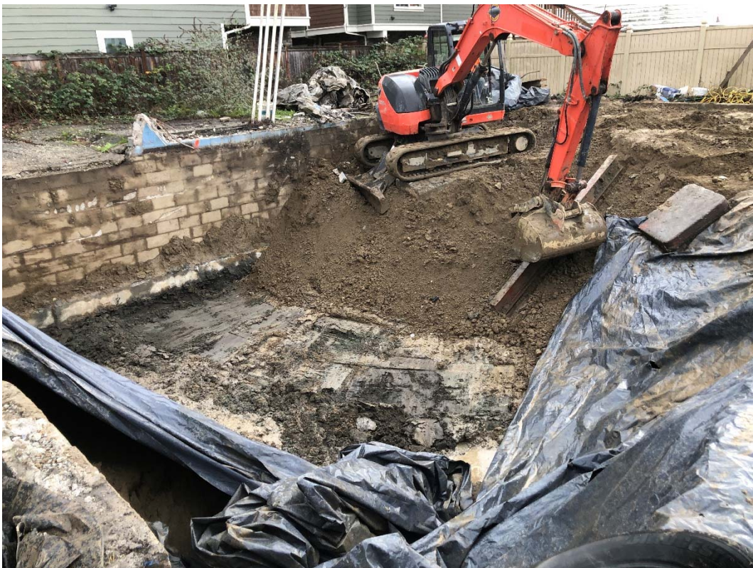
Photograph 8 – View of the excavation in the Automotive Repair Shop AOC, showing the completion of the excavation to the silty organic soil layer present approximately 8.5 feet bgs. Gas station UST vent pipes are shown.
