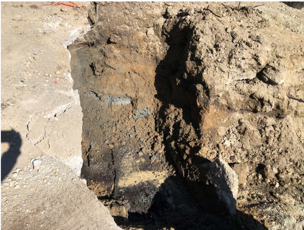
Photograph 30 – View of the Pump Island AOC excavation, showing the dark brown silty organic soil zone encountered approximately 8.5 feet to 9.5 feet bgs in this portion of the Property.
