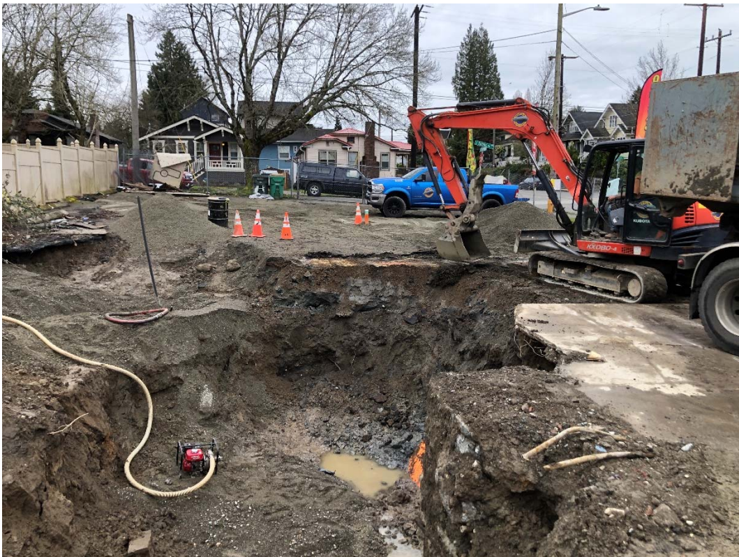
Photograph 26 – Excavation in the Pump Island AOC, showing gray PCS and remnants of the former pump island concrete slab. The mostly backfilled Heatin Oil UST AOC excavation area is shown (center-left).
