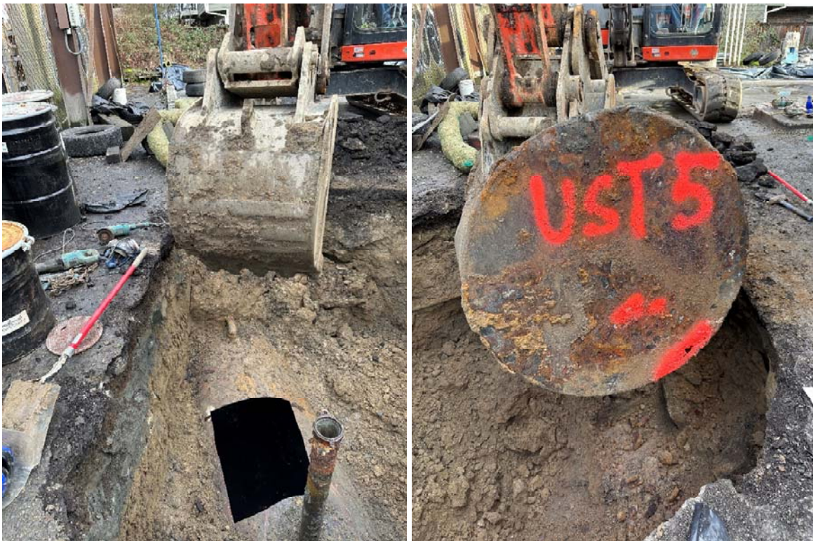
Photograph 4 – Two views showing the removal of the waste oil UST (UST-5), including in the ground with the top exposed and cut open (left), and removed from the ground with holes in the western wall of the UST painted (right).
