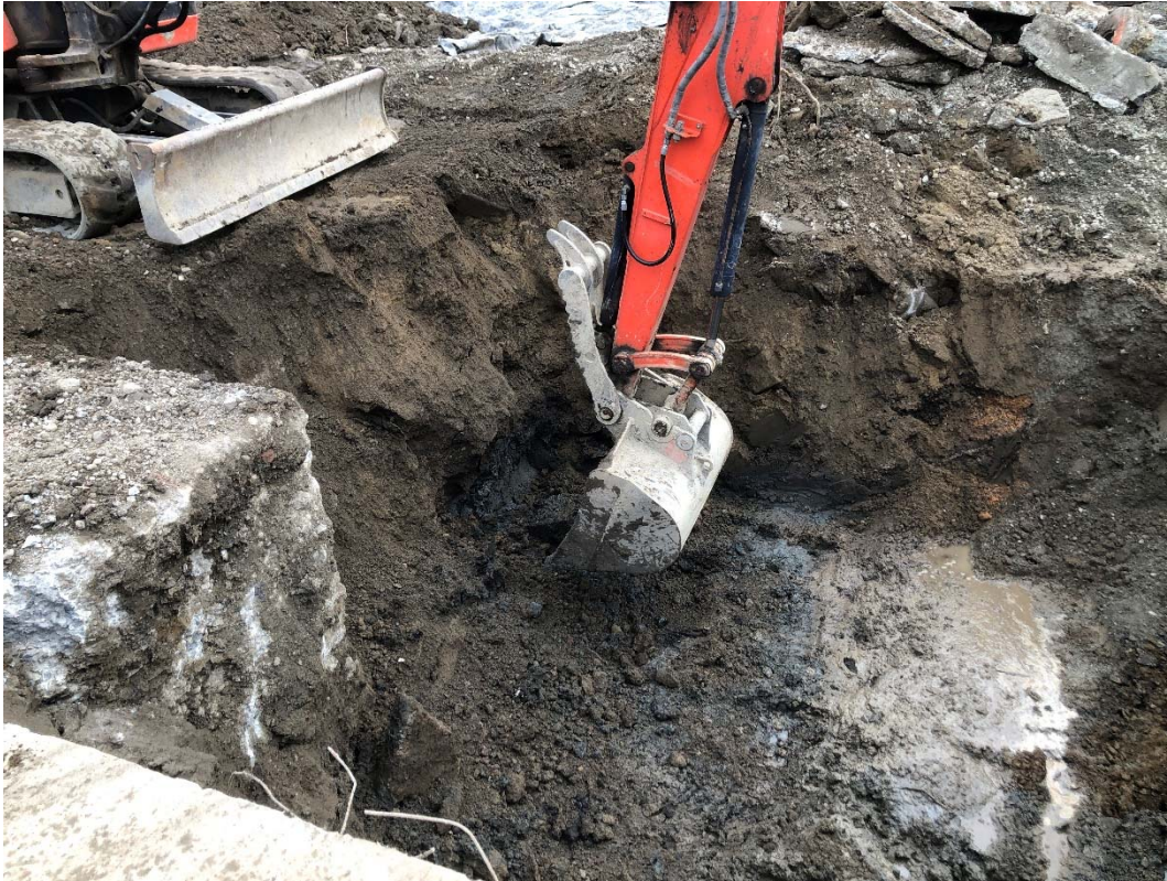
Photograph 25 – Excavation in the Pump Island AOC, showing removal of gray PCS and concrete debris. The large concrete block (left) was the eastern foundation for the pump island canopy support.
