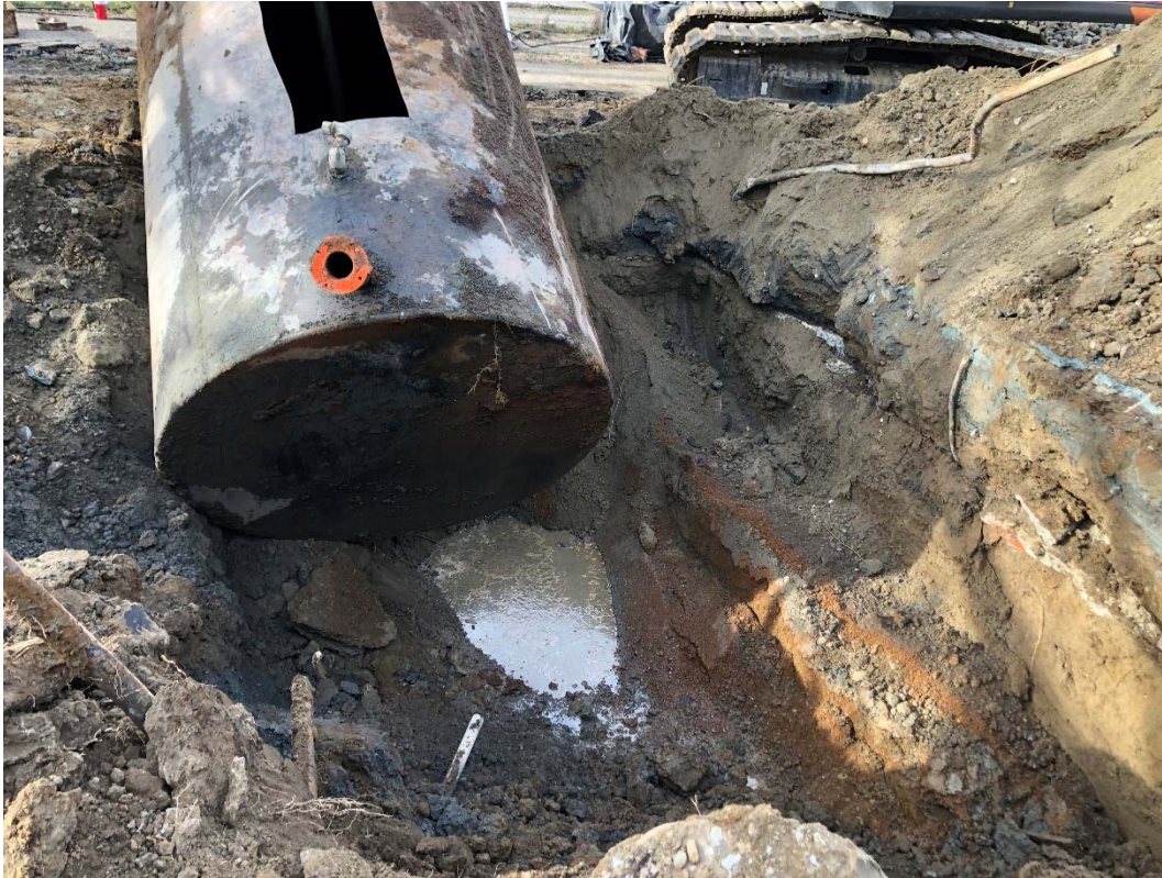
Photograph 11 – View of the Gas Station AOC in the southern portion of the Property, showing UST-1 being removed from the ground, exposing groundwater accumulated beneath with the UST pit fill material.
