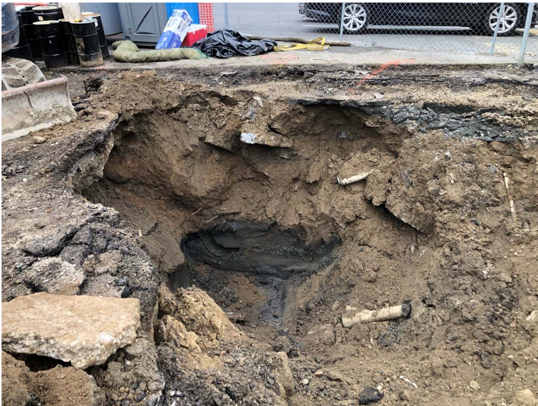
Photograph 24 – View of the Waste Oil UST AOC excavation, showing completion to the silty organic layer present approximately 10 feet bgs and PCS remaining in place approximately 7 feet to 9 feet bgs along the north sidewall (center).
