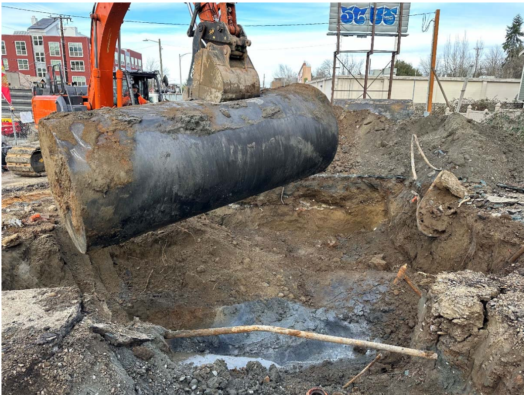
Photograph 14 – View of the UST-2 removal, showing underlying PCS indicated by the gray colored soil. UST-3 fill port is shown remaining in place (bottom-center).
