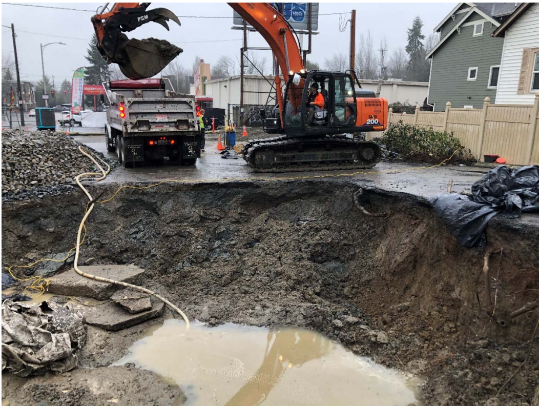
Photograph 18 – Representative view of Gas Station USTs AOC excavation, showing removal of PCS and the presence of accumulated rainwater and groundwater, which was pumped into totes for offsite disposal. Stockpiled quarry spalls backfill is present (left), ready to be placed following excavation to final depth.
