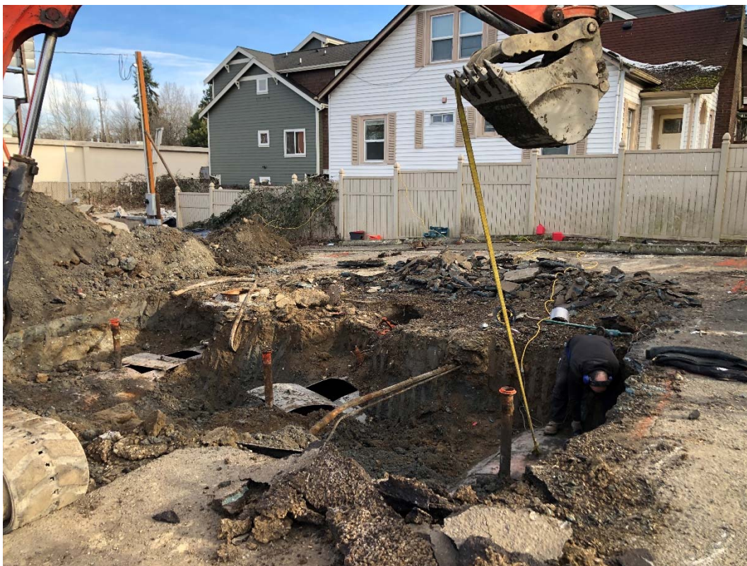
Photograph 10 – View of the Gas Station AOC in the southern portion of the Property, showing UST-1 (left) and UST-2 (center) exposed and cut open, and UST-3 (right) being cut open.
