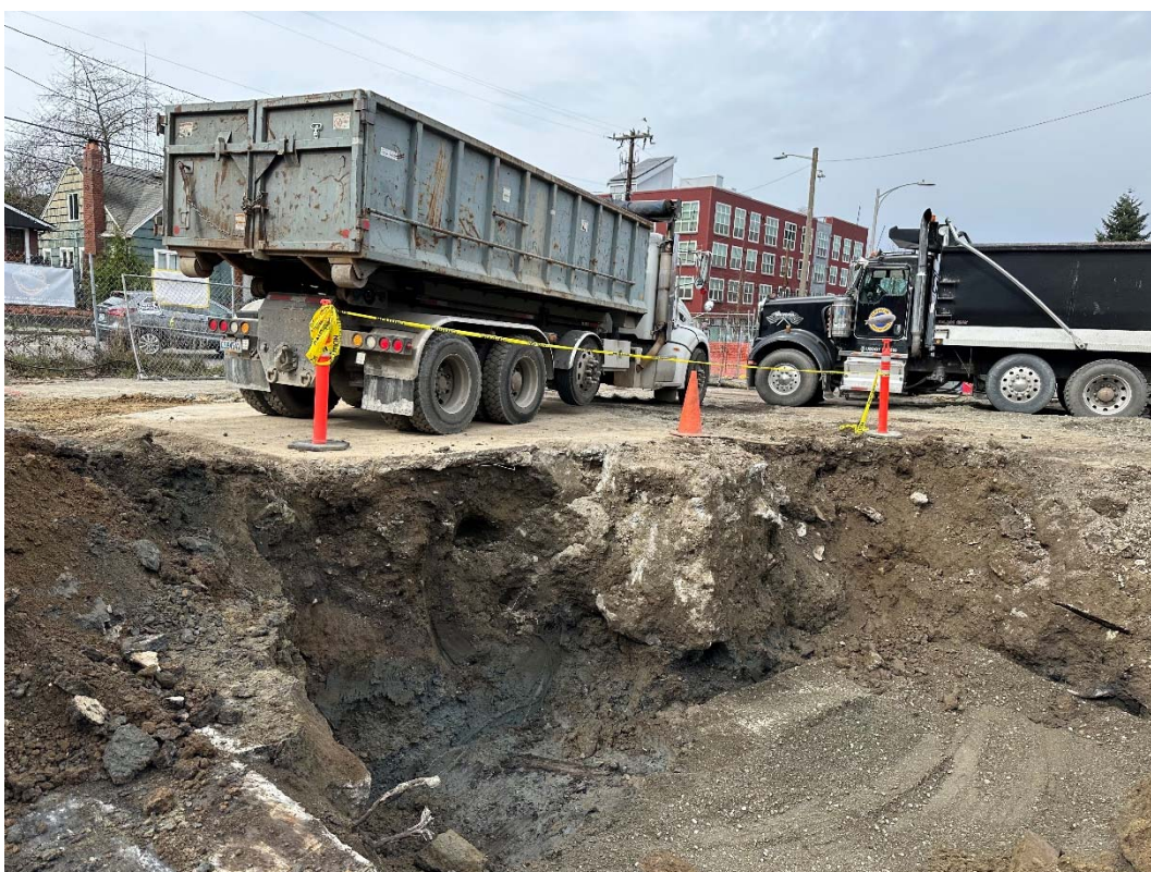
Photograph 22 – View of the completed Heating Oil UST AOC excavation, showing the type 17 backfill (lower right), and gray PCS associated with the Pump Island AOC remaining for upcoming removal.
