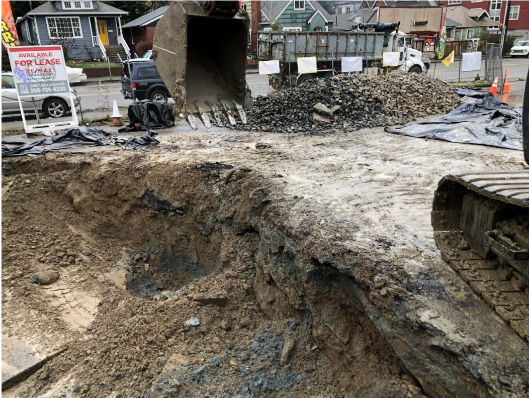
Photograph 17 – Representative view of Gas Station USTs AOC excavation following removal of all USTs, showing the presence of a zone of PCS approximately 7 feet to 10 feet bgs to the north of the former UST-4 location and west of the former UST-1 location indicated by gray soil (left of center).
