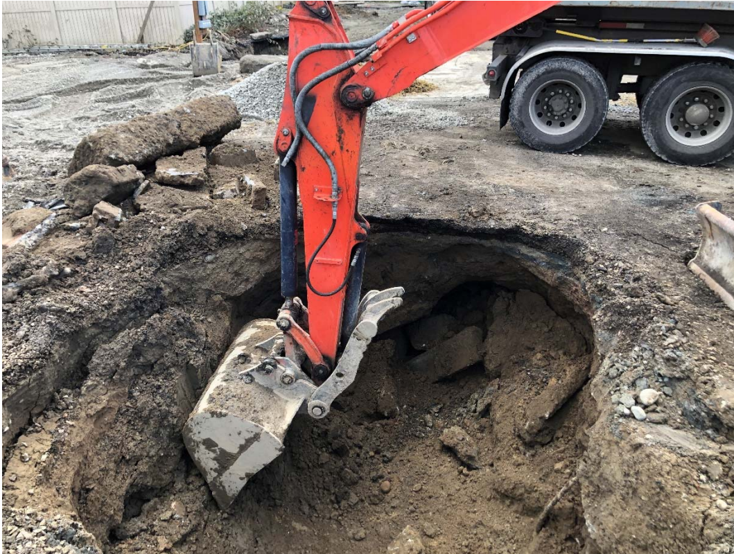
Photograph 23 – View of the Waste Oil UST AOC excavation, showing removal of PCS and the presence of concrete debris surrounding the former UST location.
