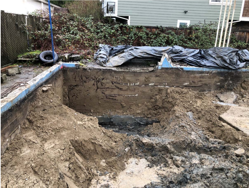
Photograph 7 – View of the excavation in the Automotive Repair Shop AOC, showing the removal of PCS in the northeastern portion of the excavation to the silty organic soil layer present approximately 8.5 feet bgs beneath the base of the western foundation wall. The northern foundation wall (left) remains supported by soil.
