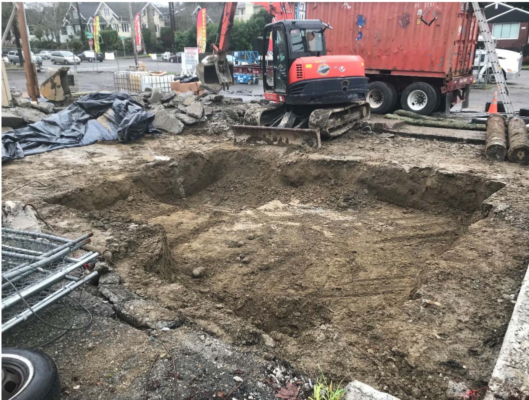
Photograph 6 – View of the initial excavation in the Automotive Repair Shop AOC, showing removal of soils for Contained-In Disposal (CID) to approximately 3 feet below ground surface (bgs). The two hydraulic lift cylinders removed from the ground are shown (right).
