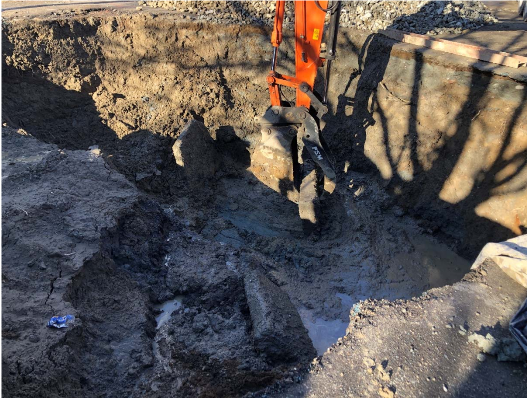
Photograph 19 – View of Gas Station USTs AOC excavation, showing the completion of the excavation to the depth of the silty organic layer encountered approximately 12 feet to 13 feet bgs in this portion of the Property.
