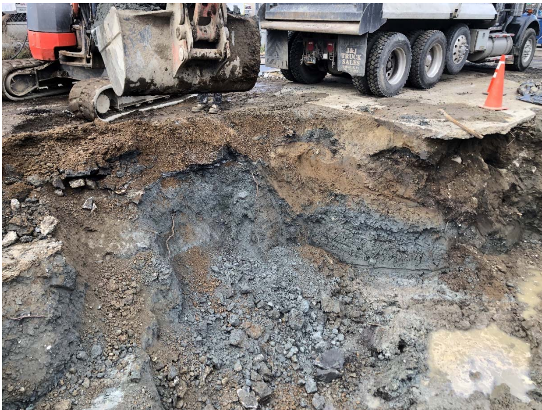
Photograph 27 – Further excavation in the Pump Island AOC, showing gray PCS and remnants of the former pump island concrete slab.
