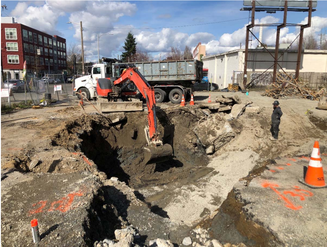
Photograph 29 – View north of the Pump Island AOC excavation, showing the backfilled eastern portion of the AOC and concrete debris. The eastern large concrete canopy support is shown (center-right).
