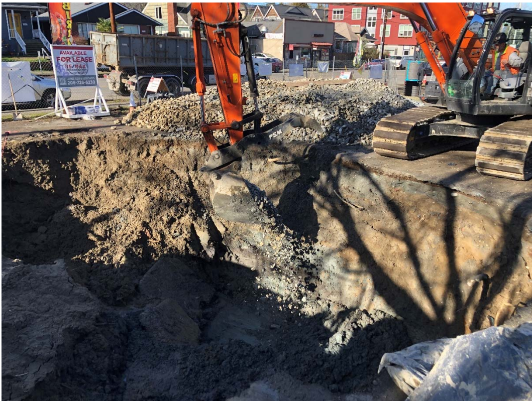
Photograph 20 – View of Gas Station USTs AOC excavation, showing placement of quarry spalls backfill at the base of the completed excavation.
