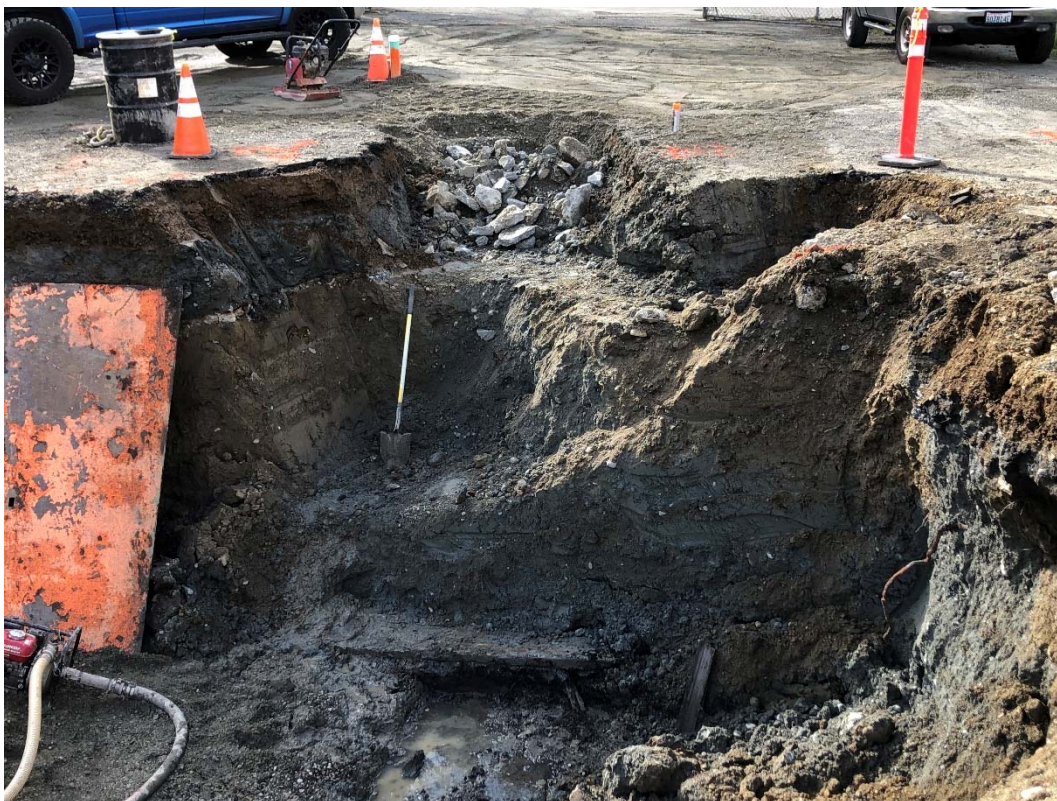
Photograph 28 – View south showing the southern extent of the Pump Island AOC excavation, and the 3-foot bgs excavation that followed the former transfer lines from the Gas Station USTs AOC (center-top) to the former pump islands.
