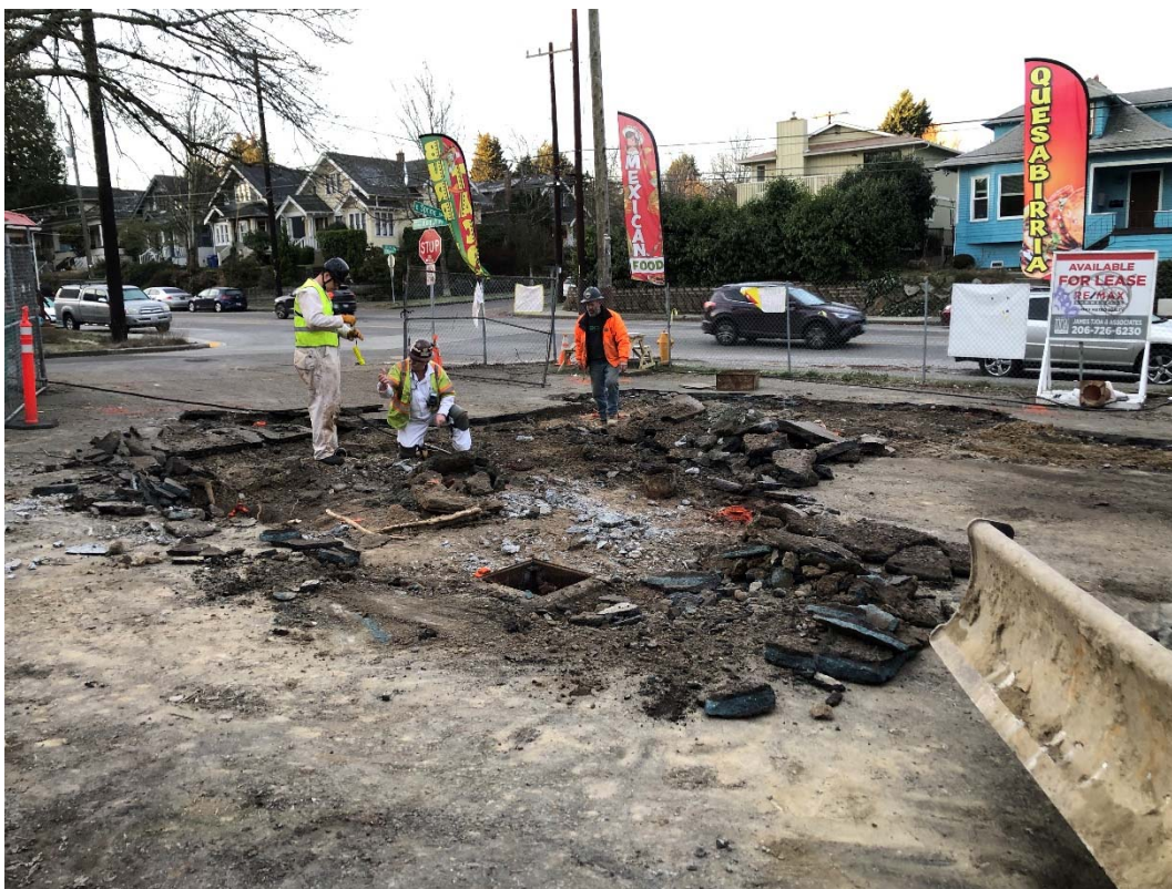
Photograph 9 – View of the Gas Station AOC in the southern portion of the Property, showing the removal of the asphalt surface. The Marine Chemist is shown testing vapors in UST-3 to determine that it is safe to cut open.
