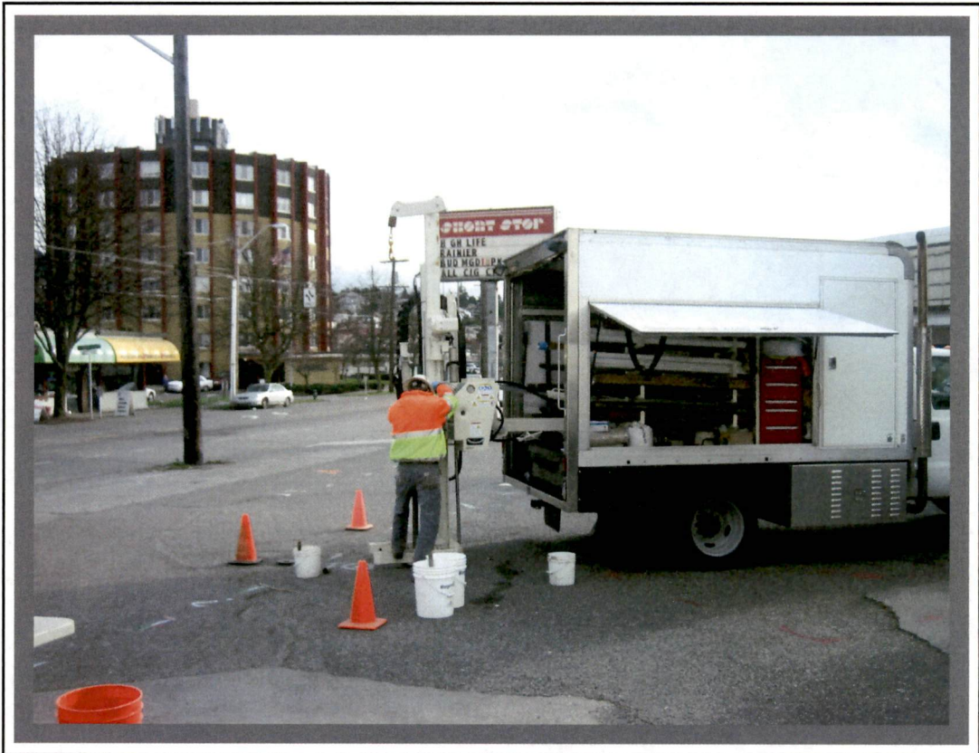
Photograph 1. This photograph shows Pacific Soil & Water installing push probe PP-1 at the upgradient location within the former UST excavation pit.
