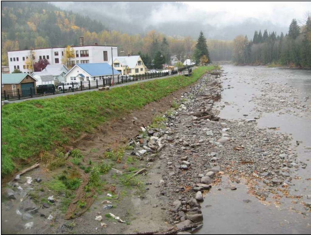
Photograph 11. Photo Point 9, on Skykomish River Bridge, facing downstream.
