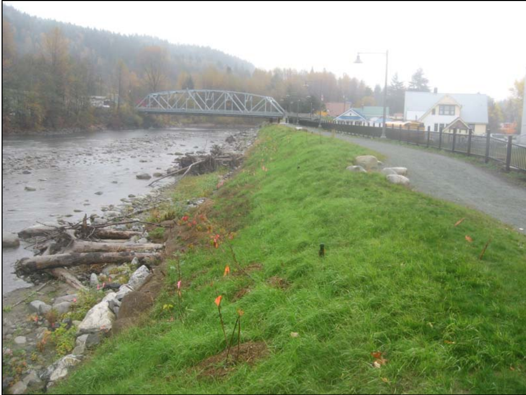
Photograph 1. Photo Point 1, top of levee, facing upstream.
