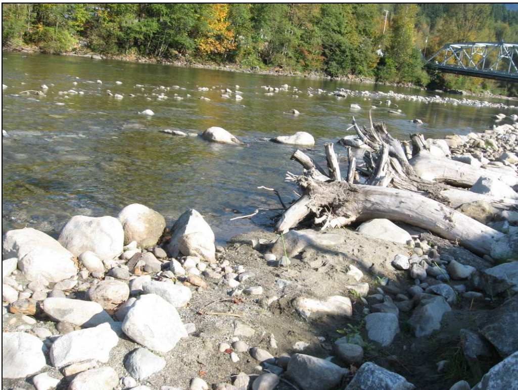
Photograph 21. Live stakes installed 10-10-08, facing upstream/east
