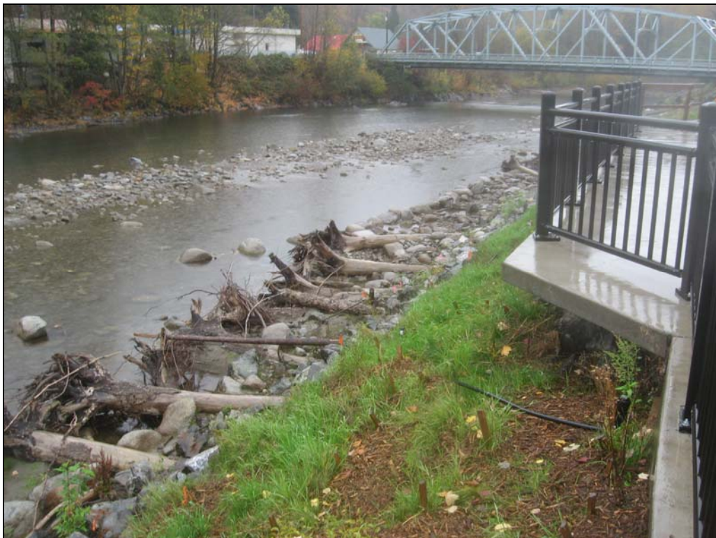
Photograph 4. Photo Point 3, top of levee, facing LWD structures below view platform.
