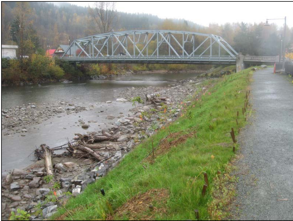
Photograph 7. Photo Point 5, facing upstream.
