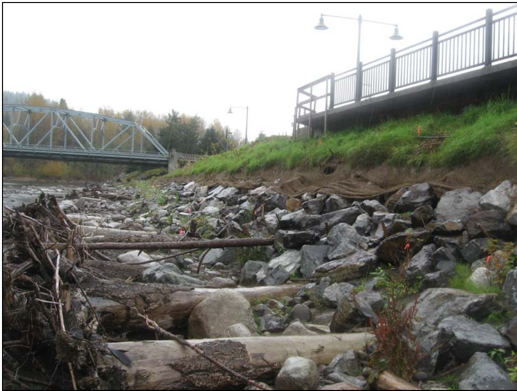
Photograph 5. Photo Point 4, facing upstream.
