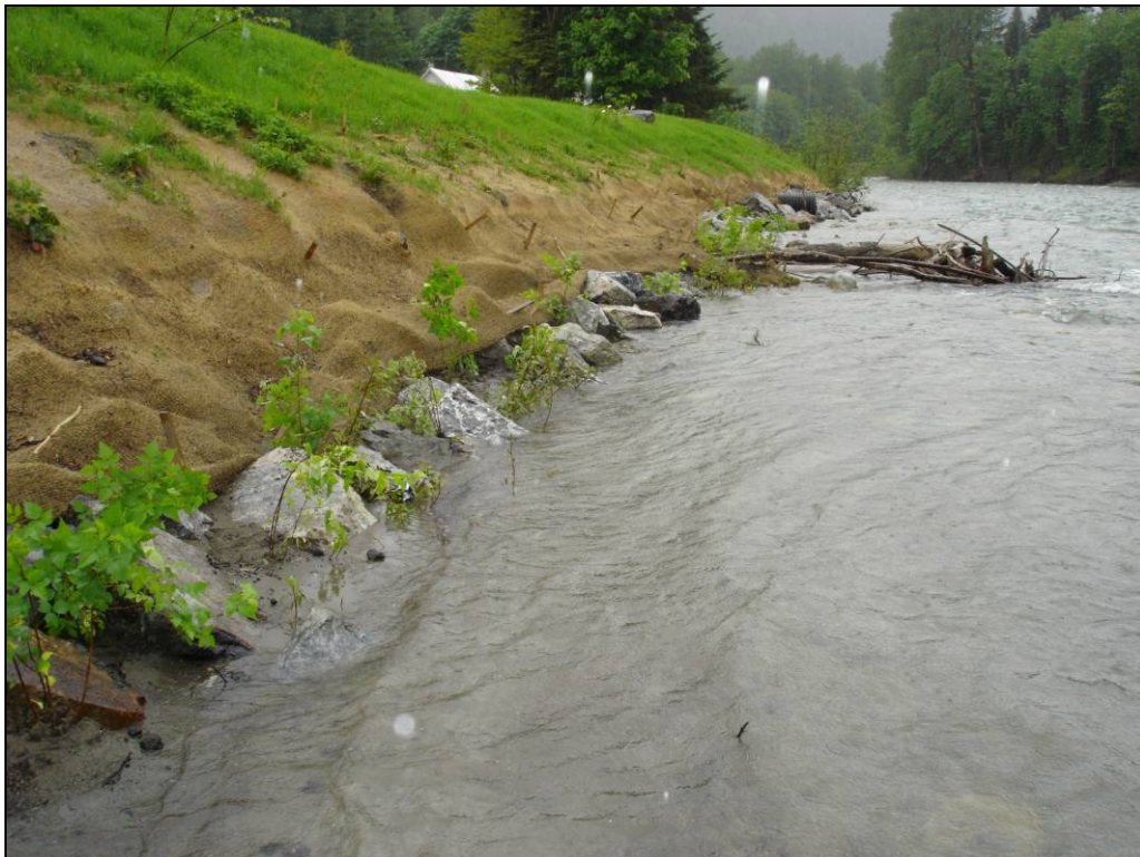
Photograph 15. Salmonberry installation on June 5, 2008; facing west/downstream.
