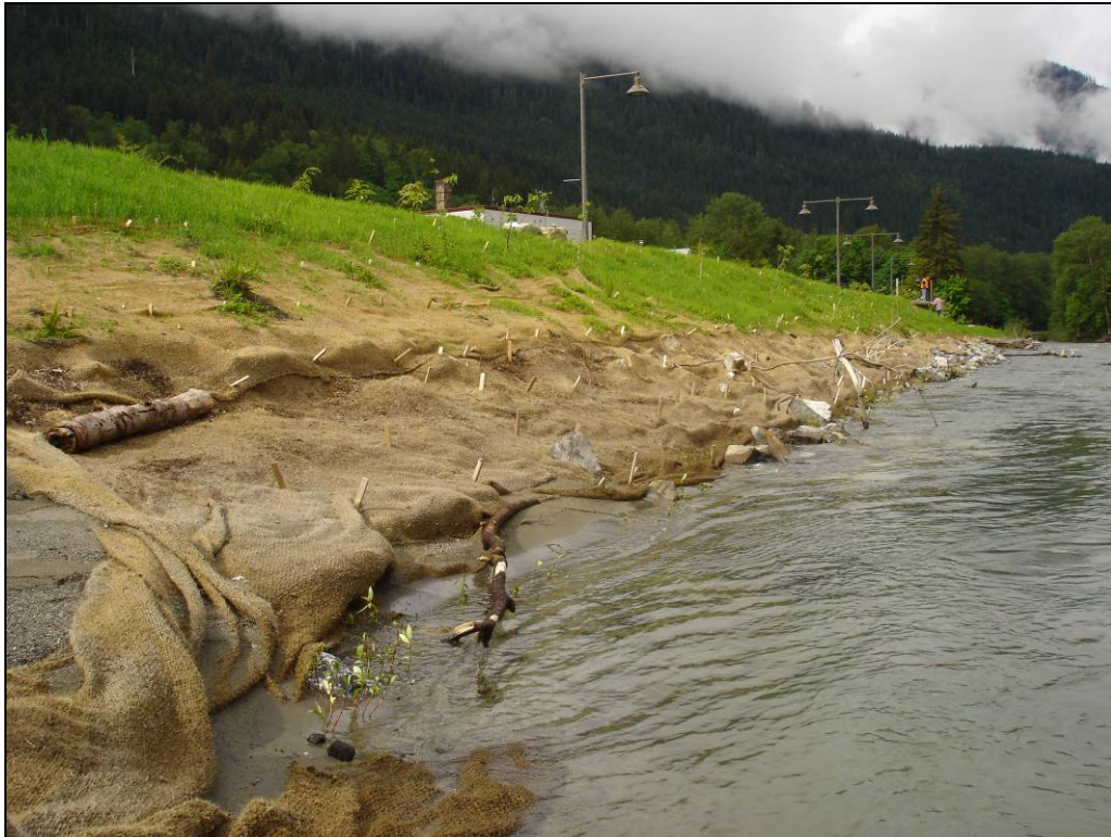
Photograph 12. Salmonberry installation on June 5, 2008; facing west/downstream.
