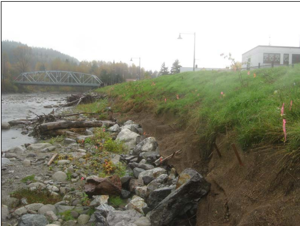
Photograph 2. Photo Point 2, bottom of levee, facing upstream.
