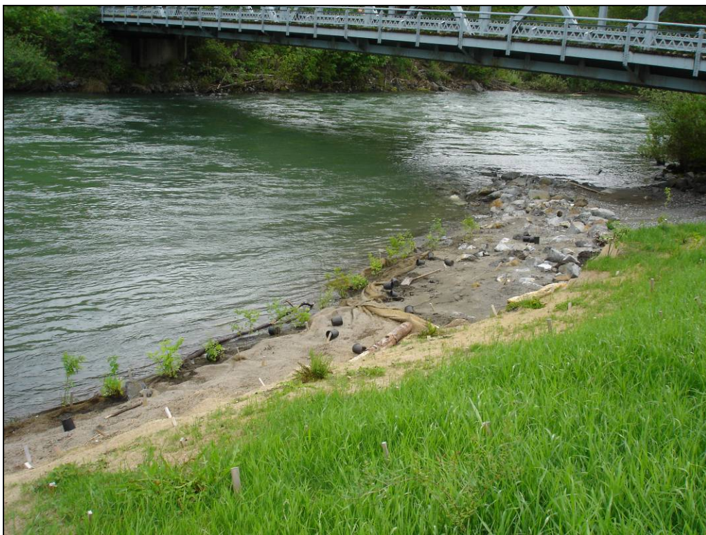
Photograph 13. Salmonberry installation on June 5, 2008; facing northeast/upstream.
