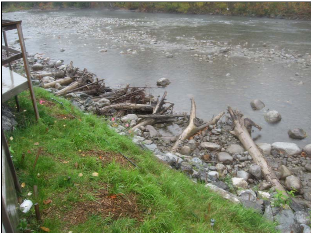
Photograph 6. Photo Point 5, facing downstream toward LWD structures below view platform.
