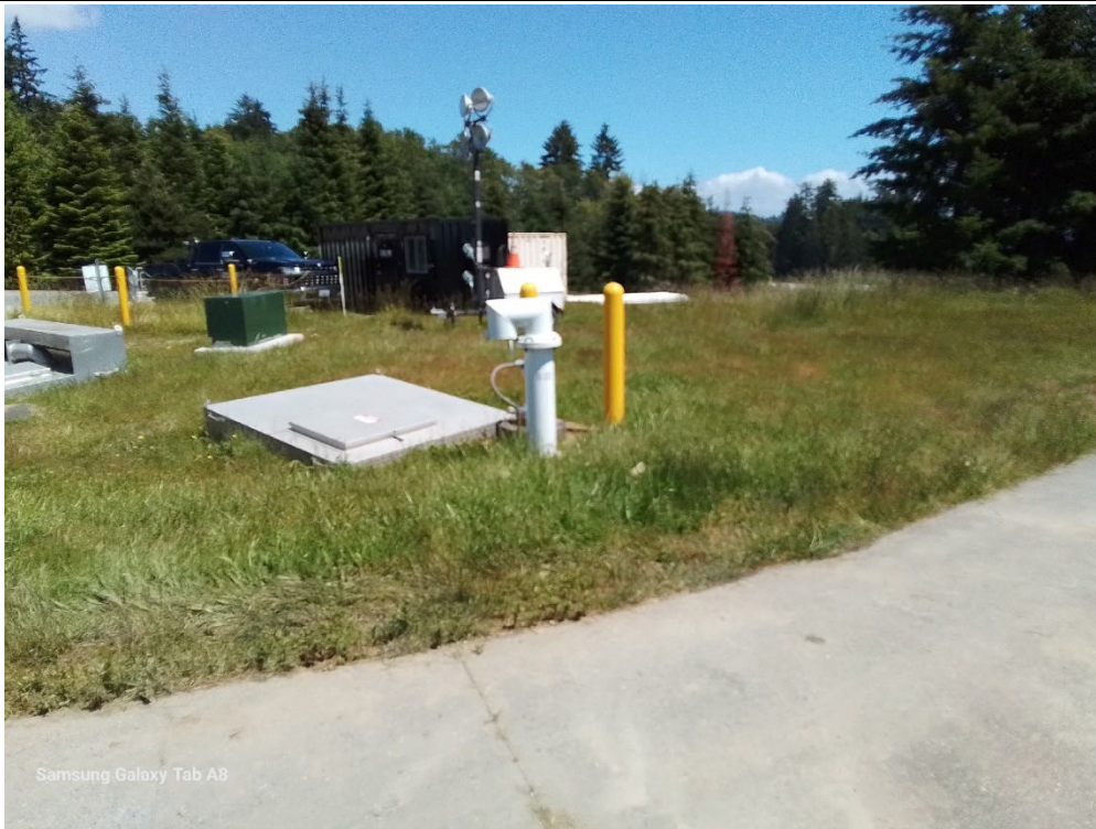
Photograph 3 Locations of former vapor monitoring wells and installed vault, facing northeast.
