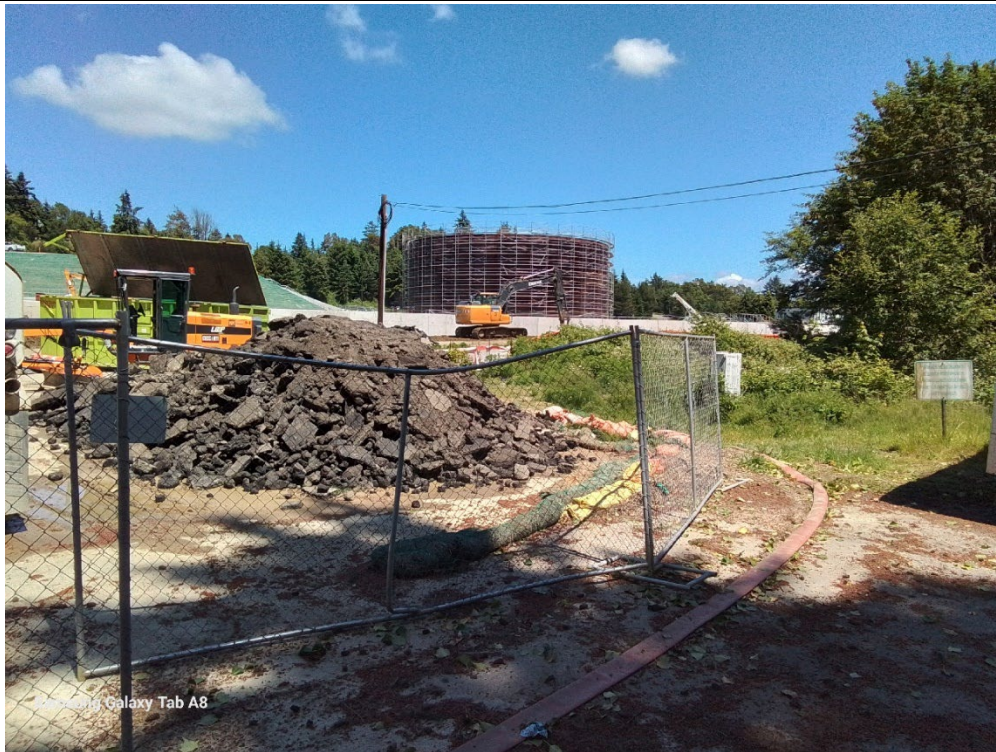
Photograph 11 Construction activities, facing northeast.
