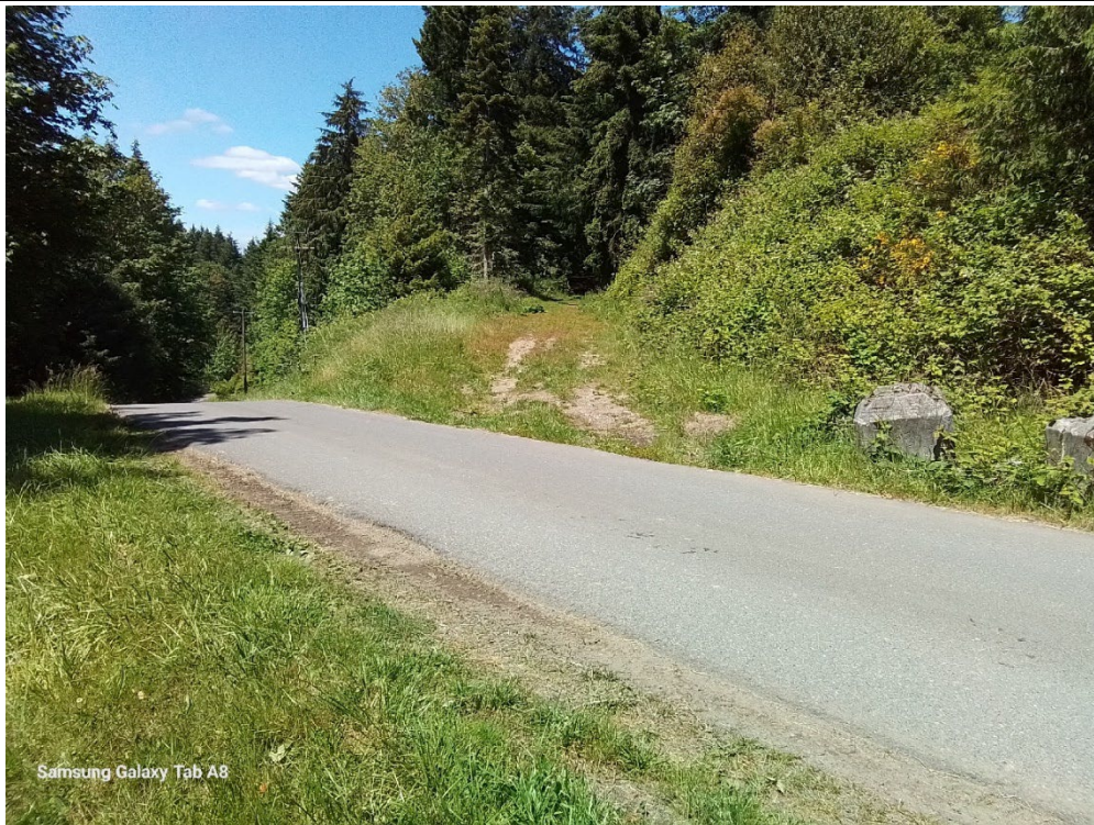
Photograph 16 Area southwest of Tank 28 along the perimeter road.
