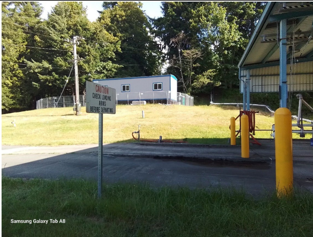
Photograph 3 Tanker truck facility and containerized fuel related waste, facing northeast.
