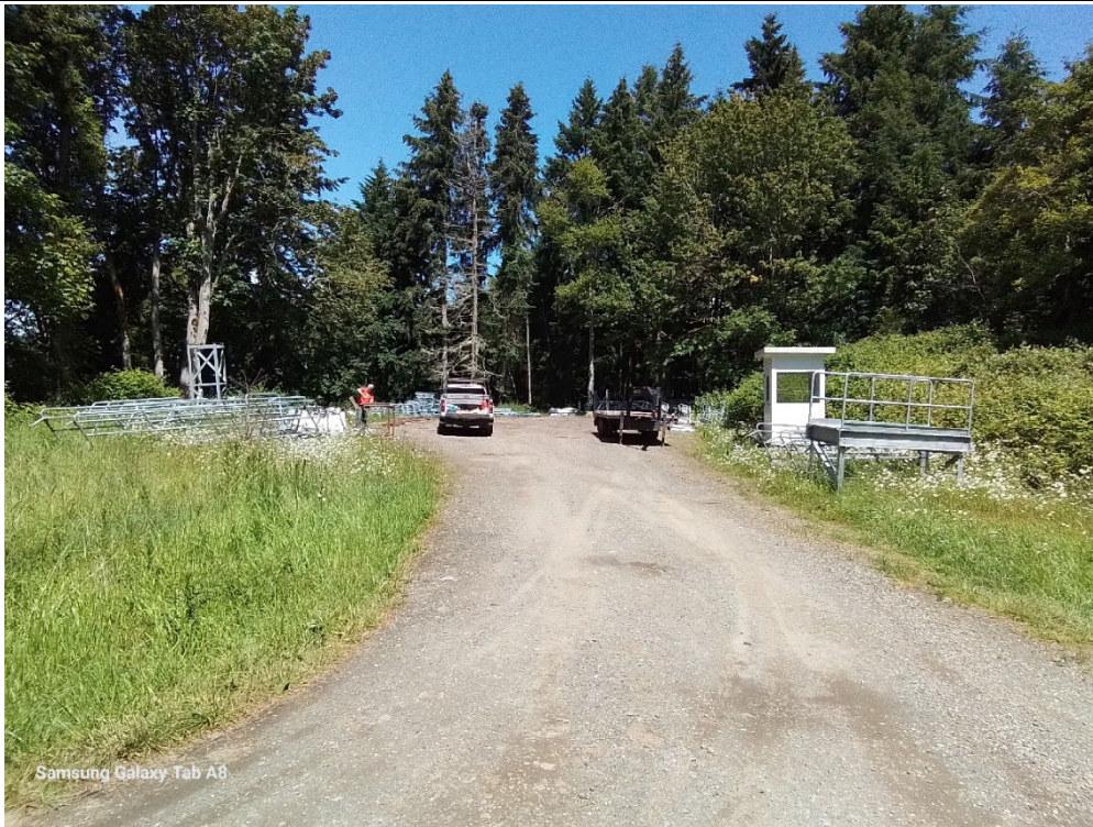
Photograph 19 Construction laydown yard north of Tank 29, facing north.
