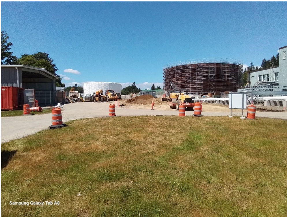
Photograph 4 Active construction activities near Tank 22, facing west.
