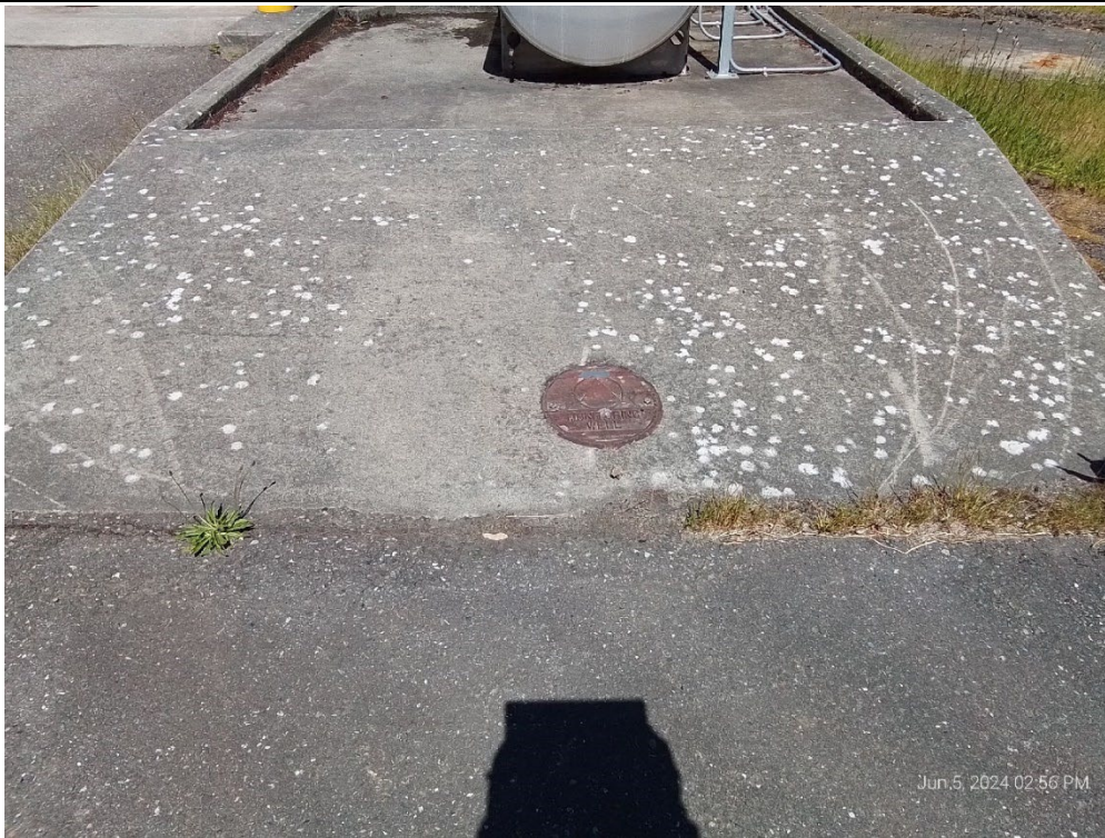
Photograph 11 Groundwater monitoring well MW-2, facing northeast.
