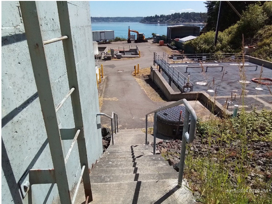
Photograph 9 Western central boundary of site, facing south.
