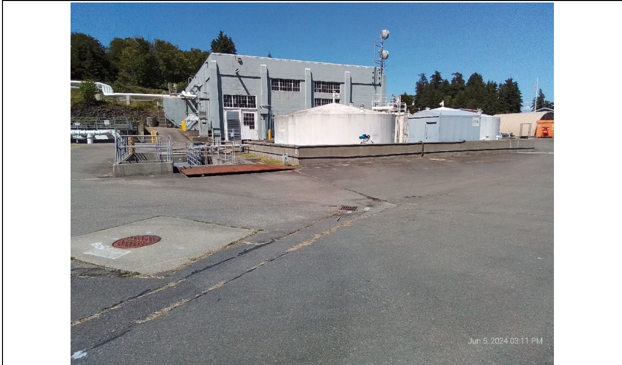
Photograph 7 Southwest boundary of site, facing northeast.
