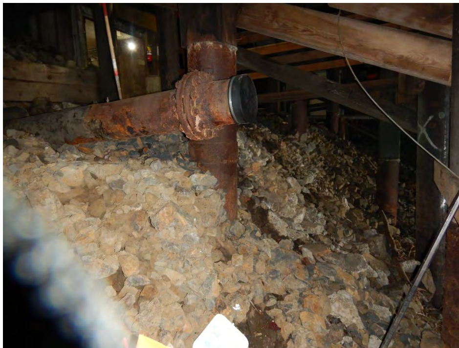
Photograph 3. View of eastern pipeline beneath Berth 2 and locations of P3 and P4. Accumulated soil was sparse due to abundant riprap.
