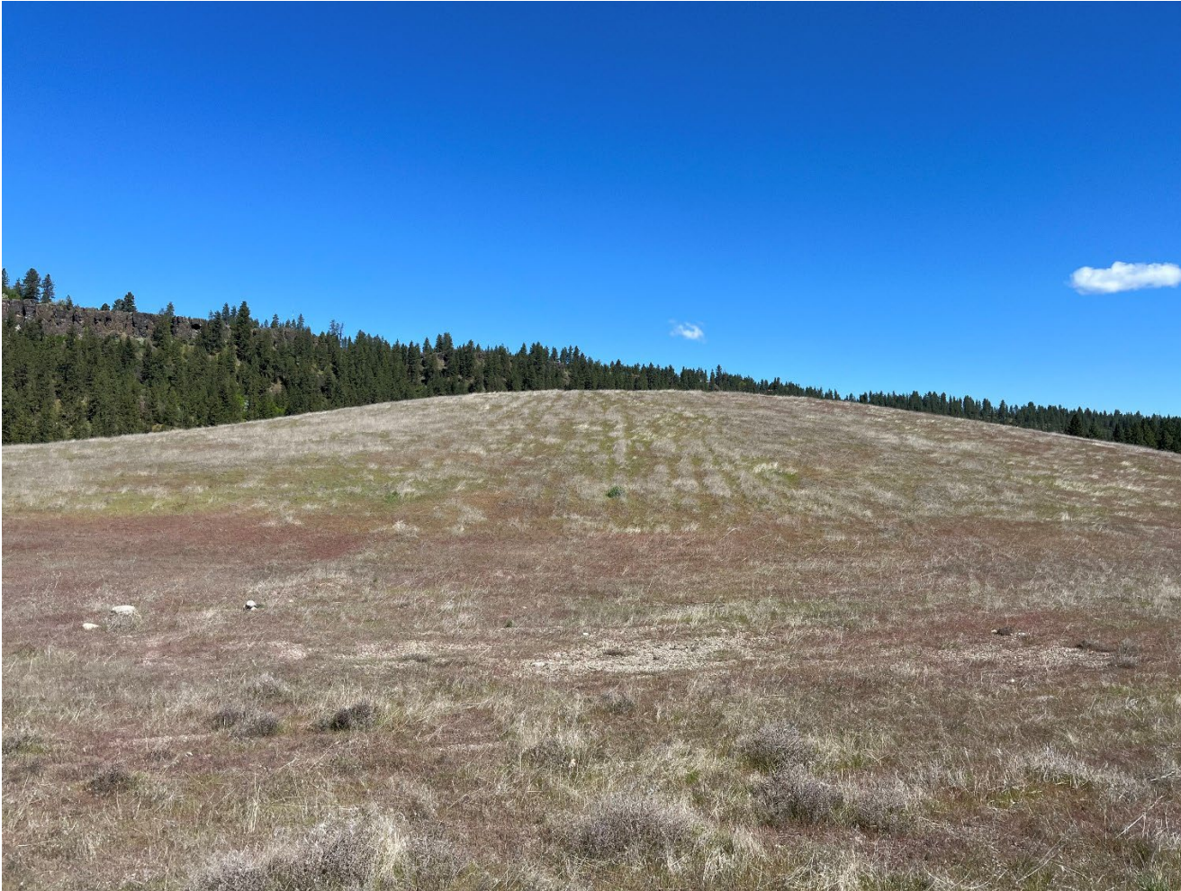
Photo 1: Landfill cap looking north/northeast
