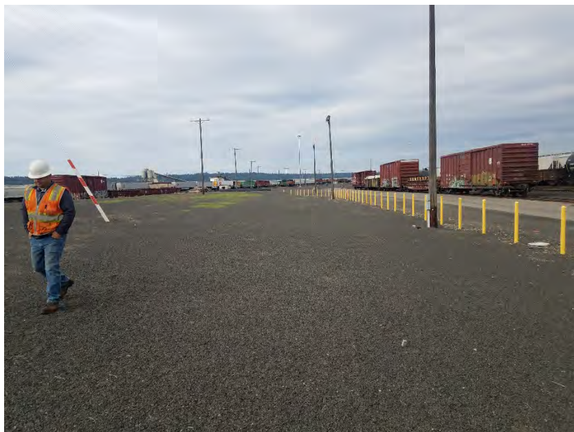
Photograph 1 – Looking to west. 6/28/2018
