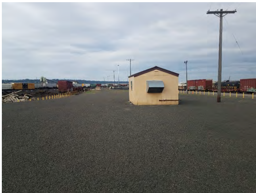
Photograph 3 – Looking to southeast. 6/28/2018
