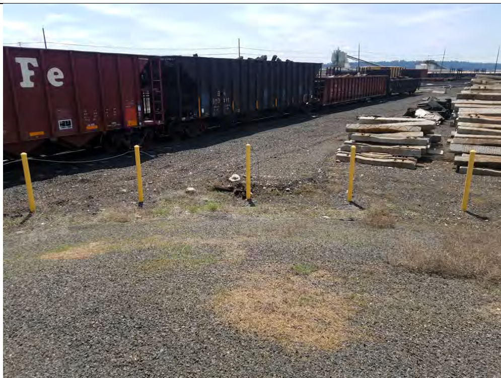
Photo #4: Damage to southwestern fence corner.
