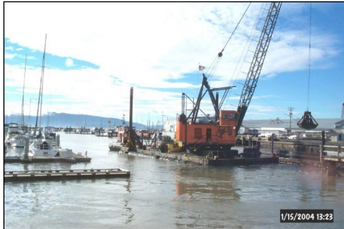
Figure 3: Loading contaminated sediment into a barge during the 2004 interim action
