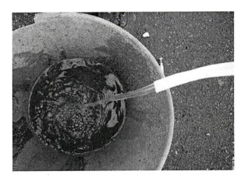
The Pump was moved up and down the Well Screen to ensure that excess material was removed from the surrounding Sand Pack. The well was pumped until the water was clear and free of suspended soilds
