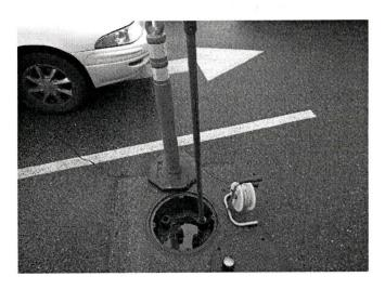
Each Well was Surged using a Surge Block in a Rapid, Repetitive Up-and-Down motion over the Entire Water Column to loosen Silt and Fine Sand
