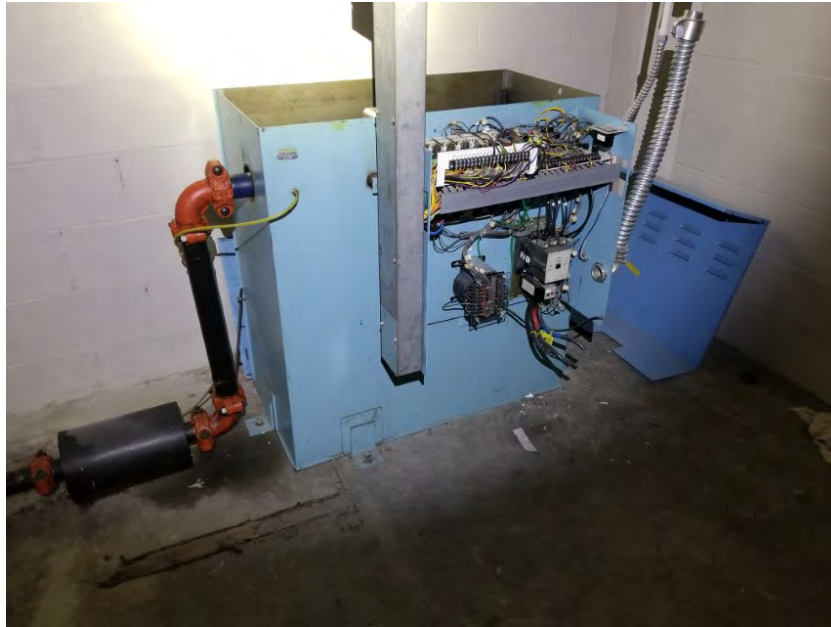
Photo 25. View Direction: Northeast Viewing the hydraulic tank and equipment in the elevator equipment room on the first floor of the 1916 Boren Avenue building. Minor staining on the concrete floor beneath the equipment motor on the left. The lid to the hydraulic tank is to the right.
