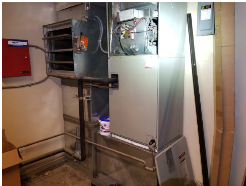
Photo 29. View Direction: Southeast Viewing natural gas furnace and air handler in the fire alarm control room on the first floor of the 1916 Boren Avenue building.
