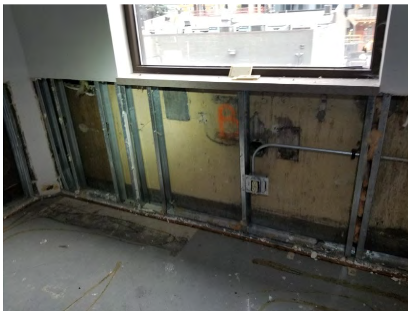
Photo 30. View Direction: East Viewing a wall on the third floor of the 1916 Boren Avenue building with drywall and insulation removed revealing concrete wall aluminum studs.
