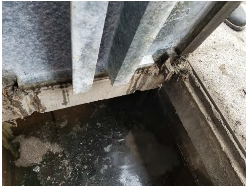
Photo 20. View Direction: South Viewing the clear water of the oil-water separator at the southeast corner of the subject property. Non-oily dirt is floating on the surface of the water.
