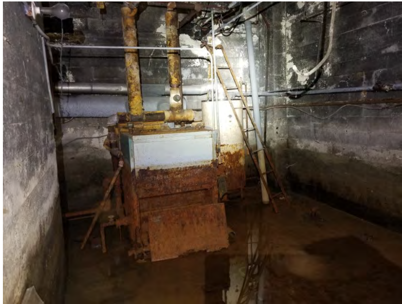
Photo 34. View Direction: Southeast Viewing the dilapidated boiler in the basement at the southeast corner of the 1916 Boren Avenue building.
