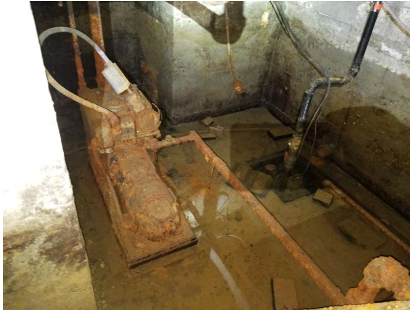
Photo 35. View Direction: East Viewing boiler water pump (left) and below-grade basement sump pump (right) in the basement boiler room at the southeast corner of the 1916 Boren Avenue building.
