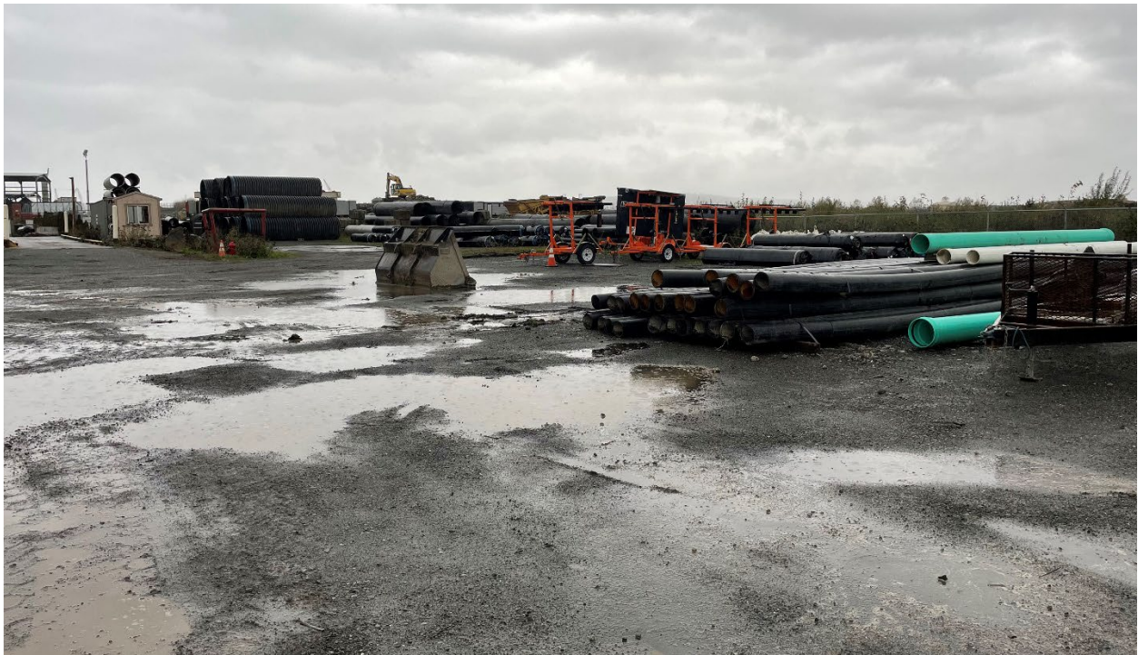
Photo 5: Graveled material/equipment storage area, looking northwest, toward Cleanup Area 12 (vegetated area in background).
