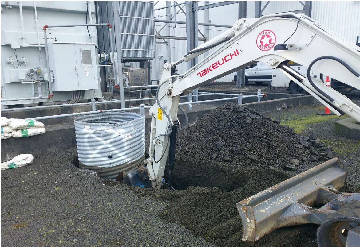
Excavating fill to allow casing removal.
