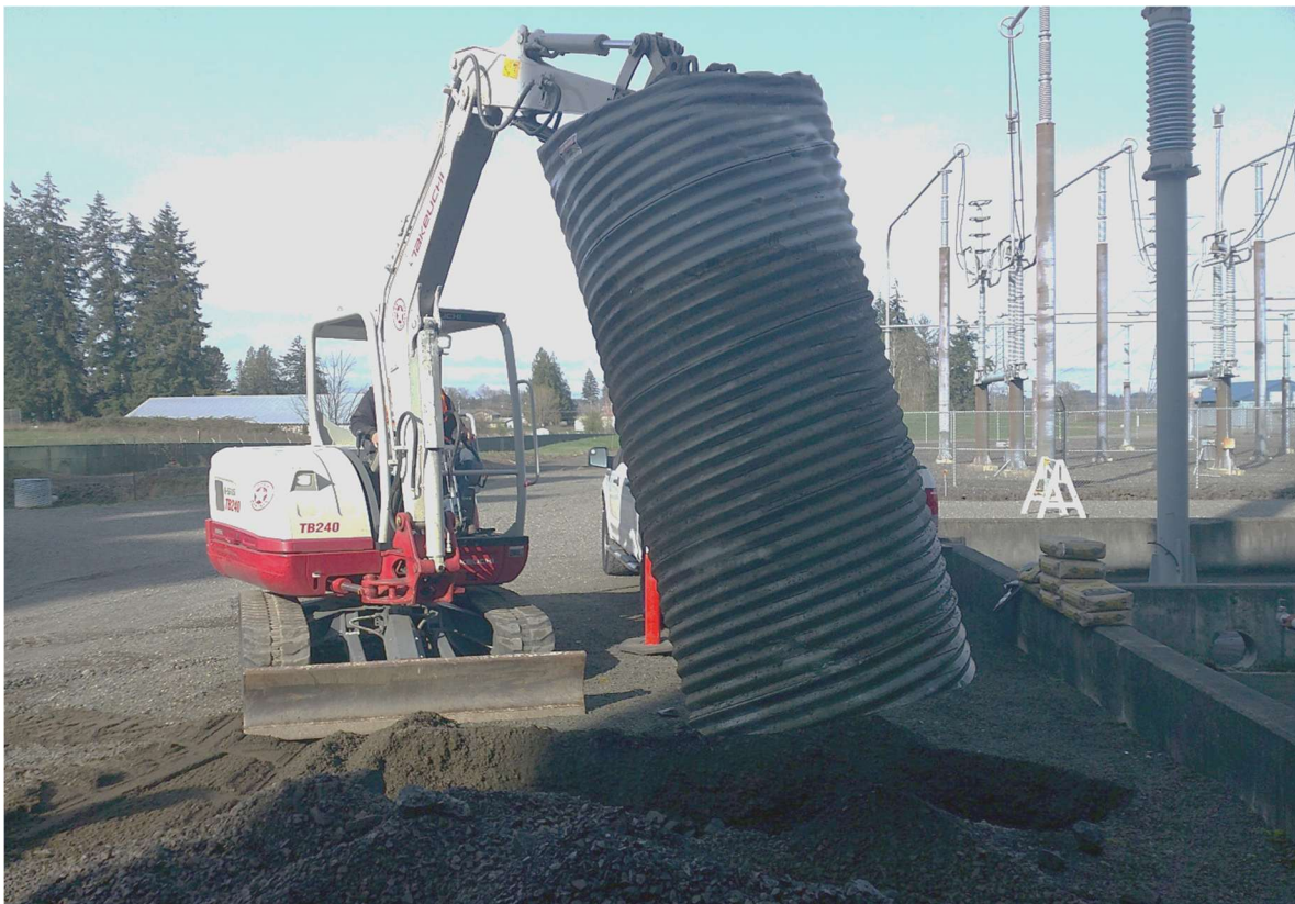
Well casing removed from subsurface.
