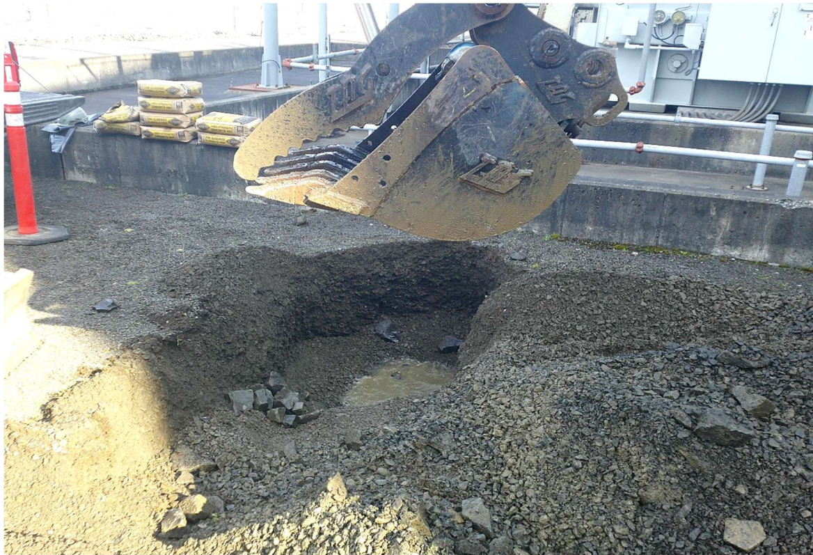
Backfilling culvert location and excavation with fill.
