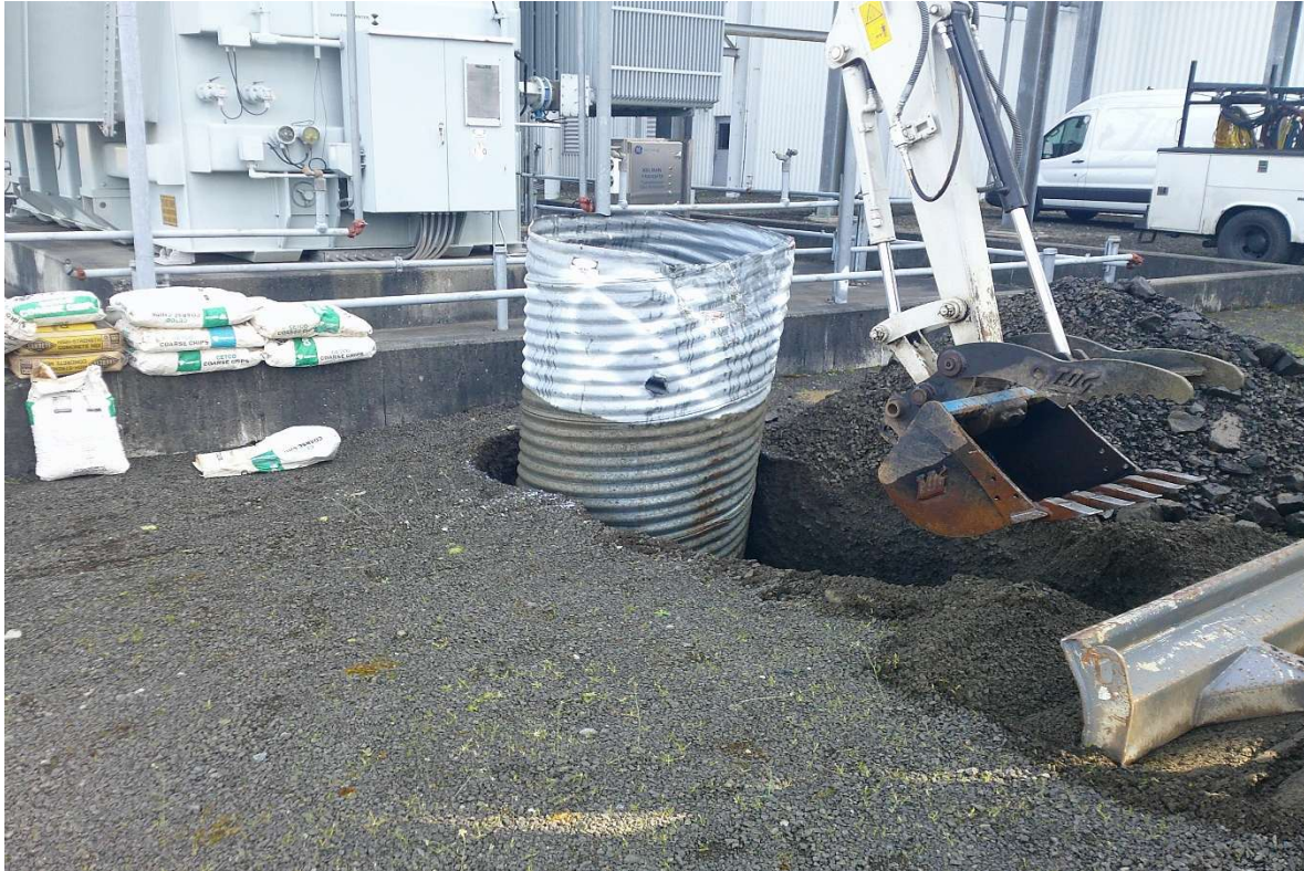
Casing prior to adding bentonite and concrete ready-mix.
