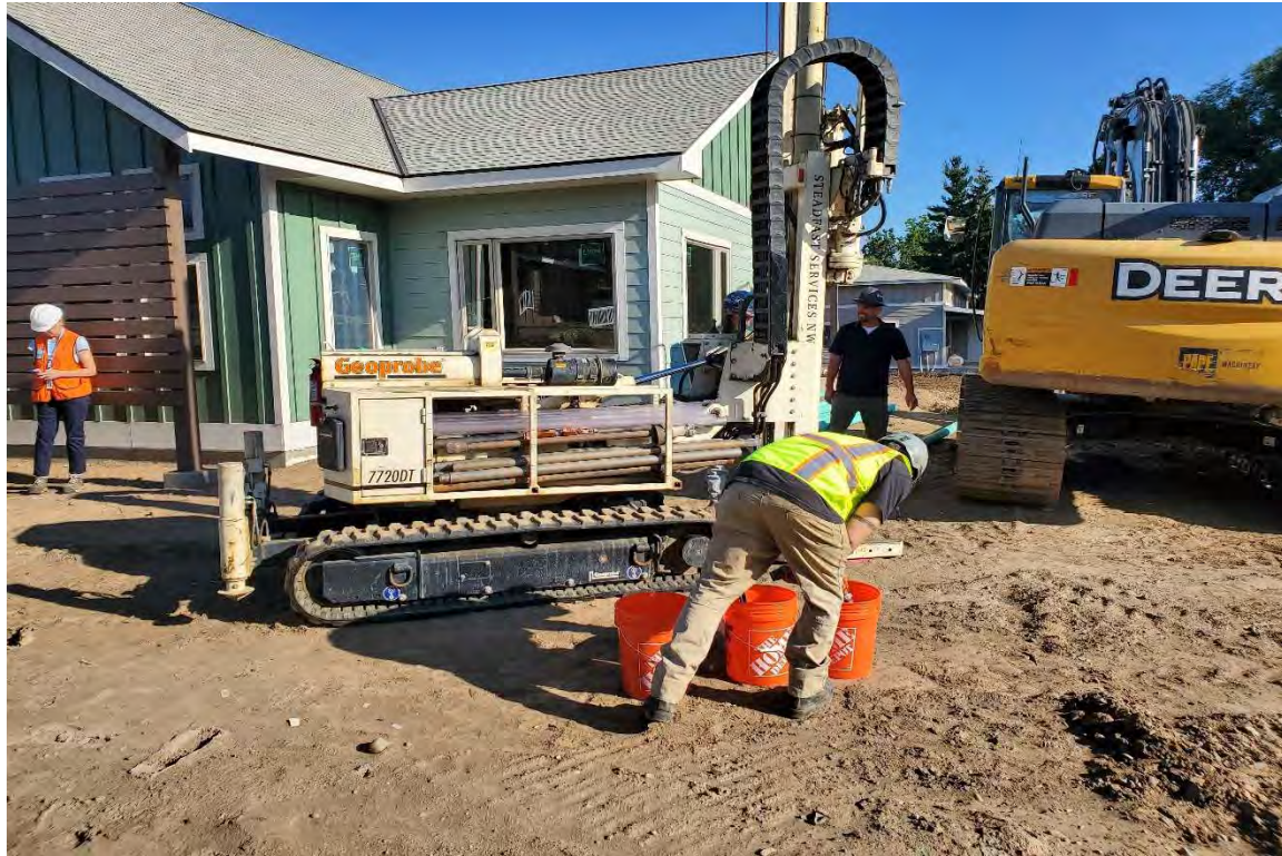
DRILLING BOREHOLE B1
