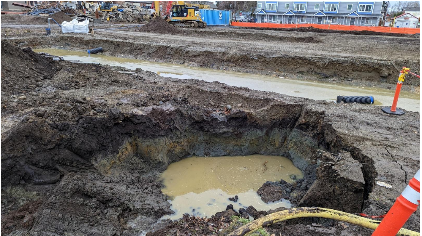
Photograph 3. Southern extent of excavation at a depth of 7 feet below ground surface (bgs), filled with groundwater at a depth of 5 feet bgs. No sheen observed.
