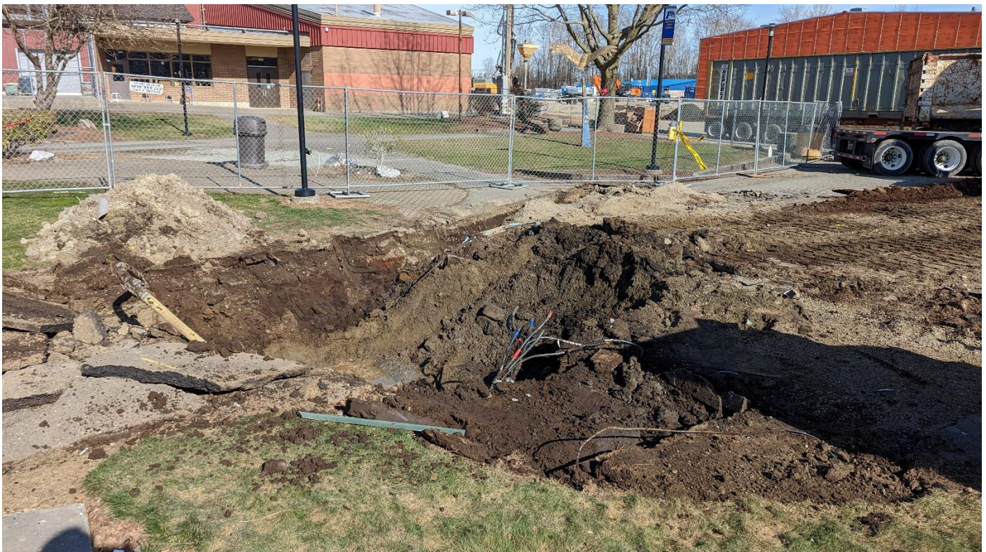
Photograph 2. Conduit extruding from the surface soil layer at the former location of the transformer.
