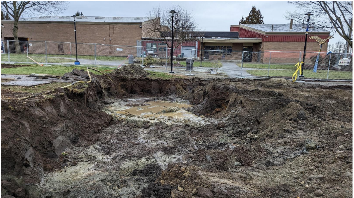
Photograph 4. Extent of the majority of the excavation at a depth of 4 feet bgs.
