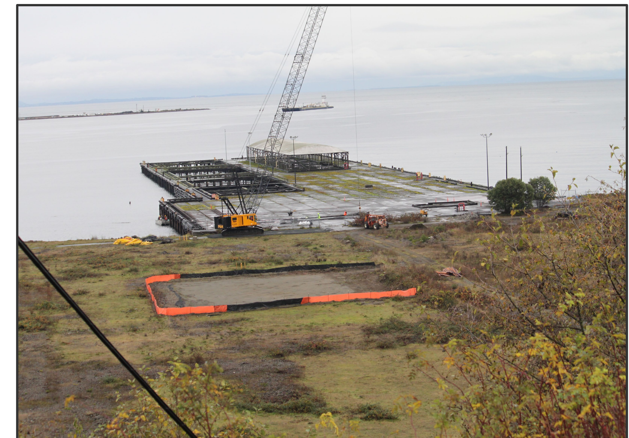
Removal of dock concrete panels, 2020
