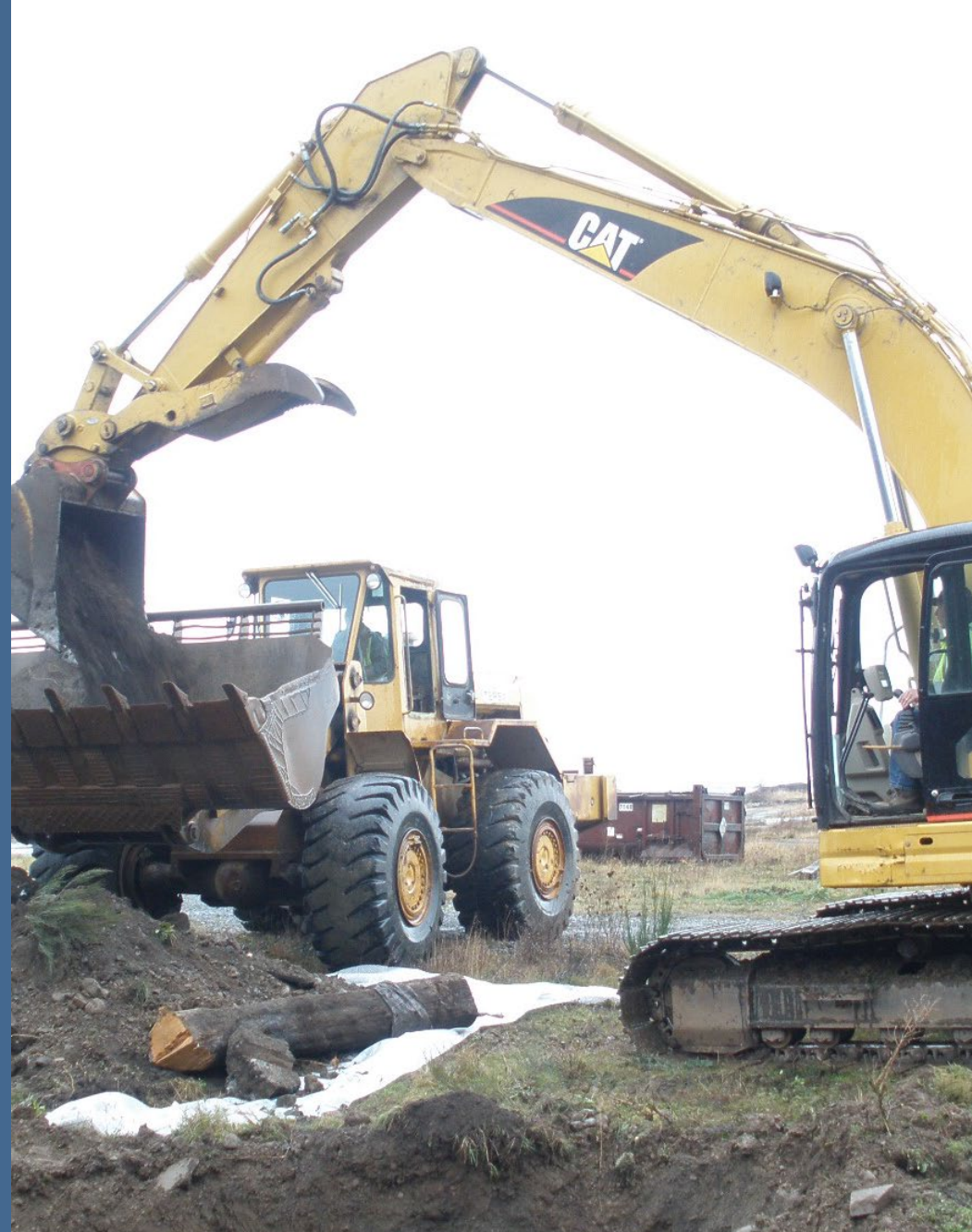
Test Pitting at Rayonier Mill
