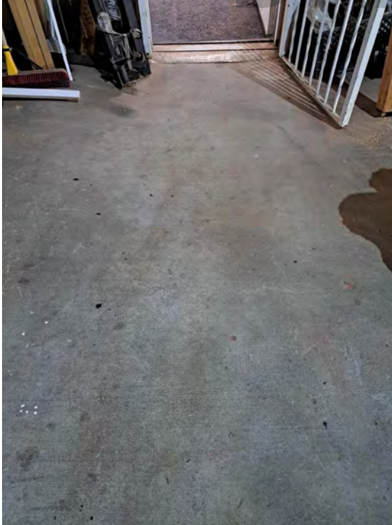
Photo 1: From Garage Looking East
