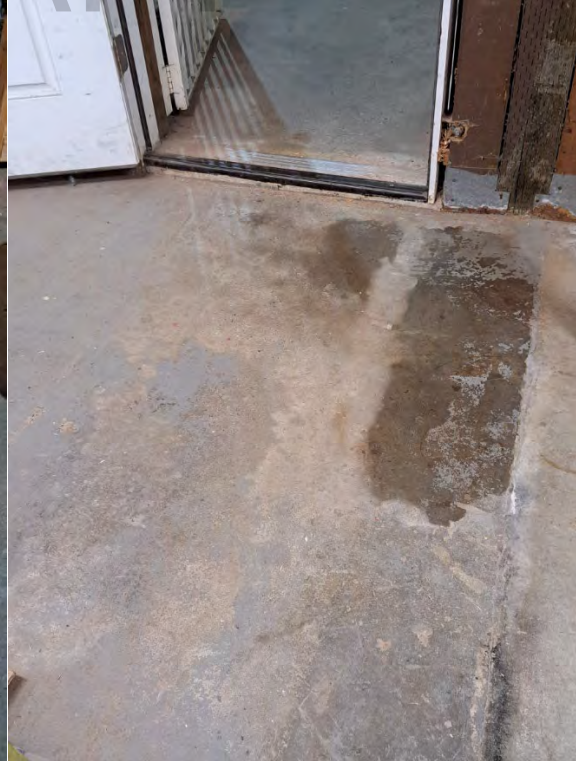
Photo 2: From Storage Area Looking West
