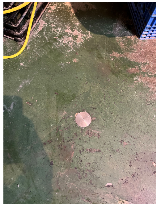
Photograph No. 08: Zoomed view of a vapor pin completed with flush, stainless steel covering following sample collection.
