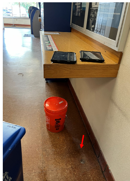
Photograph No. 04: View of newly installed vapor pin, VP-4, located inside of the U.S. Post Office building
