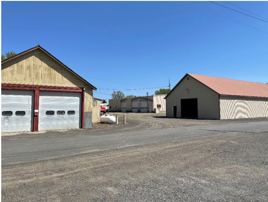
Photo 4: View northeast of Lincoln County maintenance yard and buildings
