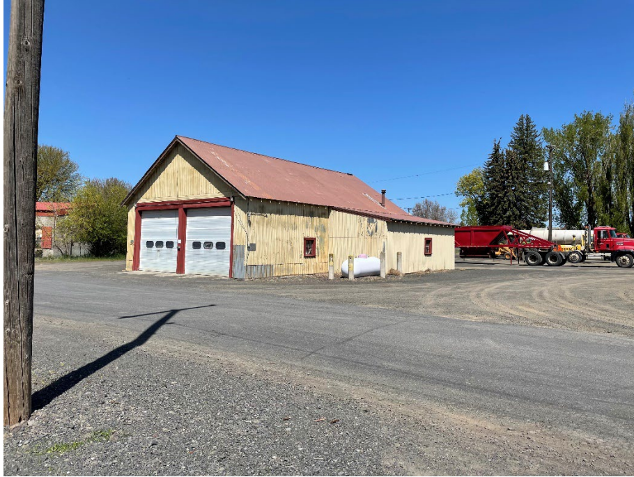
Photo 1: View northwest of former WSDOT property
