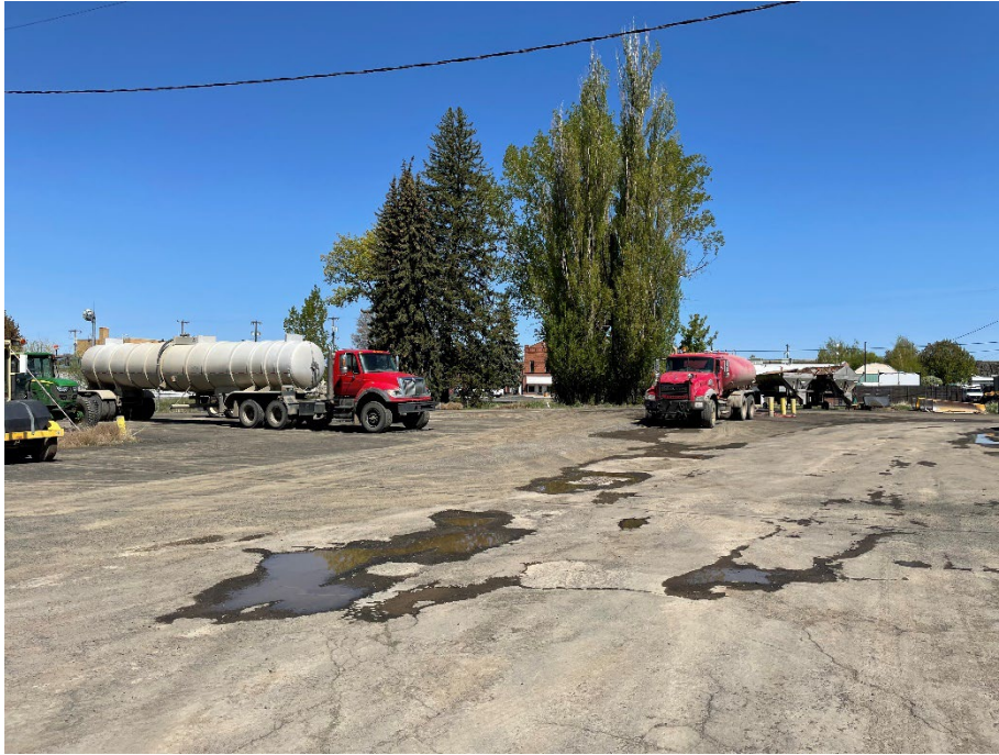
Photo 3: View north of paved portion of Lincoln County maintenance yard
